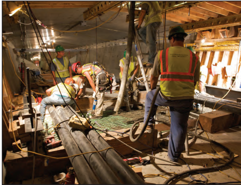
Workers Inside the northbound box girder during the concrete pour for the closure of the center span over the river on July 22, 2008.
