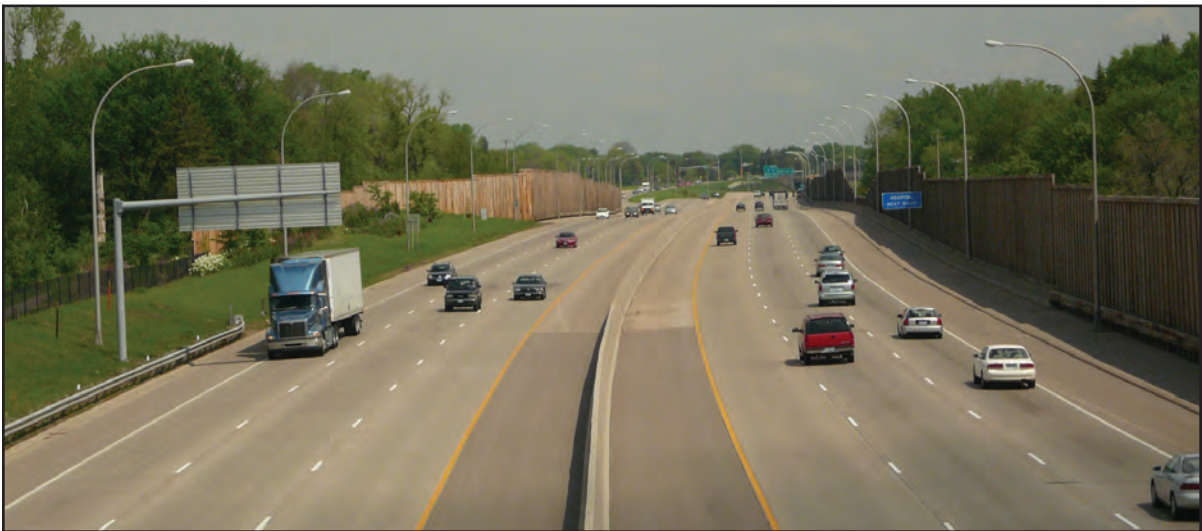
Typical lighting on urban freeways: “Cobra head” lamps on 49-foot poles. There are literally thousands of such poles on Minnesota highways. These are on Highway 100 in New Hope. Before the highway was reconstructed in 2003, light poles were mounted atop a median barrier.
