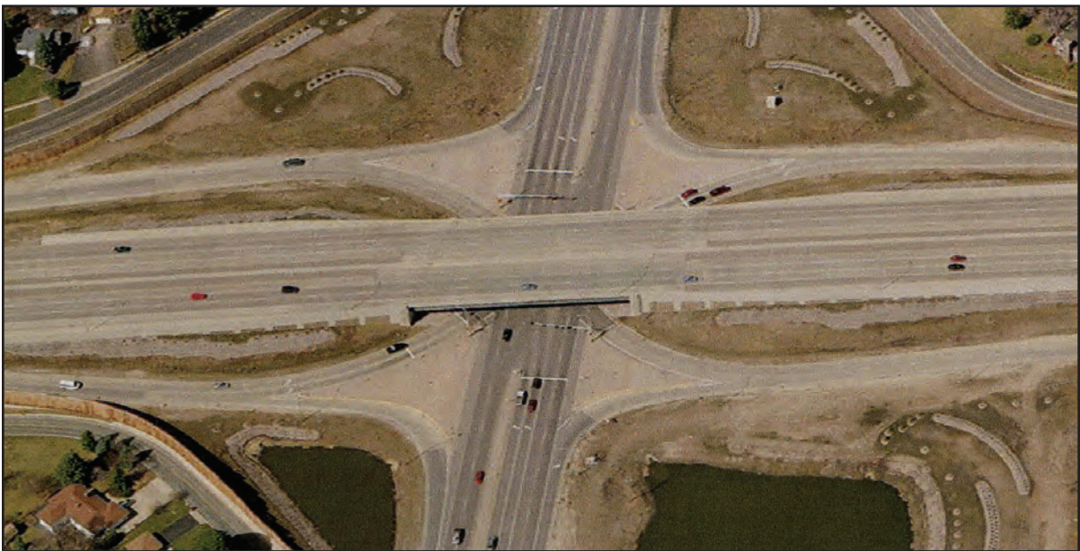
This single-point diamond interchange on Highway 100 at Olson Highway (Highway 55) replaced the cloverleaf built in 1940. There is only one signalized intersection in this type of interchange compared to the two signalized intersections needed at most busy standard diamond interchanges.
