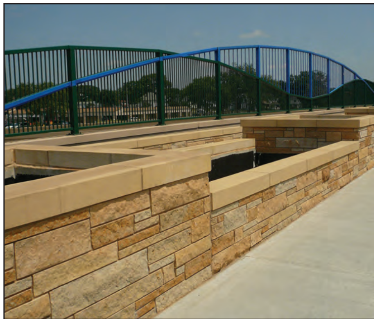
Detail of the railings and planter boxes on the north sidewalk of the Second Street Southwest bridge. Plantings were yet to be installed at the time the photo was taken.
