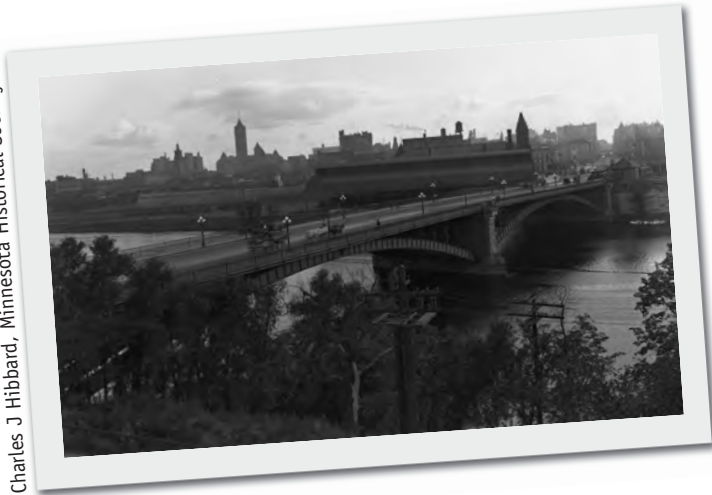
The third Hennepin Avenue Bridge, a two-span, steel-arch structure, as photographed from Nicollet Island in 1911. Steel had just begun to replace iron as a preferred bridge building material by the time the bridge was under construction in 1889. The deck was 56 feet wide between curbs with a 12-foot sidewalk on each side.
