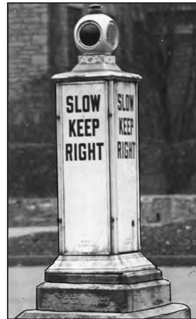
This "KEEP RIGHT" installation was located somewhere in St. Paul, ca. 1930. Today, it would clearly violate the implied rule that any device installed on the road should do less harm (if anything were to collide with it) than whatever it is warning drivers about or protecting them from. Note that "SLOW" signs are not provided for in today's MUTCD.
