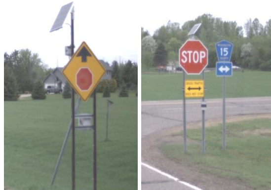
Sign-Mounted Detector and LED STOP Sign
