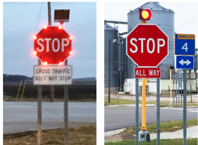
Figure 6. Edge-Lit LED STOP Sign and STOP Sign with Red Beacon
