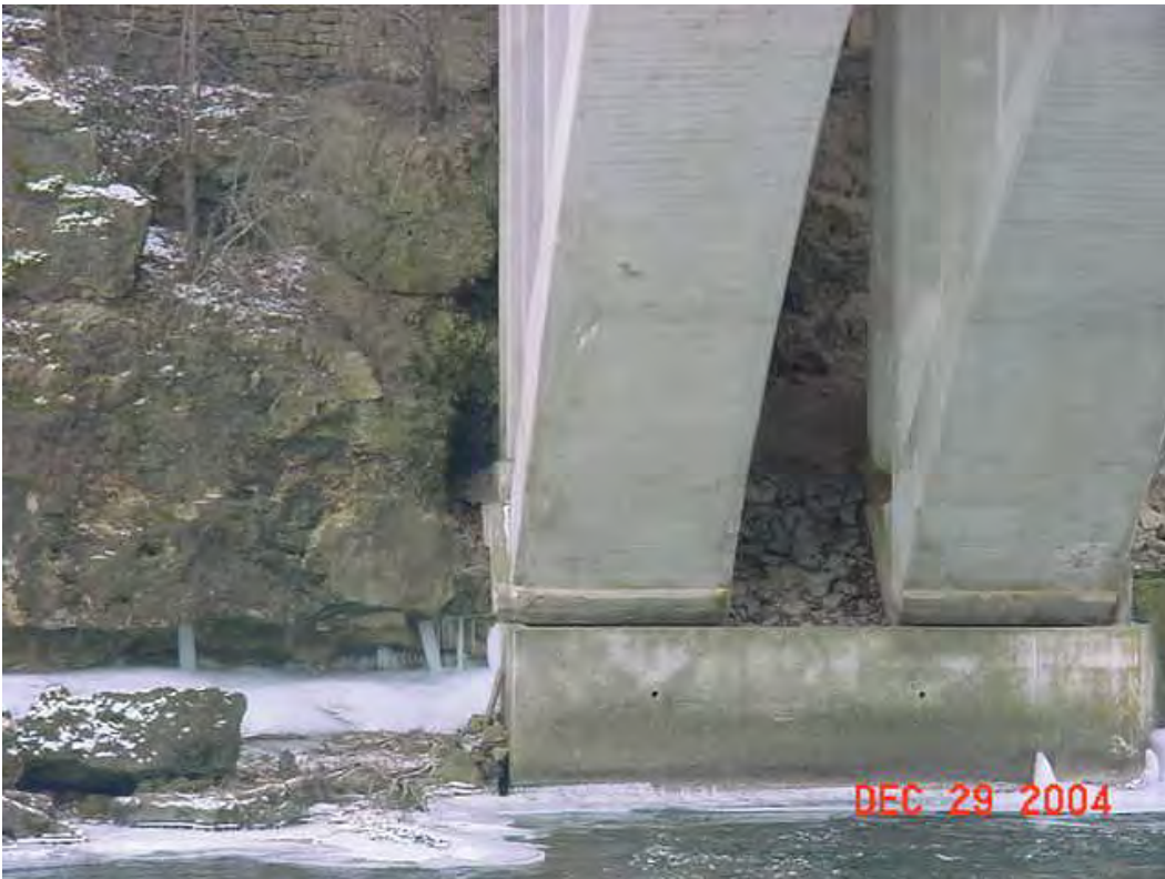
South Abutment footing
