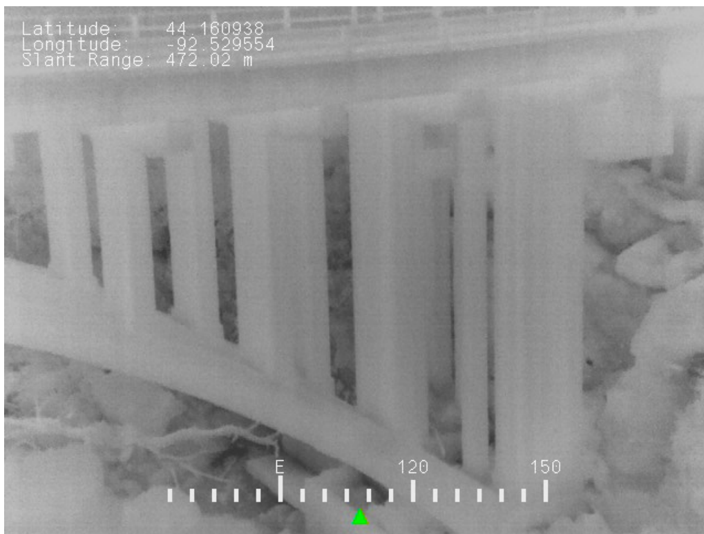
Figure 5-9 Bridge 448 IR View of Arch.
