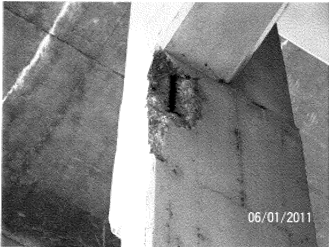
Photo 2 - East Arch Column 2 South End
