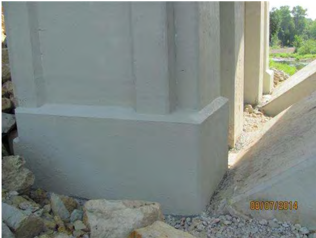
Photo 12 - Repaired Northwest side of Arch ftg.
