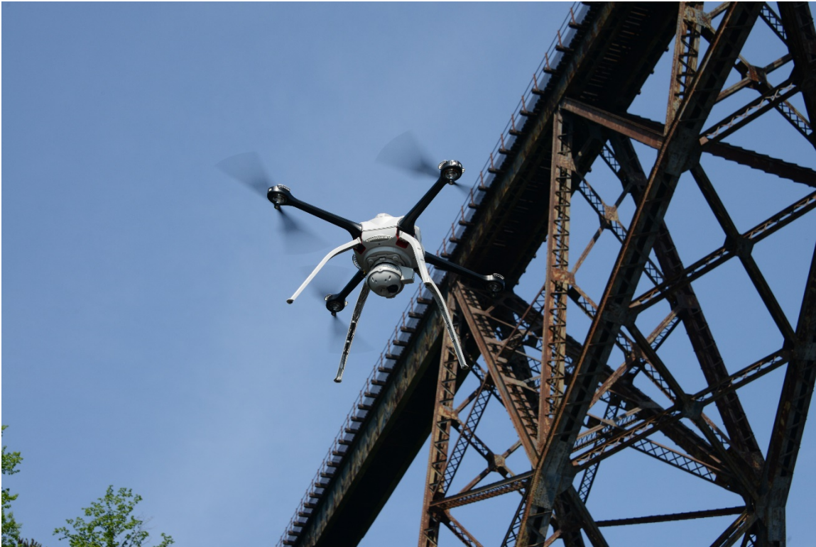
Figure 4-1 Photograph of the Aeyron Skyranger UAV Next to Bridge.
