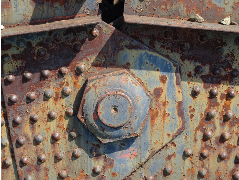
Figure 5-21 Close up Photograph of Arcola Bridge Pin Detail Photo 4.
