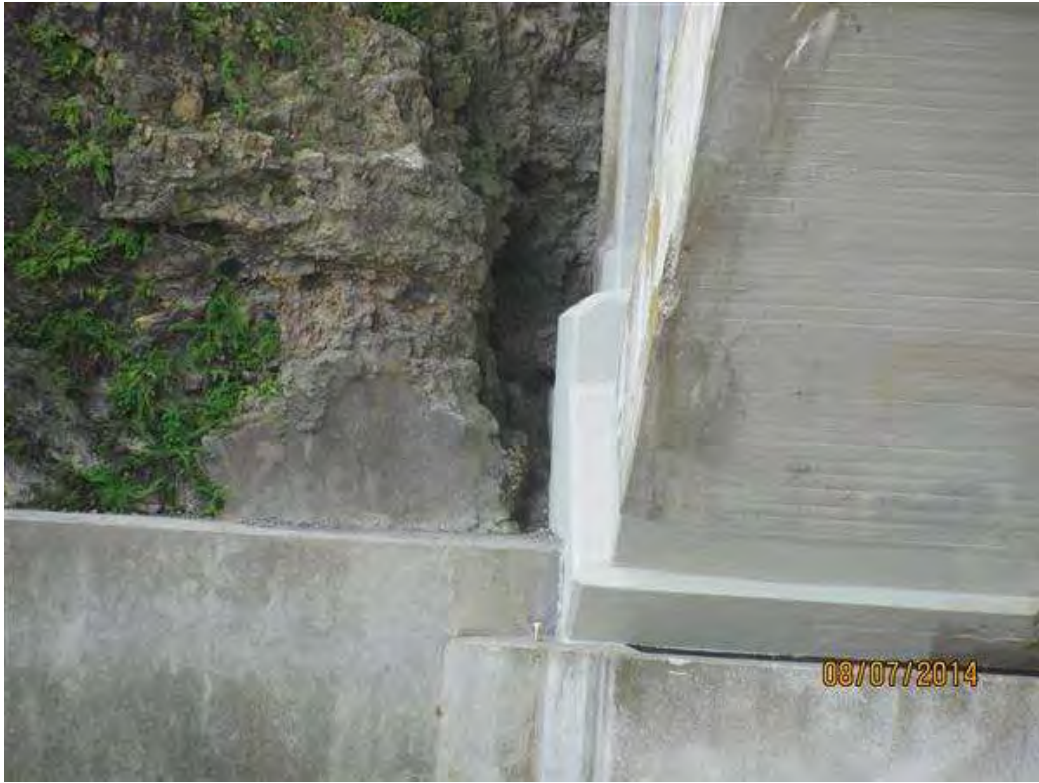
Photo 15 - SE corner of the arch repaired
