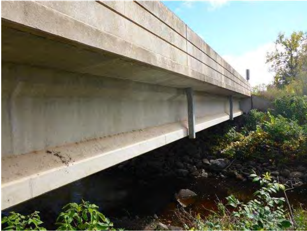
Photo 5 - West Fascia Looking South
