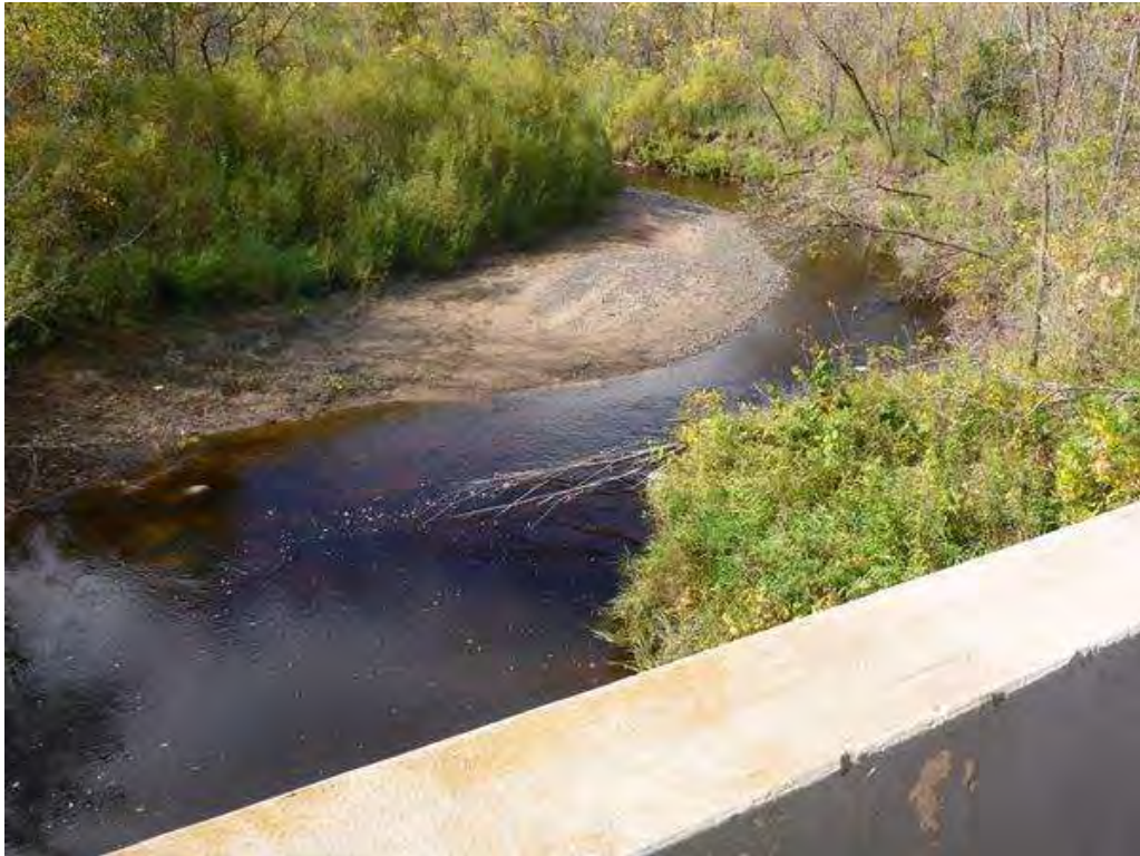
Photo 2 - Upstream Channel Looking West
