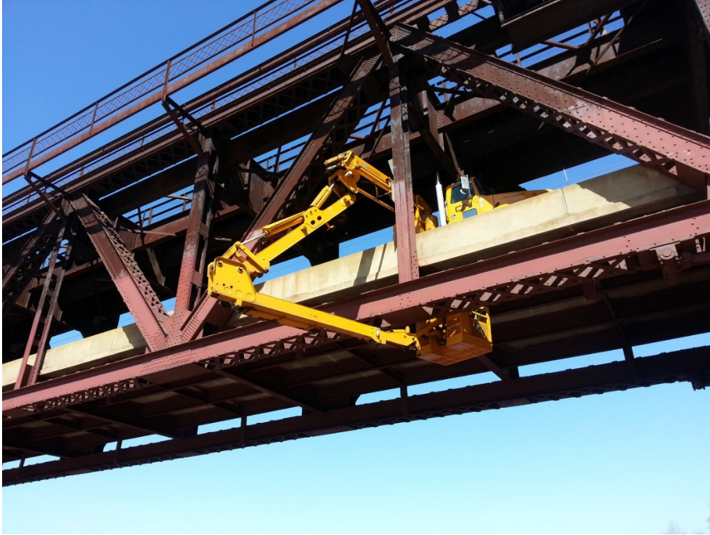
Figure 3-1 Example of a Under Bridge Inspection Vehicle.
