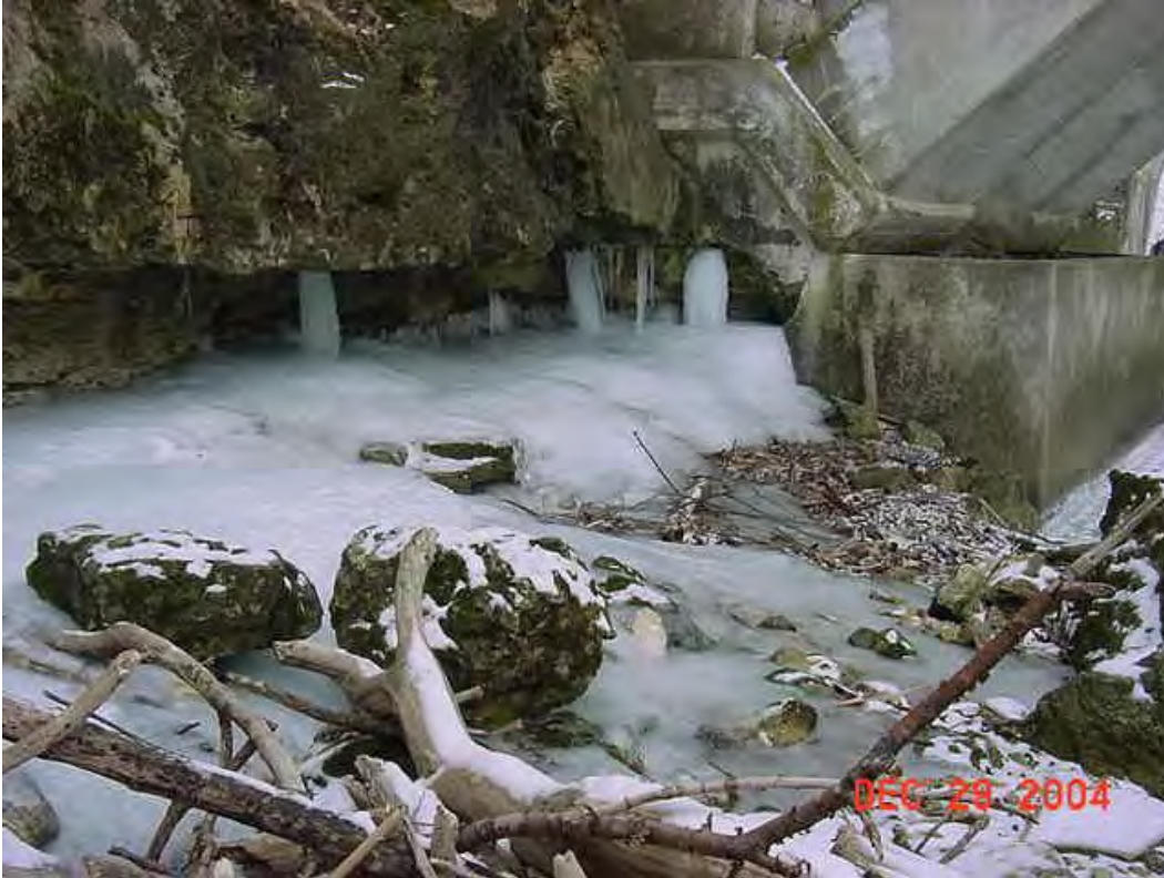
South Abutment footing
