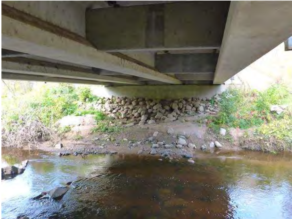
Photo 6 - Underside of Bridge Looking North
