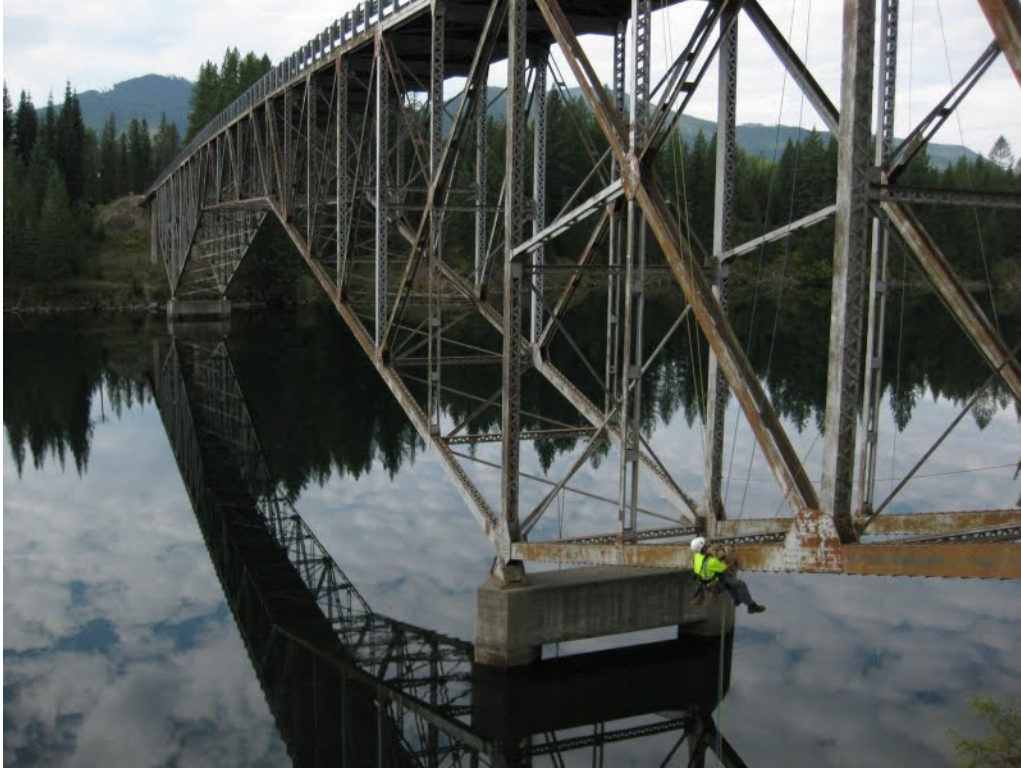
Figure 3-2 Example of a Rope Access Inspection.
