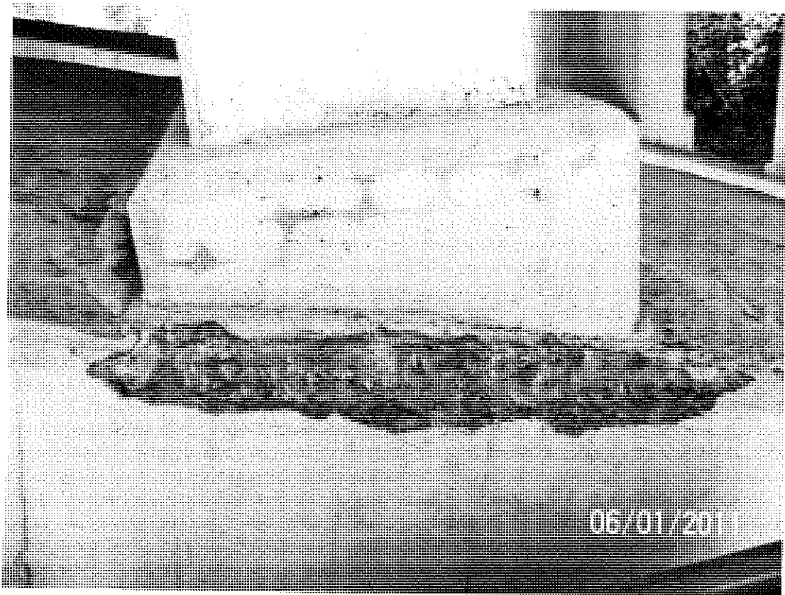
Photo 24 - West Arch West Face Spandrel Column 5
