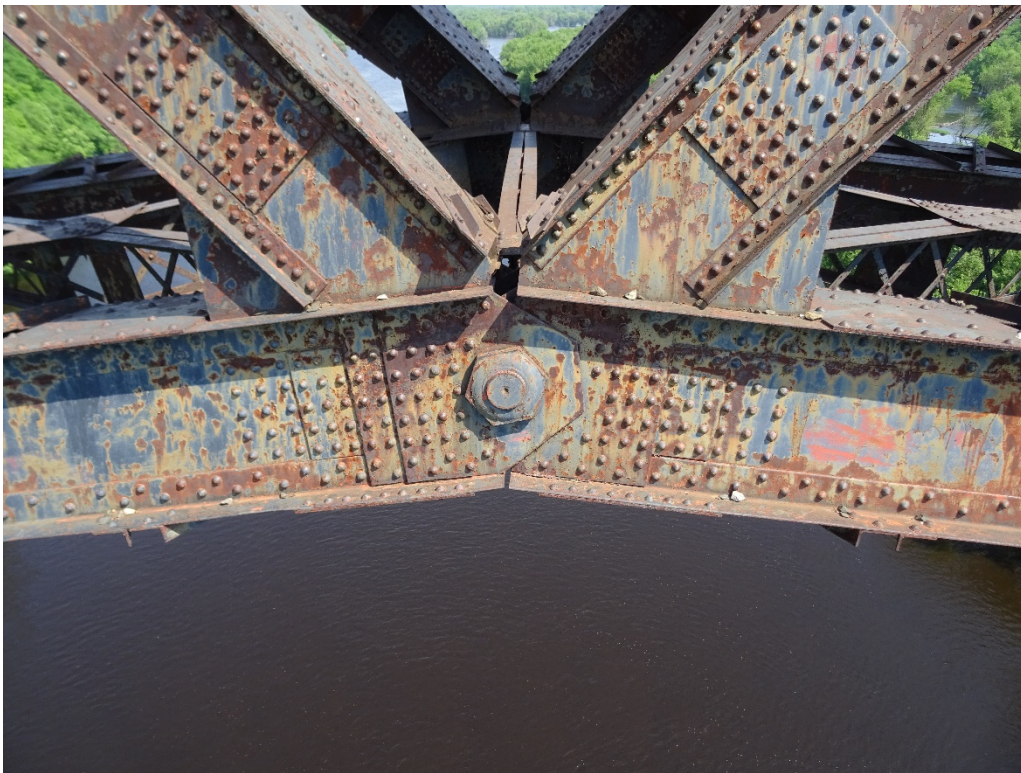
Figure 5-20 Photograph of Arcola Bridge Pin Detail Photo 3.
