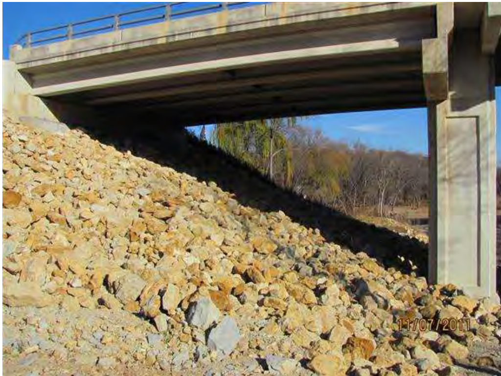
Photo 2 - New Rip rap at North abutment.
