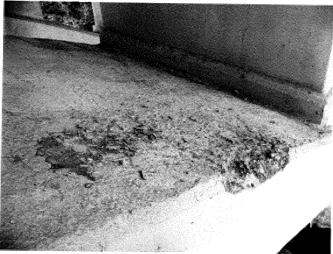
Photo 23 - West Arch West Face North of Spandrel Column 3
