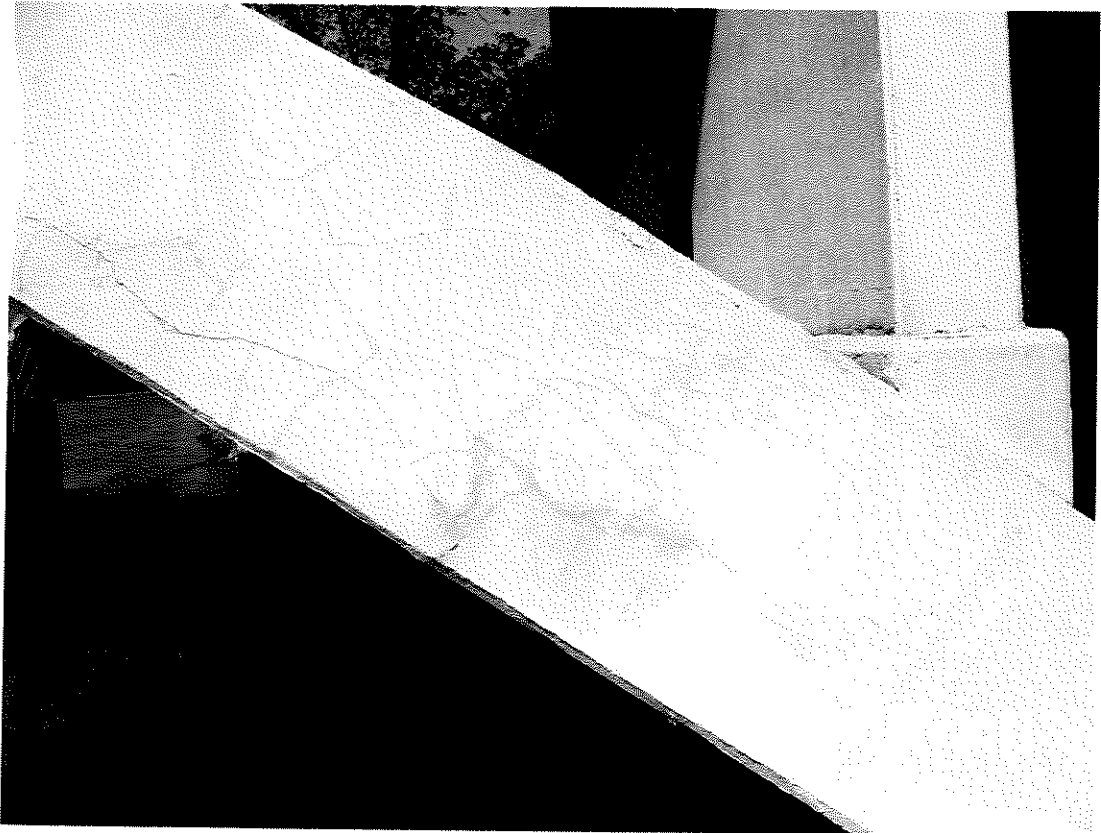
Photo 17 - East Arch Between Spandrel Columns 15 & 16
