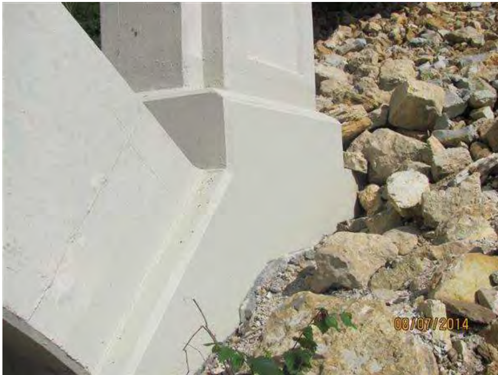
Photo 14 - Repaired Northeast side of the arch.
