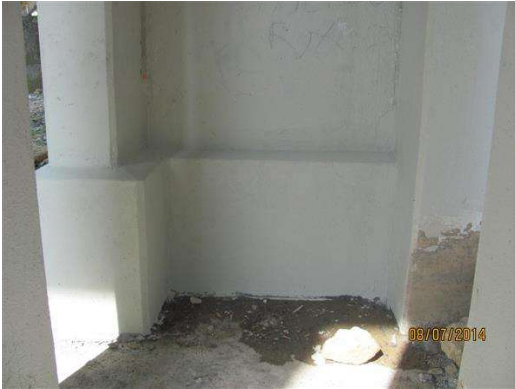
Photo 17 - Column repairs at north base of arch.
