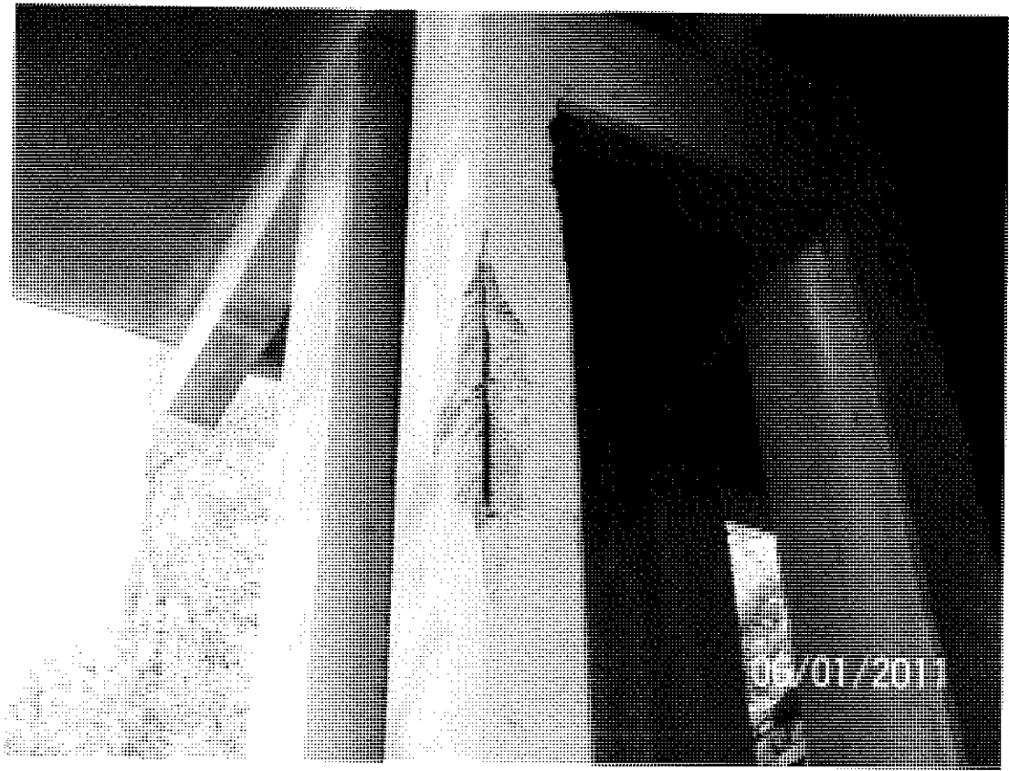
Photo 3 - East Arch Column 2 South End
