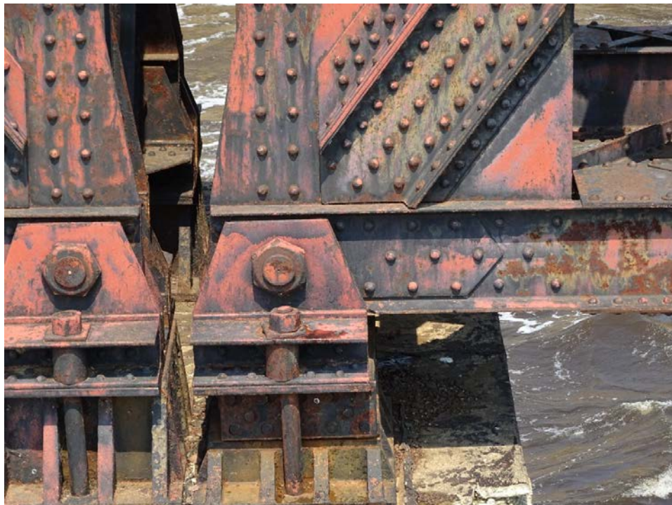
Figure 5-13 Photograph of Bridge 49553 Top Chord.
