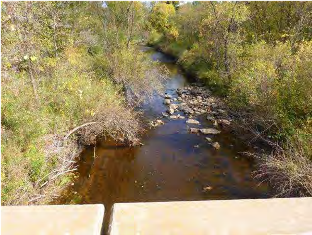
Photo 3 - Downstream Channel Looking East
