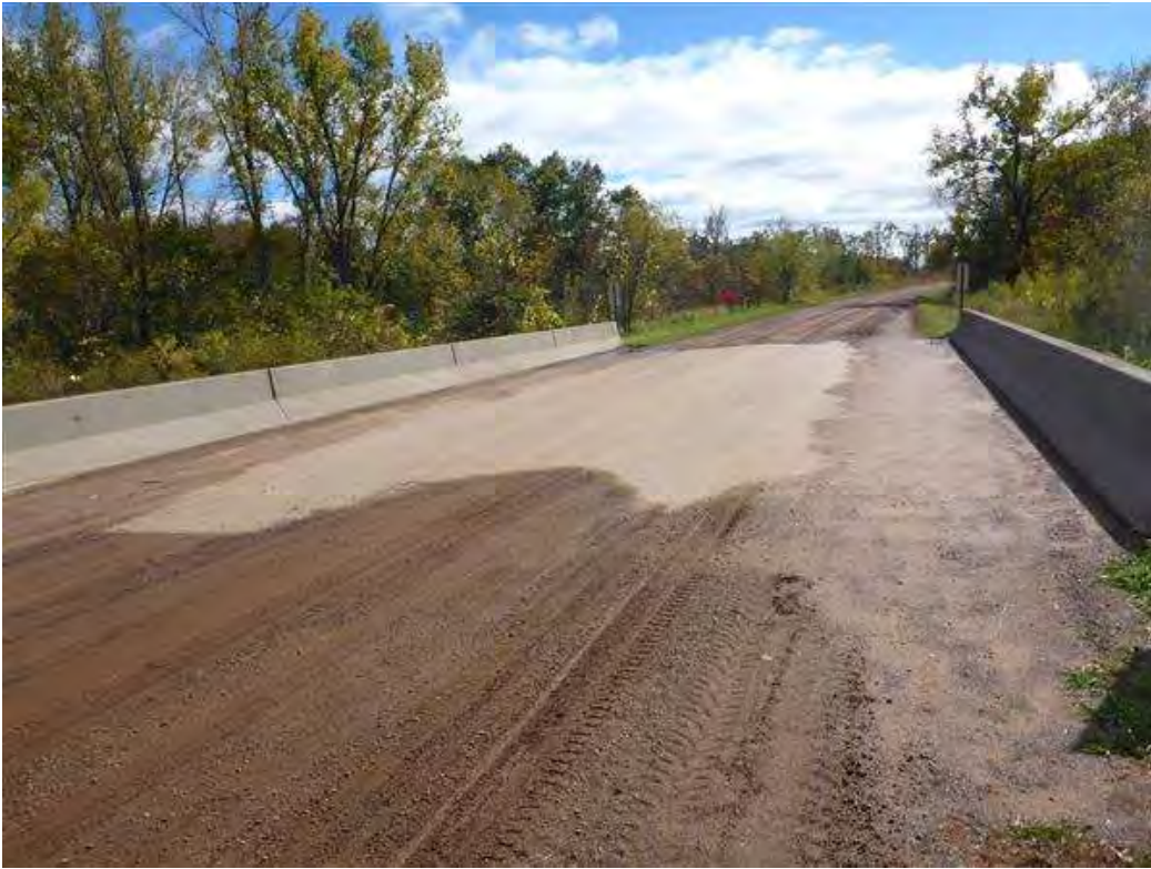
Photo 1 - Top of Deck Looking South
