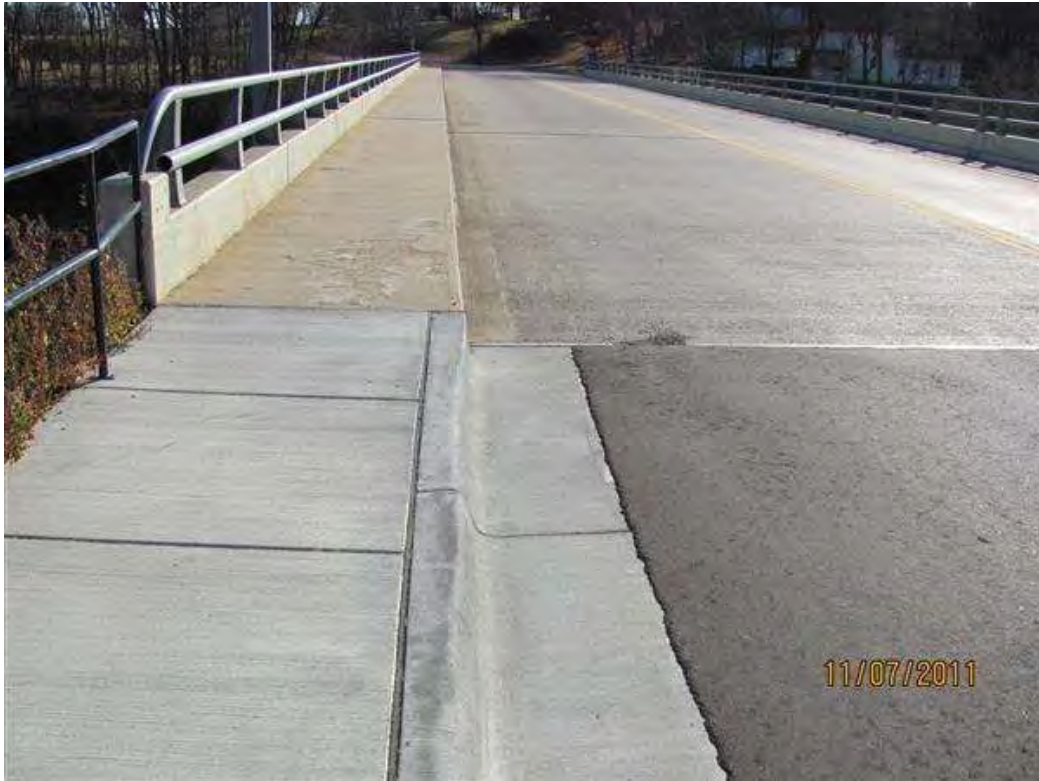
Photo 1 - New sidewalk and curbs at North abutment.
