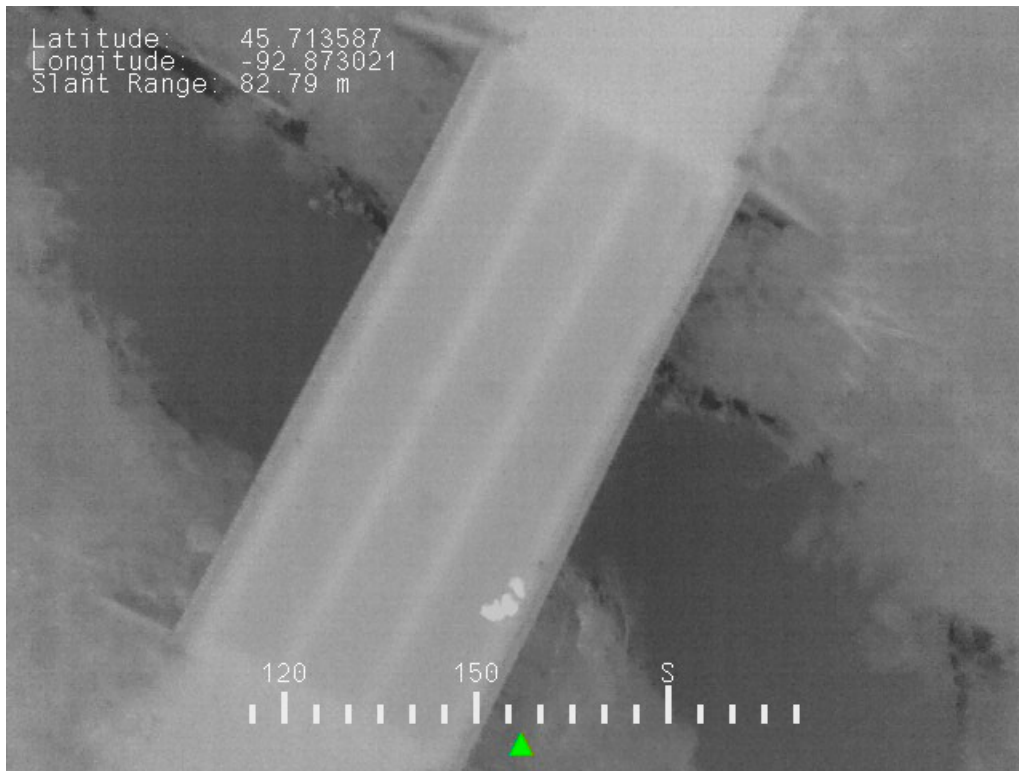
Figure 5-3 Bridge 13509 IR Image of Bridge Deck.
