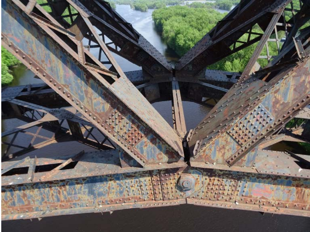
Figure 5-19 Photograph of Arcola Bridge Pin Detail Photo 2.
