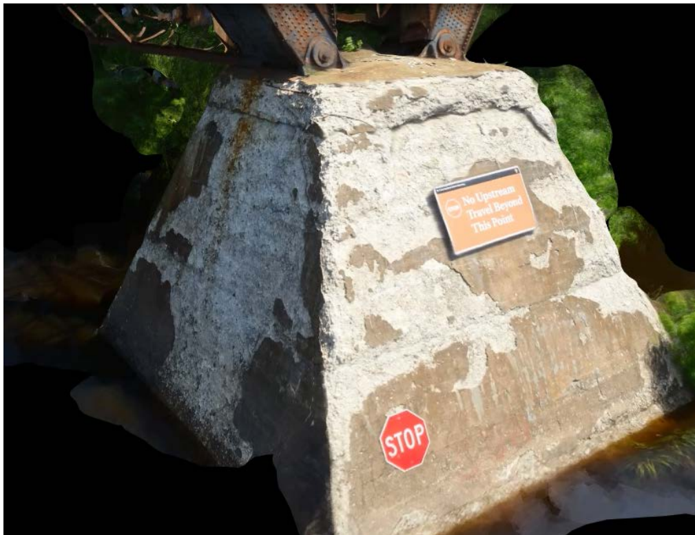
Figure 5-23 3D Orthographic Model of Bridge Foundation.
