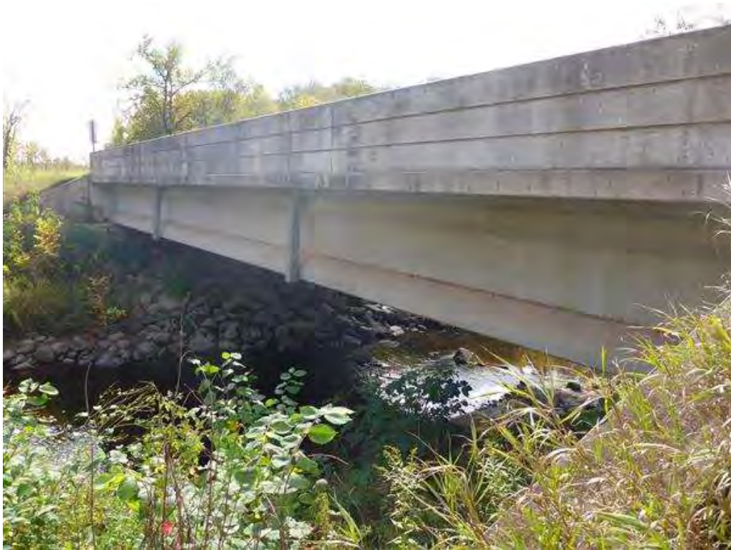
Photo 4 - East Fascia Looking Southwest
