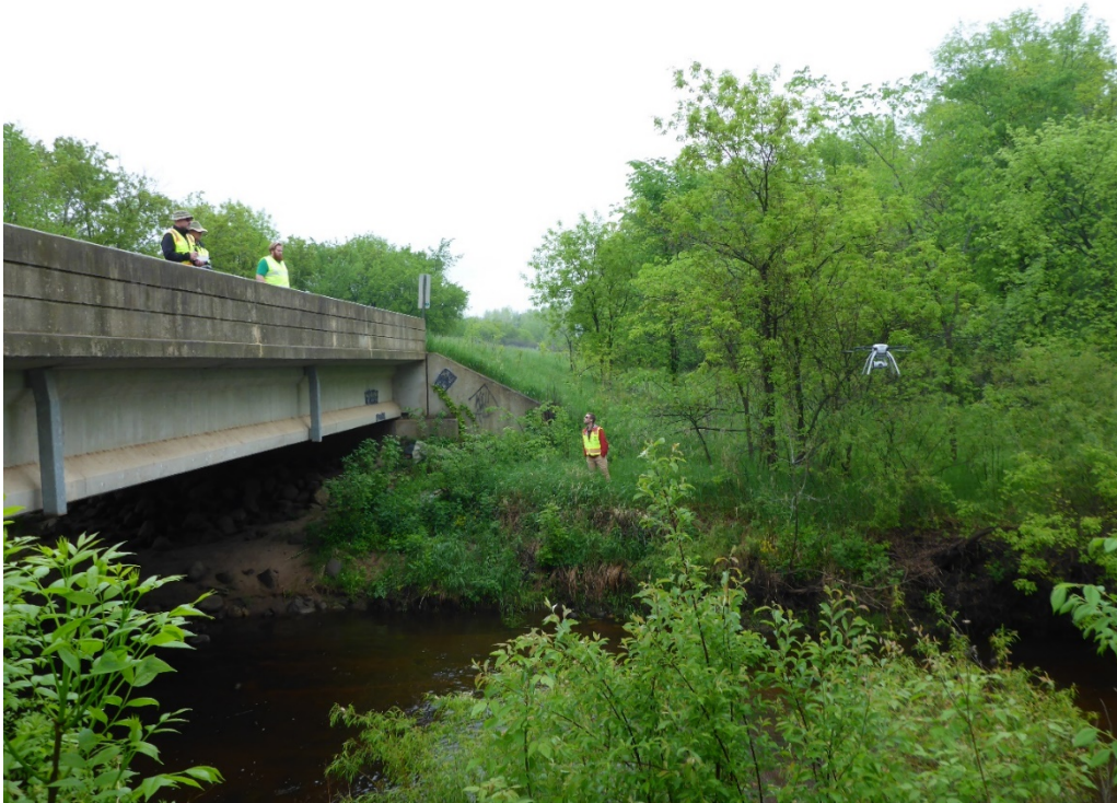
Figure 5-2 Bridge 13509 Overall View of Inspection.
