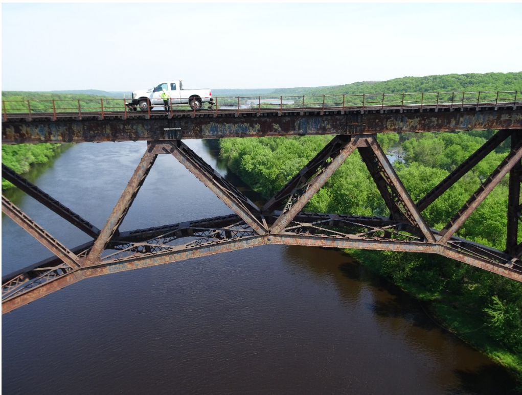
Figure 5-18 Photograph of Arcola Bridge Pin Detail Photo 1.
