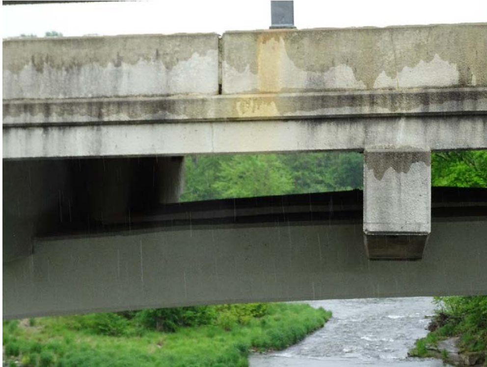
Figure 5-8 Photograph of Bridge 448 Detail Near Top of Arch.
