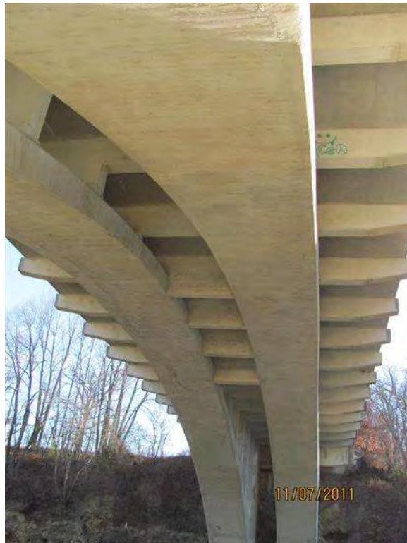
Photo 4 - Under side of archs
