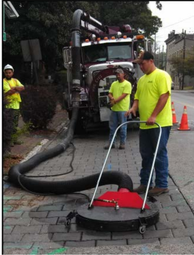
Figure 2.6. Maintenance of permeable-articulated concrete block/mats with a Vac Head (Photo courtesy of University of Louisville and D. Buch, PaveDrain LLC.).
