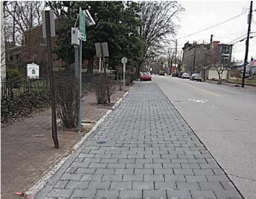
Figure 2.5. Permeable articulated concrete block/mat A) installation and, B) completed project (Photos courtesy of University of Louisville and D. Buch, Pavedrain, LLC.).
