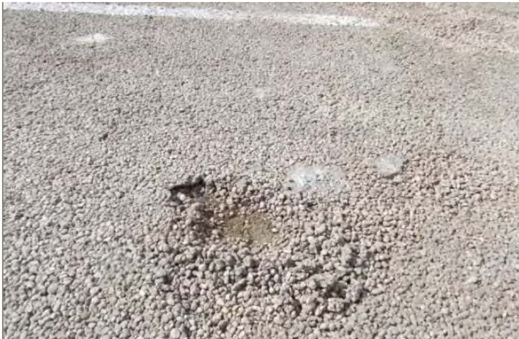
Figure 9.23. Pervious concrete parking lot at National Renewable Energy Lab in 2011. a) Deteriorated surface with loose aggregate, b) Close-up of parking stall (photos courtesy of K. MacKenzie, UDFCD).
