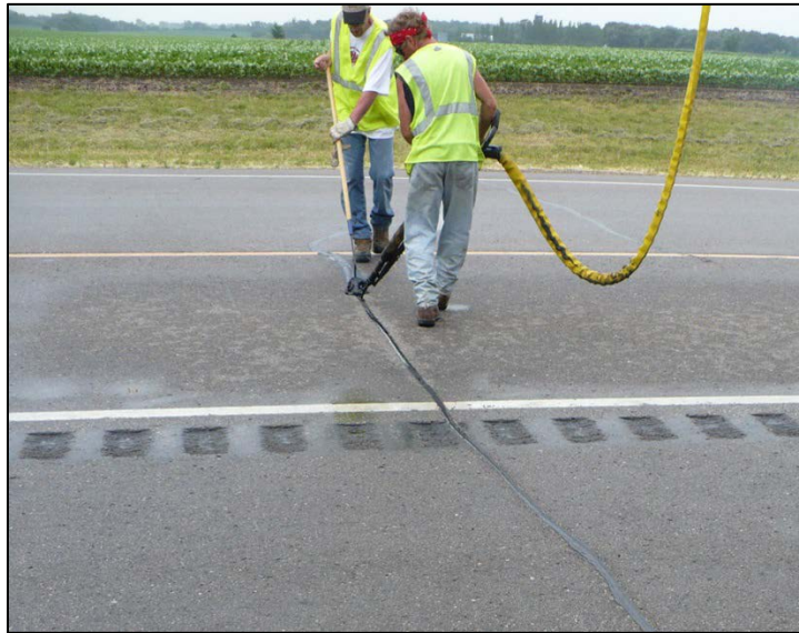
Figure 21. Crack Sealing.
