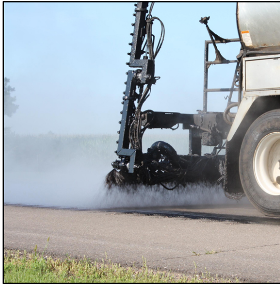
Figure 25. Chip seal emulsion application.
