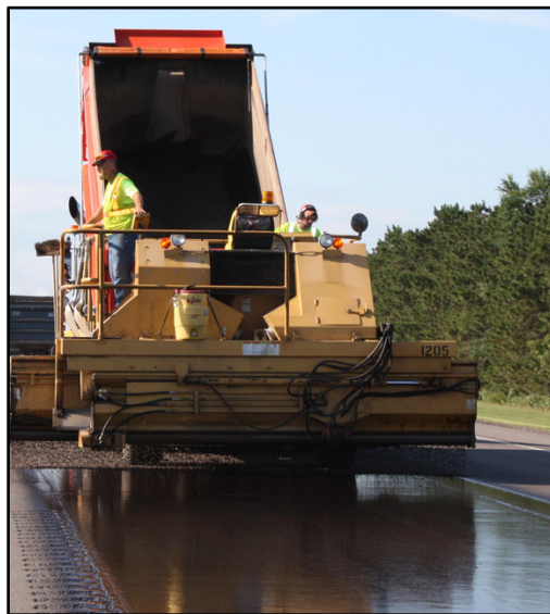
Figure 26. Chip seal application.
