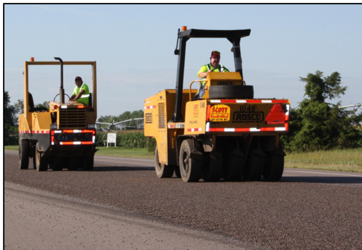
Figure 28. Chip seal rolling operation.
