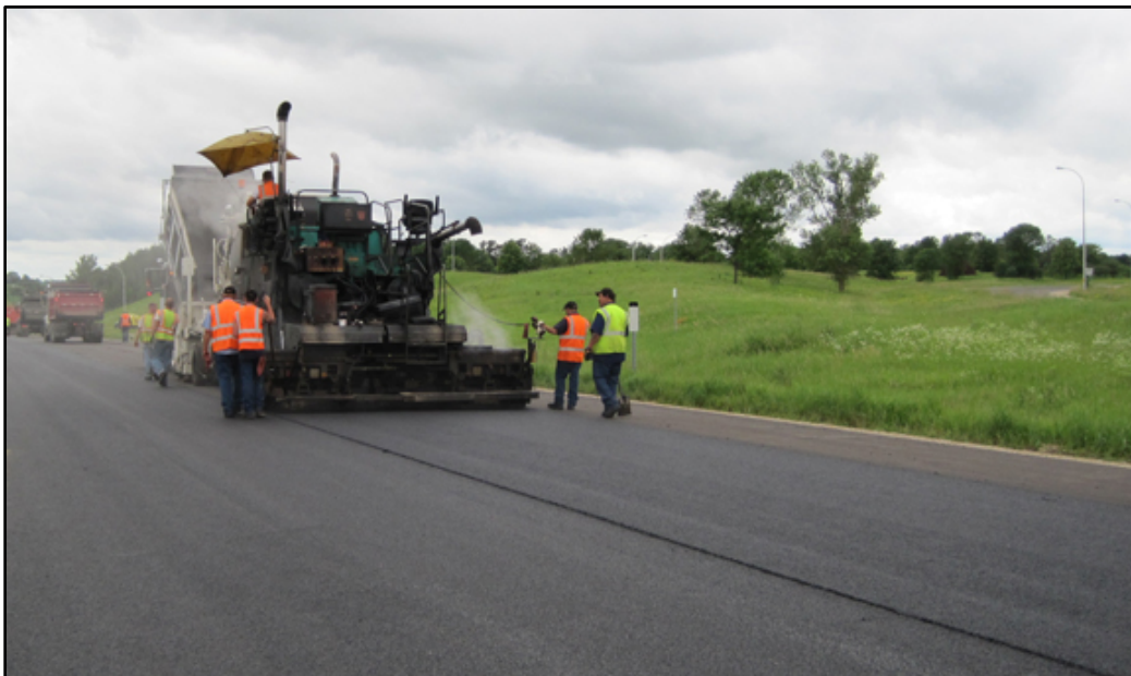
Figure 30. Thin bonded wearing course application.
