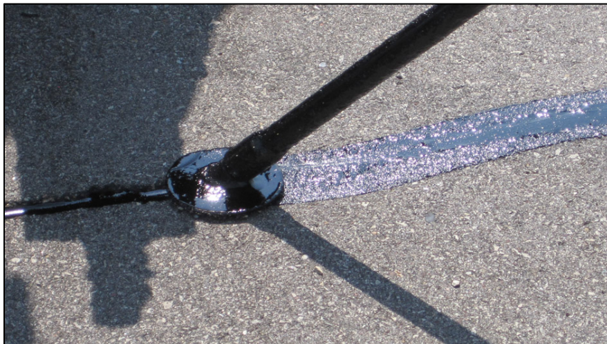
Figure 22. Crack Sealing.
