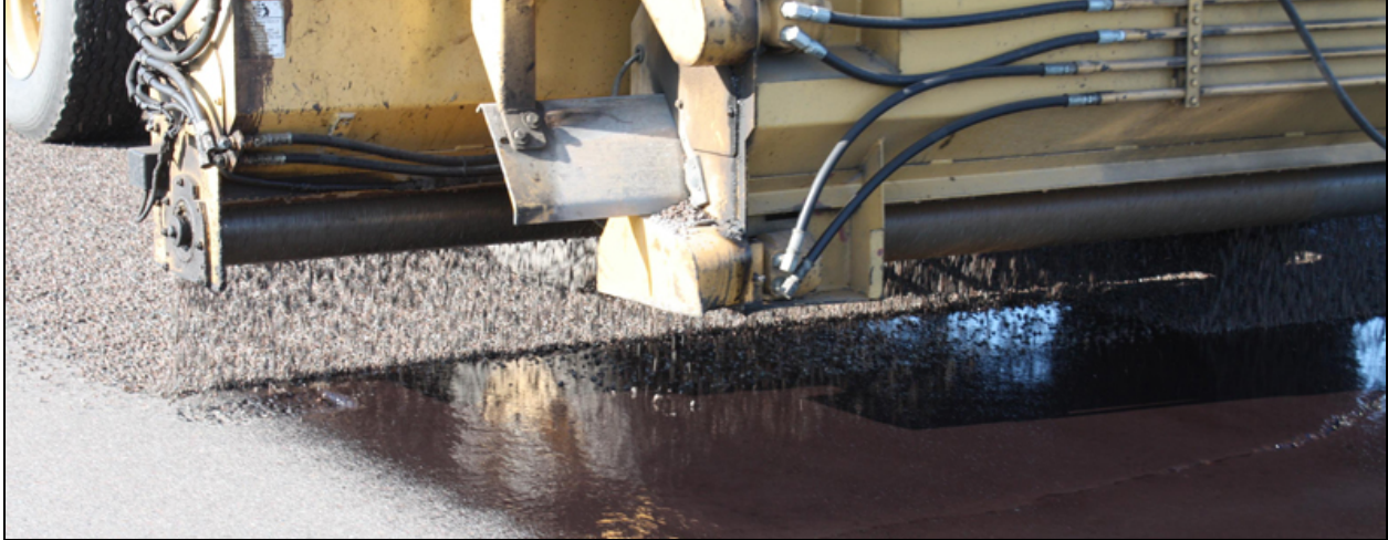
Figure 27. Chip seal application.
