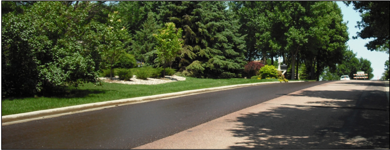
Figure 29. Micro surfacing.
