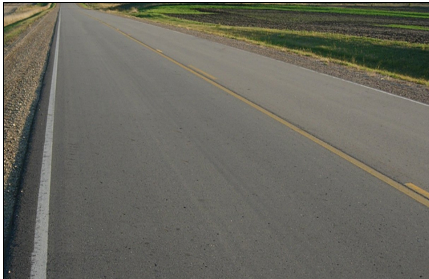
Figure 12. Newly-paved flexible pavement.
