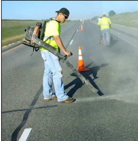
Figure 23. Cleaning cracks prior to sealing.
