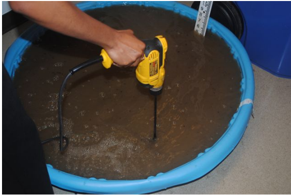
c) Mixing by drill-mounted vertically-oriented turbine to 6-inch deep water in tank made from kiddie pool.
