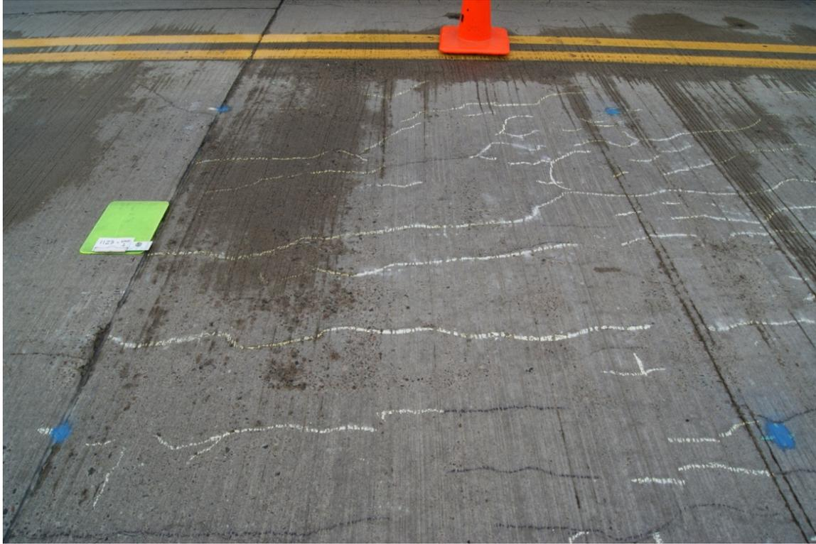
Figure A.3: Photograph of 6 ft. x 6 ft. square area on bridge surface indicated by four blue painted dots with crack locations marked in chalk
