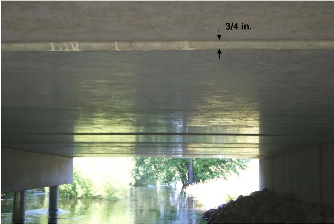
**Figure 3.19: Observed differential camber of the inverted-tee beams from Bridge No. 33008**
