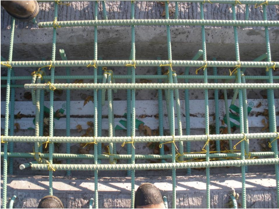
**Figure 5.4: Construction photograph showing the placement of a mastic bond breaker on Bridge No. 08006**
