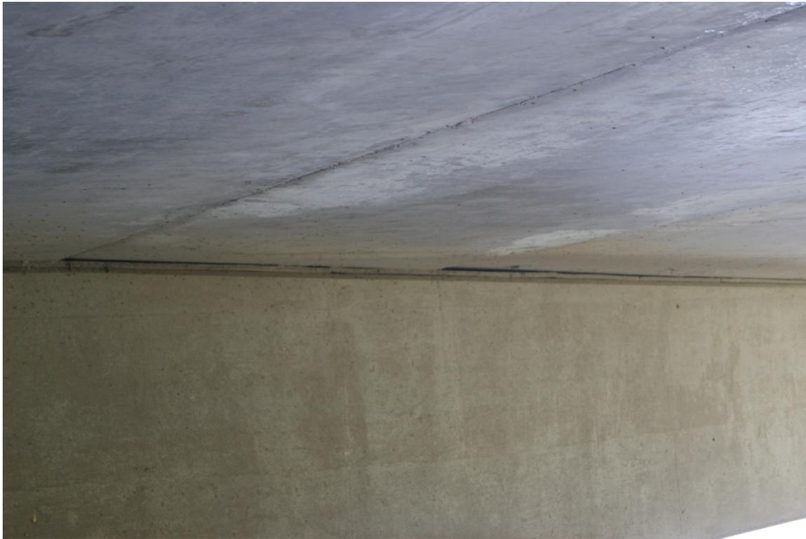
**Figure 3.18: Uneven bearings of end-span precast beams at the north pier of Bridge No. 33005**
