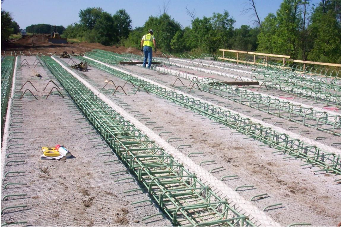
**Figure 1.3: Photograph of Bridge No. 49036 during construction showing the drop-in cage reinforcement prior to placement of deck reinforcement and CIP concrete (MnDOT 2009)**
