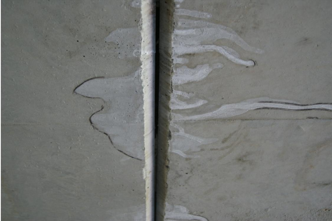
**Figure 3.9: Efflorescence at a longitudinal joint underneath Bridge No. 49007**
