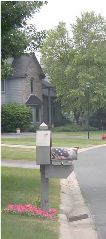
A Typical Community Mailbox at Risk of Being Struck by Winter Maintenance Equipment (too low and forward of back of curb)
