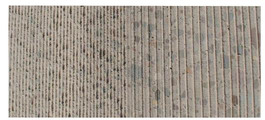
The innovative/ultimate grind (right) has wider and flatter grooves than the conventional diamond grind (left) and can reduce tire-pavement noise over it by as much as 4 decibels, or 67 percent.
