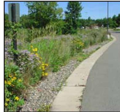
Infiltration Trench - Source: Minnesota Stormwater Manual
