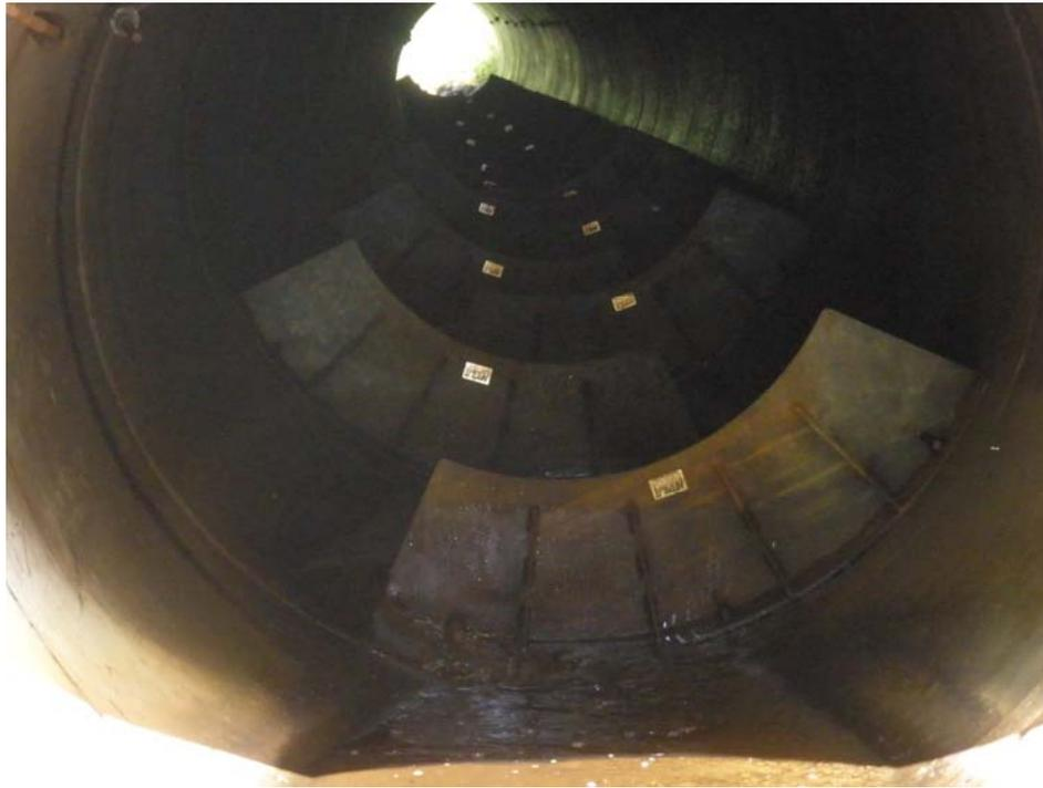
**Figure 4.5. Offset baffles retrofit in round concrete culvert. (St. Louis County).**
