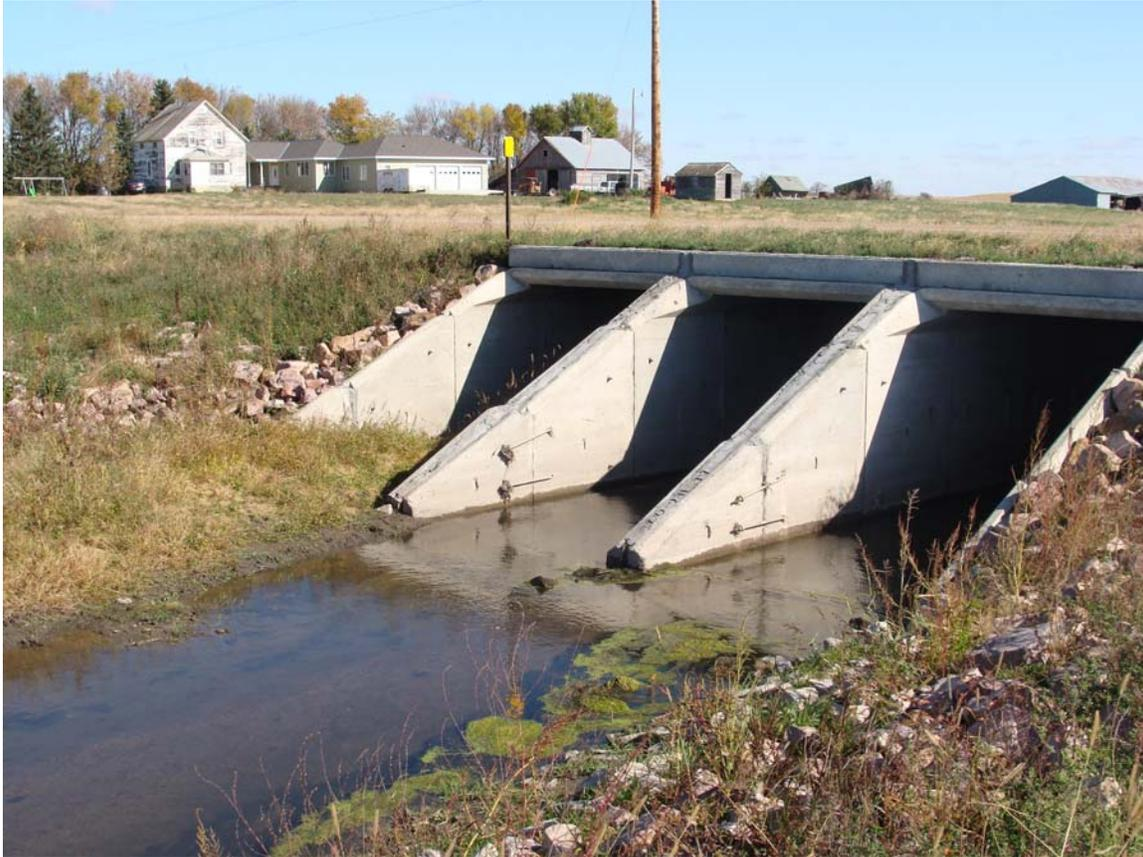
**Figure 4.2. Multiple culverts set at same elevation with one culvert filling in with sediment.**
