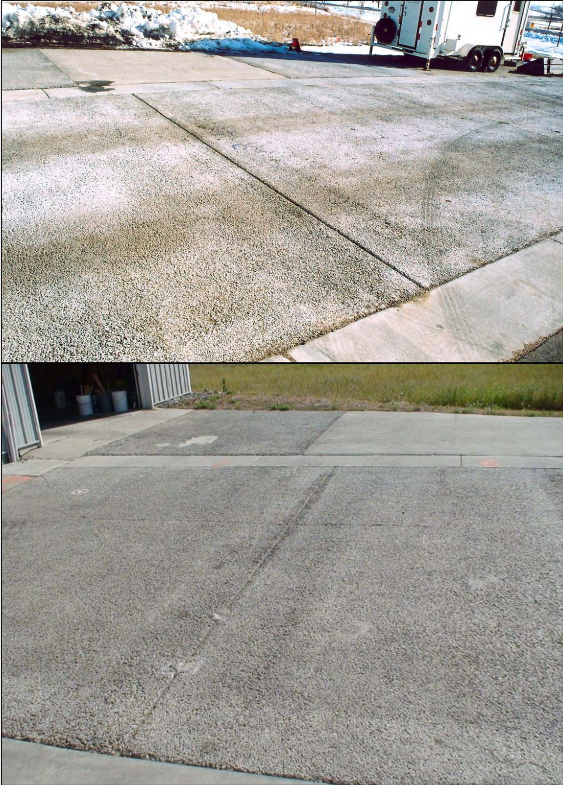
**FIGURE D-1: Tooled joint, Top: 9.21.06, Bottom: 8.11.08.**
