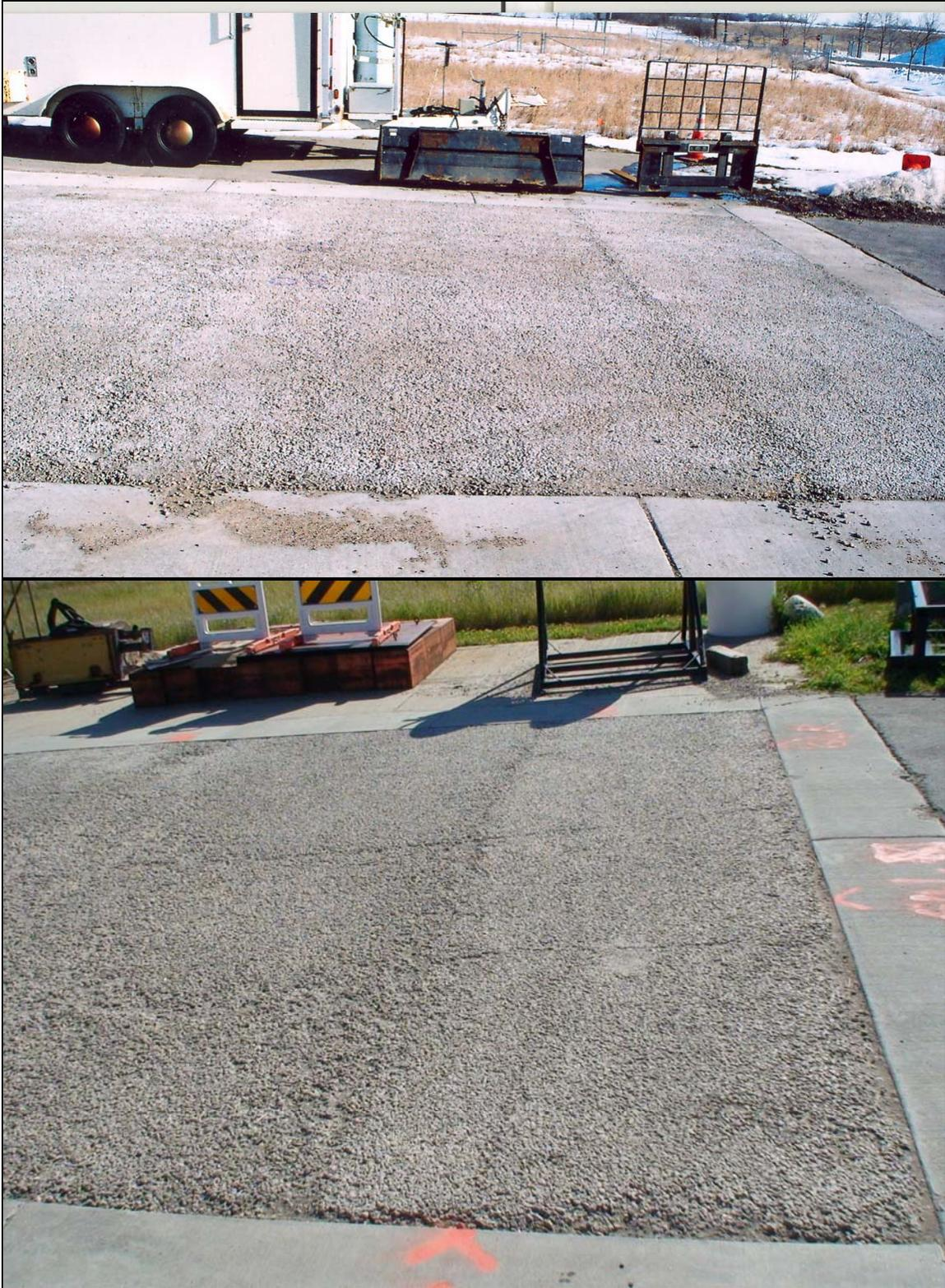
**FIGURE D-4: Coterminous joint at Mixes #2 and #3, Top: 9.21.06, Bottom: 8.11.08.**
