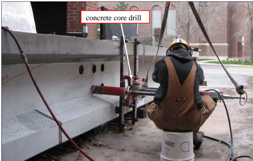
Figure D-6 Setup for taking concrete cores
