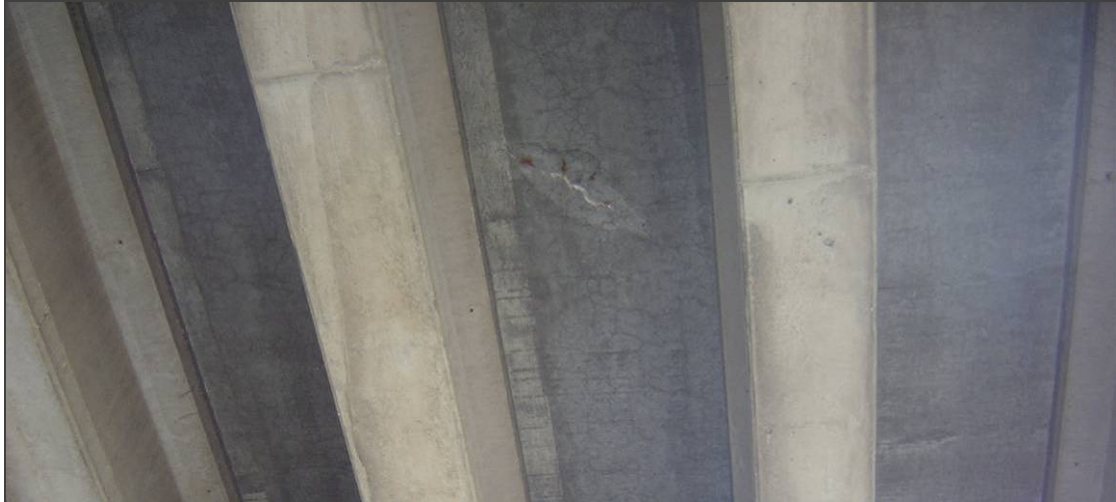
Figure 6.32 Evidence of efflorescence and rust staining on the underside of the deck of bridge 27812.
