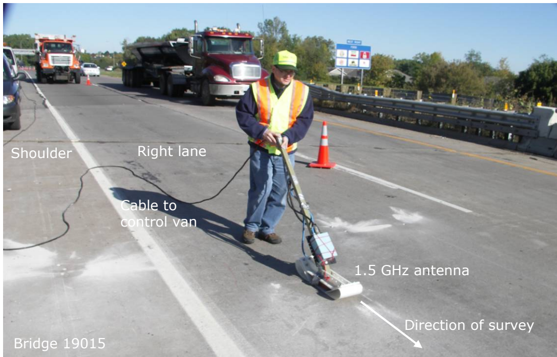
Figure 2.8 Ground Penetrating Radar System used in the imaging of the bridge decks.
