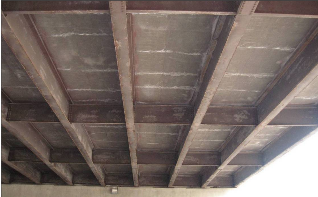
Figure 6.47 Evidence of efflorescence and rust staining on the underside of the deck of bridge 27815.
