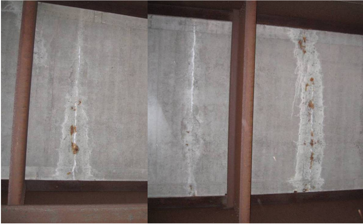
Figure 6.17 Evidence of efflorescence and rust staining on the underside of the deck of bridge 27062.
