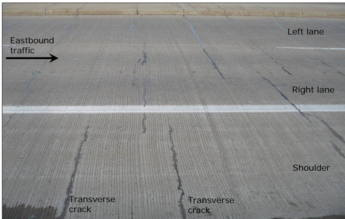
Figure 6.16 Detailed view of transverse cracking on the deck of bridge 27062.
