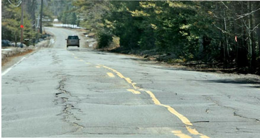
Damp subgrade and pavement may shift during expansion in freezing temperatures, causing frost heave that can severely damage surface conditions and ride quality.
