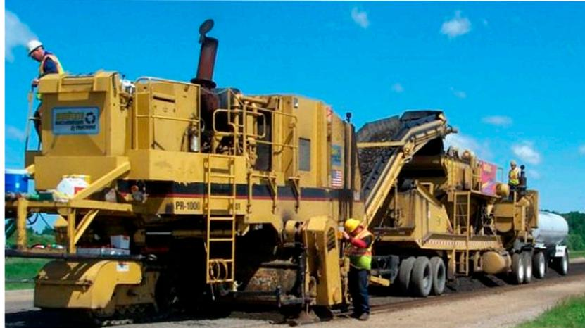
This cold-in-place recycling train is used for reclaiming the surface, conveying and crushing the millings, mixing the recycled material and laying the new cold mix.
