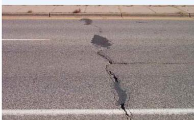
Transverse cracks like these may be repaired by full depth reclamation or cold-in-place recycling, but are too severe for mill and overlay.
