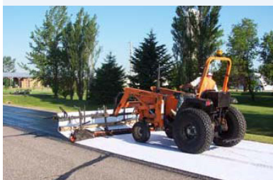
A contractor lays spun-glass paving fabric over asphalt before overlay.
