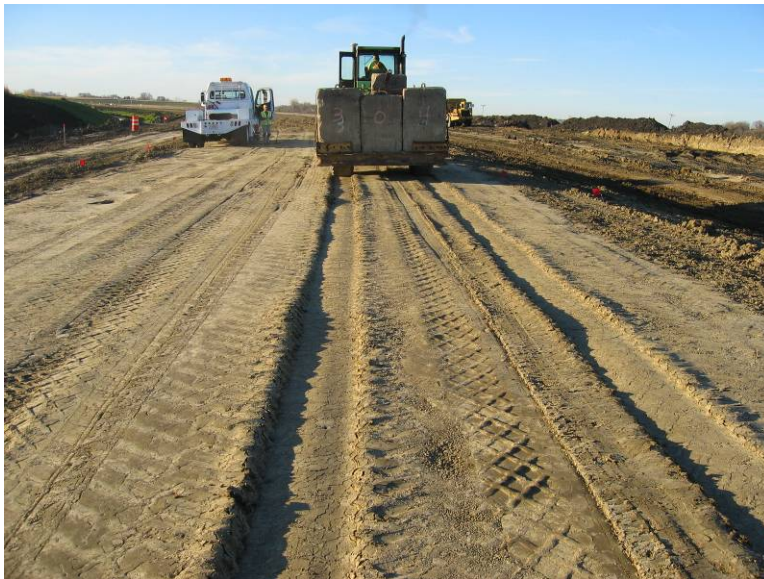
Figure 4.28. Rutting observed following test rolling
