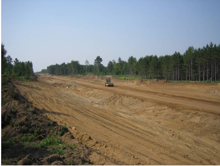
Figure 5.3. TH 64 soil compaction operation at STA 265 (6/29/06)
