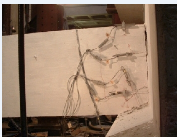
Investigators measured the response of a bridge test section to stresses.
