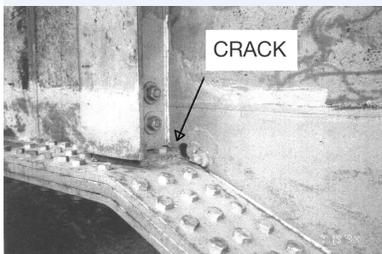
Haunch insert cracking on the Lexington Avenue Bridge is one of the 18 fatigue-critical details that will be represented in Pontis.
