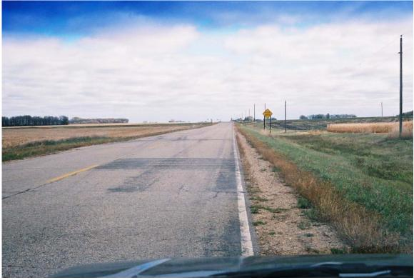
Photograph #8 (Reel #1, 22A) (from West, looking East): first rumble strip and warning sign in view.
