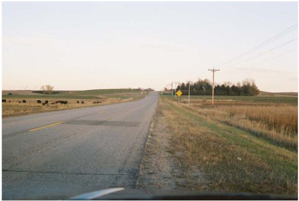
Photograph #68 (Reel #4, 12A) (from West, looking East): first rumble strip and warning sign in view.
