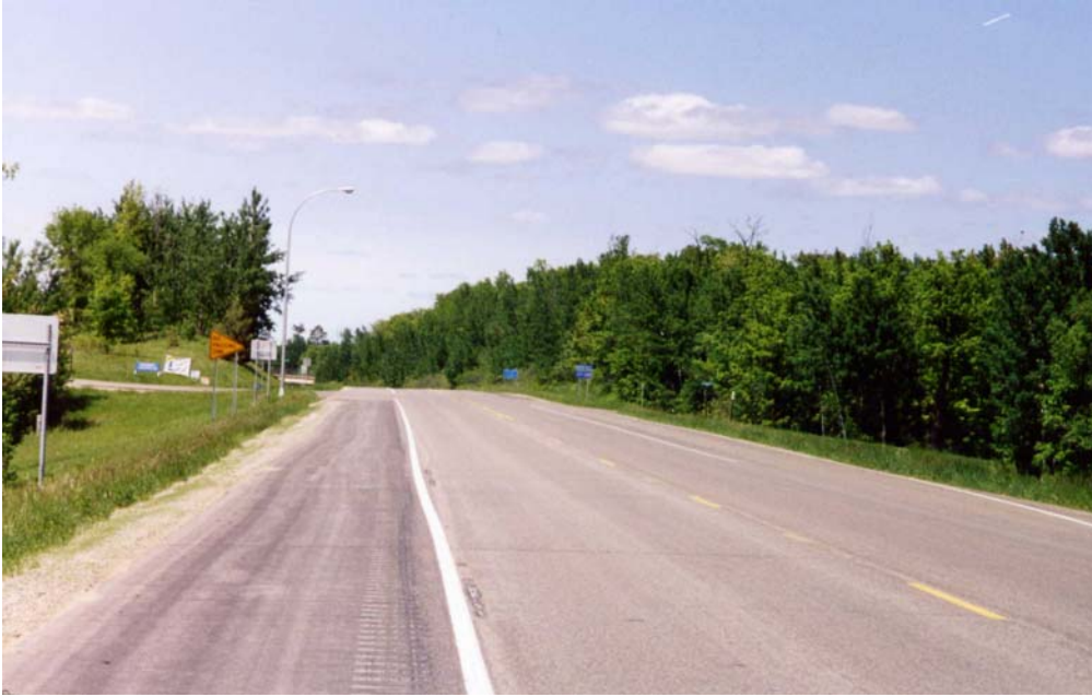
Cass County: TH 371/200 and CSAH 38 (looking north)
