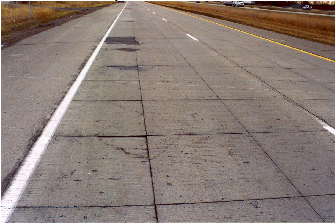
Photo 2.3. Patched corner crack areas near outside wheelpath, May 2004. MnROAD Test Cell 93, driving lane.
