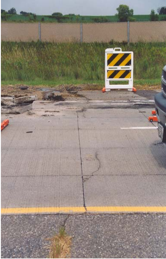
Cell 93 reflective cracking. Facing north (left photo) and south (right photo). 8-25-2004/A-5
