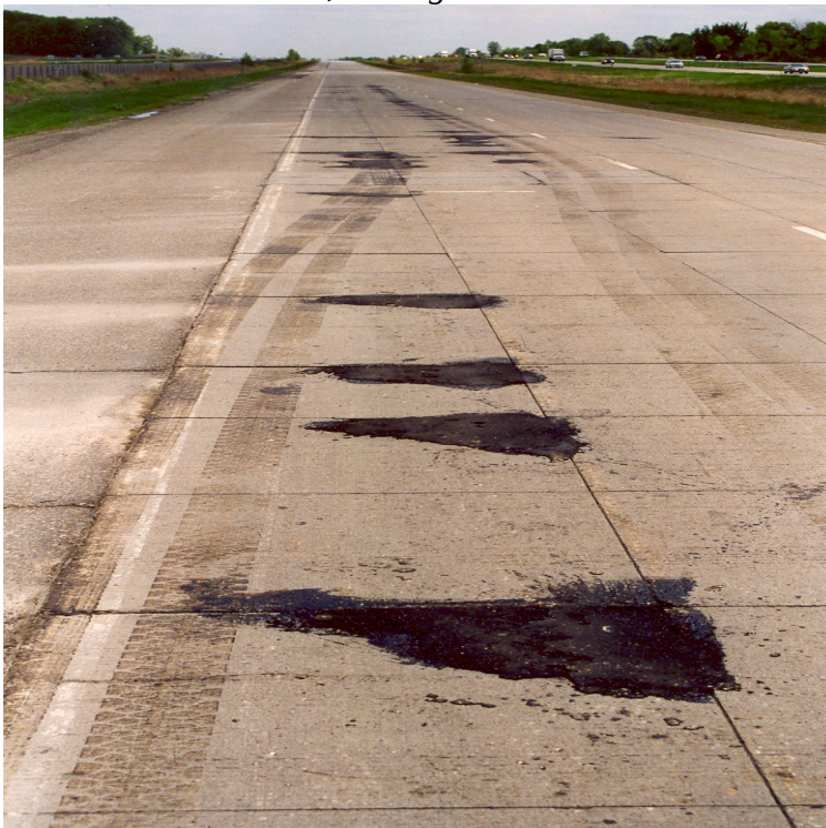
Photo 2.3. Patched corner crack areas near outside wheelpath, May 2004. MnROAD Test Cell 93, driving lane.
