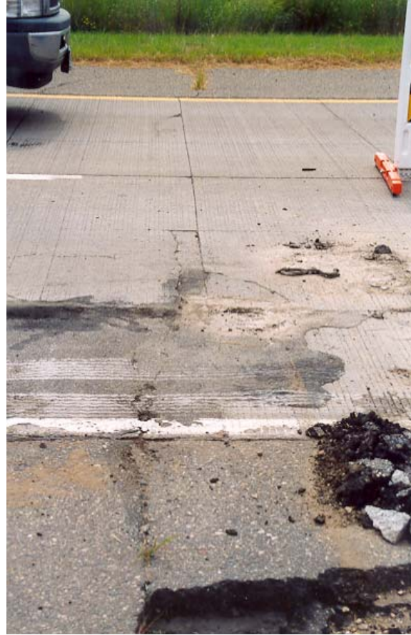
Cell 93 reflective cracking. Facing north (left photo) and south (right photo). 8-25-2004/A-5
