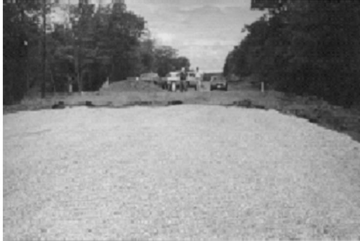
**Figure 3.10. Wood Chips above Geofabric**
