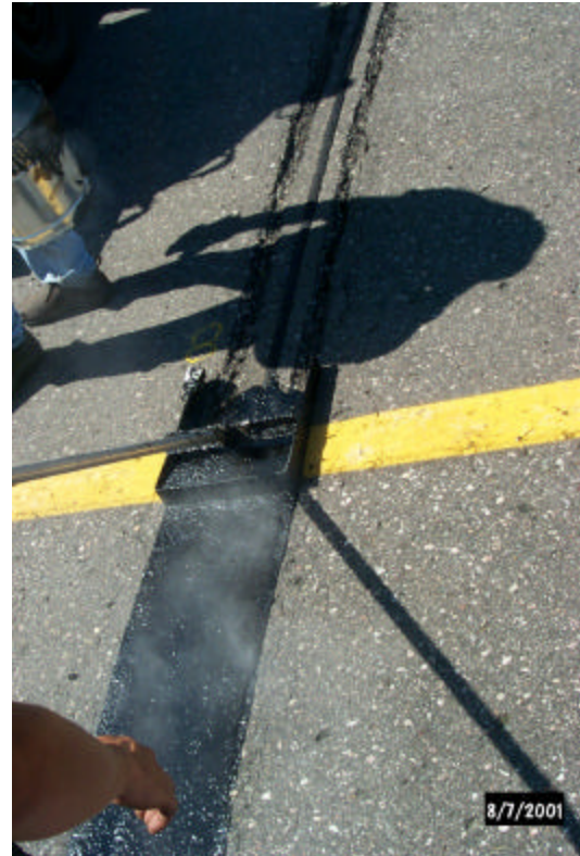
Photo 7. This is the 12-in. wide rake. A 19-in. wide rake was also used.
