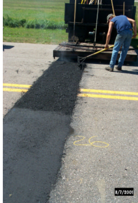
Photo 13. Joint 26, preparing the area for compaction.
