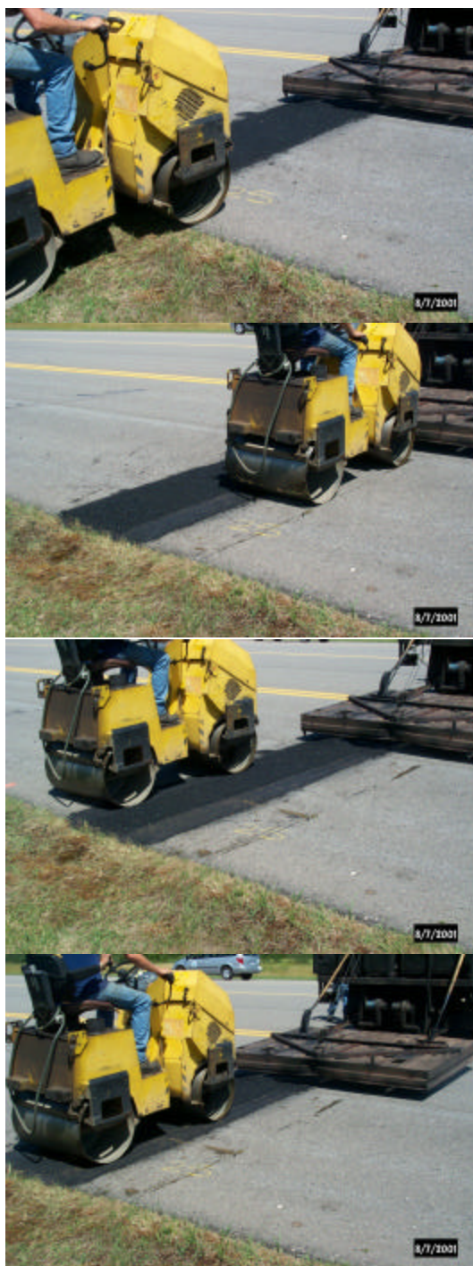
Photos 14, 15, 16, and 17. Compact each edge first, than roll down the center of the patch.
