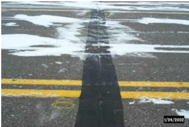
Photo 23. Joint 8 did not appear to be cracked; however joints 2-8 were “skimmed leveled” with joint sealant, approximately two days after placement of the PolyPatch material. The joint sealant may have been masking a small crack in the patching material.
