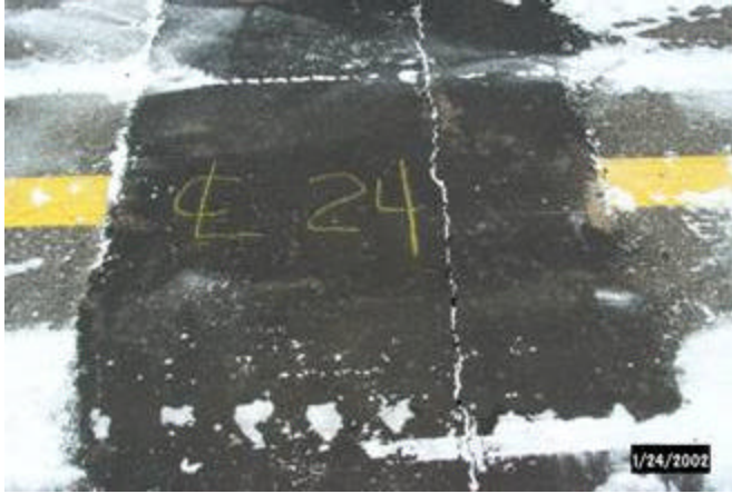
Photo 24. Joint 24. The three joints repaired by the thermo patch method had cracked.
