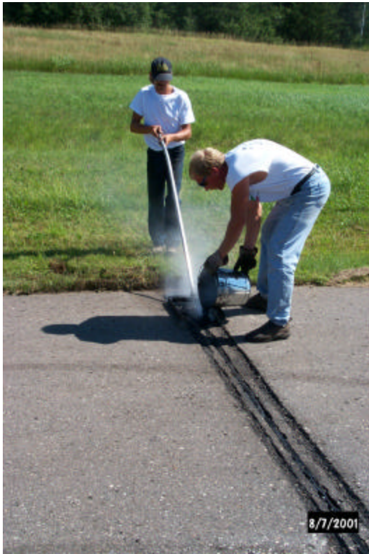
Photo 4. Typical routed joint. Fill from the shoulder toward the centerline. Recommended application temperature is 375-410° F.
