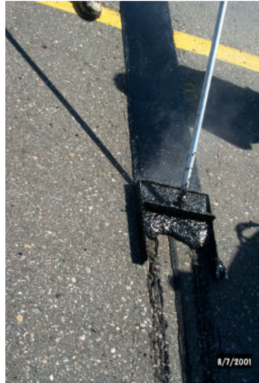
Photo 5. Type 1 material used the larger size aggregate, (vs. the fine mix – type 3). The routed edge provides a better “edge” for the material to bond against.
