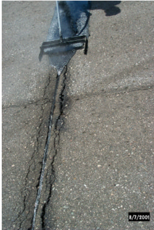
Photo 19. Typical skim patch operation. Clean and dry.
