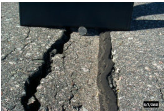
Photo 2. Close up of joint. Severe cupping occurred across the entire joint. The coin is a quarter.
