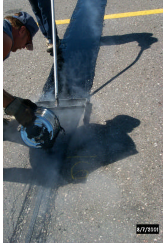
Photo 10. Filling joint 9. This is type 1 material. It will perform better in colder weather than fine mix - type 3. Type 1 has a lower adhesion property than type 3 (15psi vs. 25psi). The routed edge should help the patch material bond to the taxiway. The type 1 also has a larger aggregate size than the fine mix - type 3. Therefore type 1 is better suited for the deeper patches.
