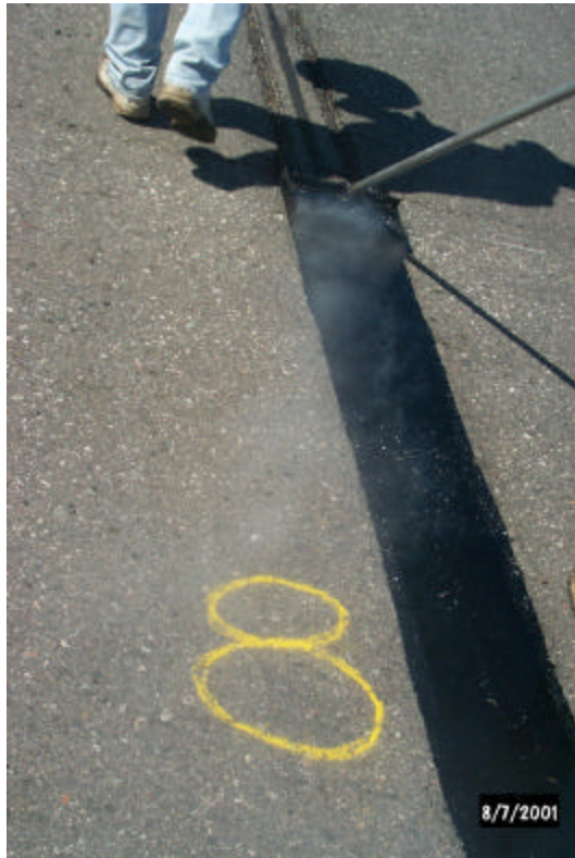
Photo 6. The material easily flowed into cracks and provides a smooth level surface across the joint.
