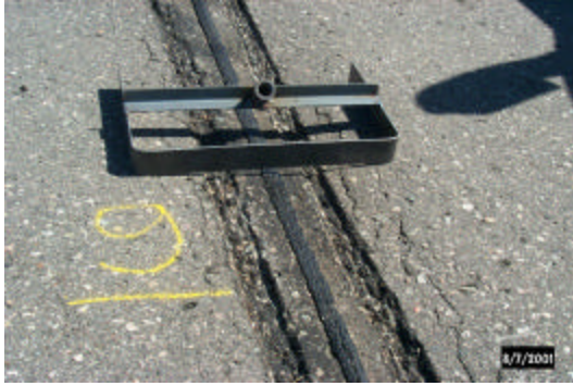
Photo 9. This is joint 9. The 19-in. rake shows that the cupping at the joint was often greater than a foot wide. The router was run across the taxiway on each side of the joint. This provided a better “edge” for the patch material to adhere to.
