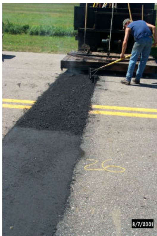
Photo 18. The heating unit progressed across each joint. The sawed and sealed joint will reflect through this repair. The width of this repair is about 41-42 inches.
