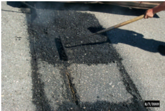
Photos 11 and 12. Raking the heated joint. Additional new fine HMA was added and mixed together with the existing material. The joint will reflect through the patch.
