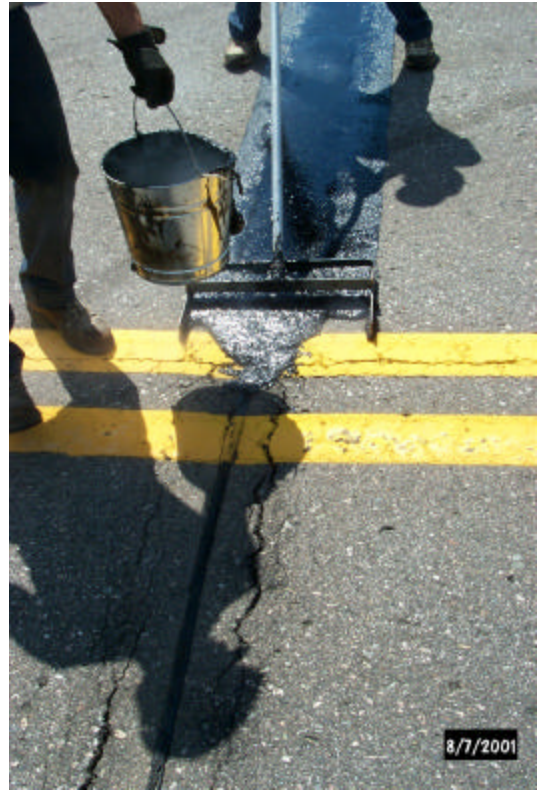
Photo 20. The pavement surface temperatures during this repair work were up to 140° F by mid afternoon.
