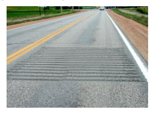
Figure 1-2: In-lane rumble strips, wheelpath
