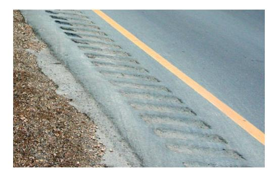
Figure 1-4: Longitudinal rumble strips, clustered
