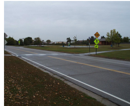
Figure 5-26: Site Conditions – After (view North)
