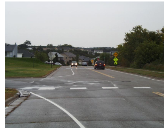
Figure 5-27: Site Conditions – After (view South)
