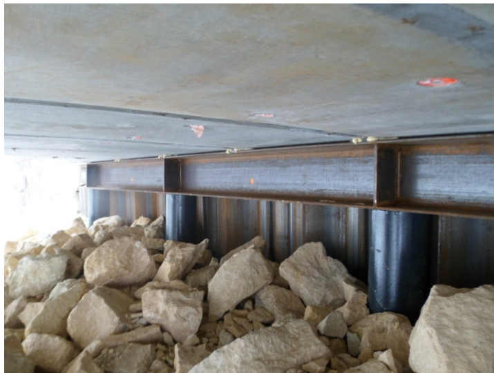
3-2 Blue Earth County Bridge 07593 Sheet Pile Abutment
