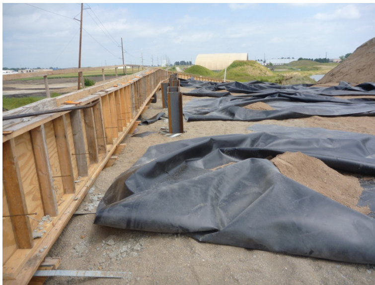
A4-5 MSE Wall and Abutment Piles for Bridge 74551
