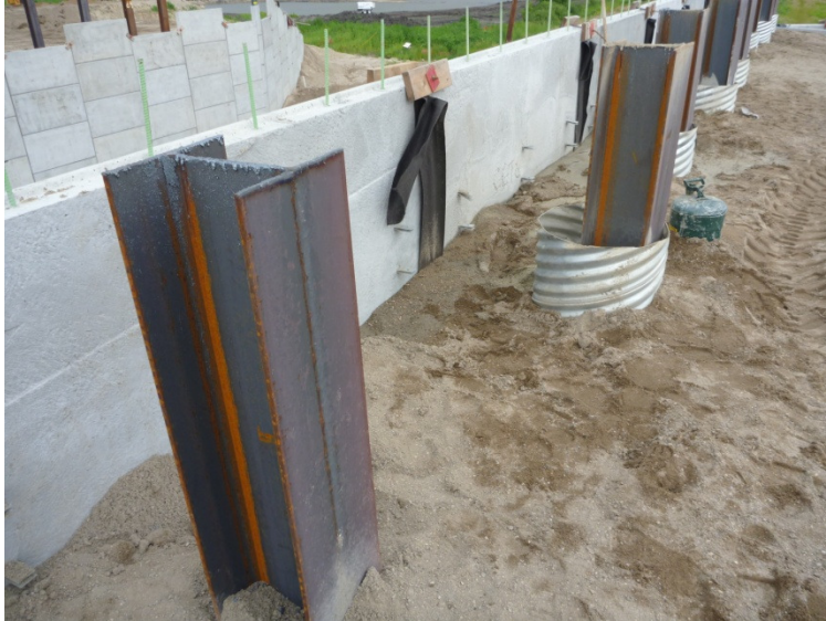
A4-4 MSE Wall and Abutment Piles for Bridge 74551
