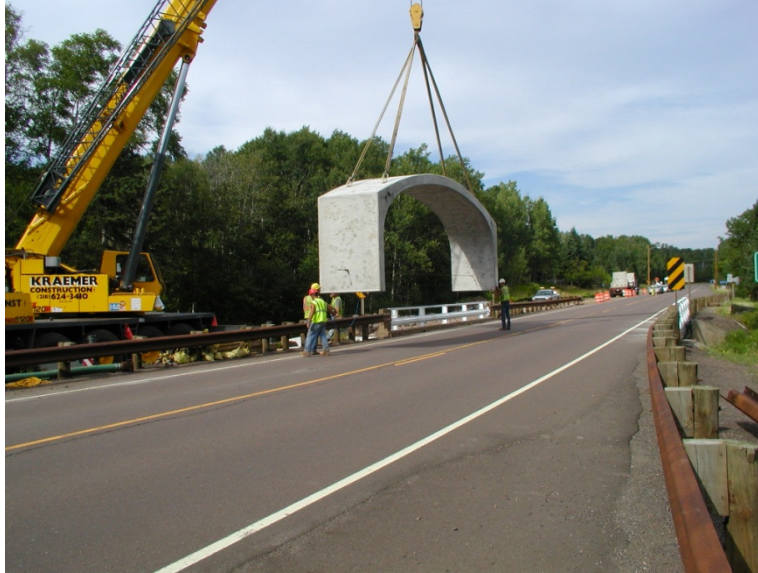
A6-2 MnDOT Bridge 16X03 over Kimball Creek; 32-foot span (courtesy of Cretex Concrete Products)
