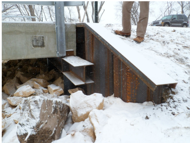
A3-5 Sheetpile abutment wing at Bridge 07593
