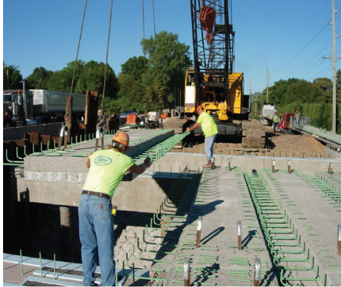
2-1 Setting precast inverted tees for MnDOT bridge
