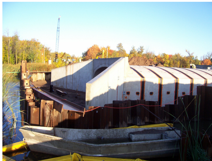
6-2 Morrison County Bridge 49J44
