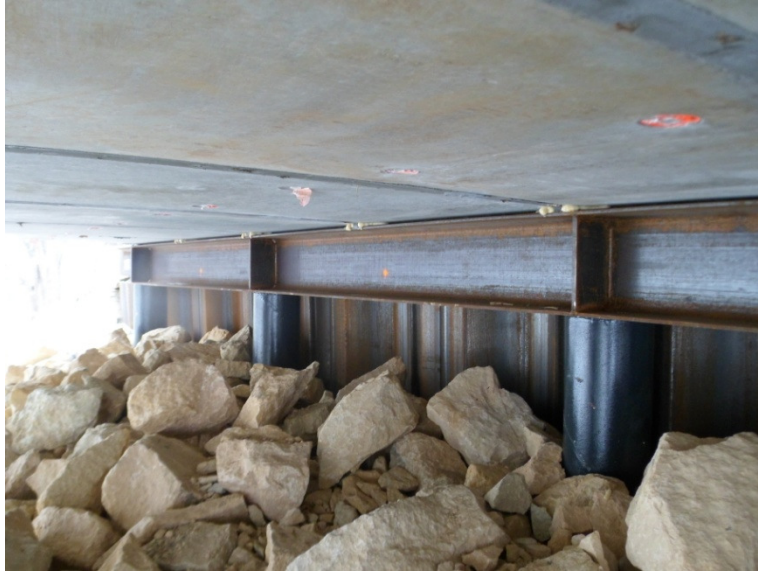
A3-4 Sheetpile abutment at Bridge 07593
