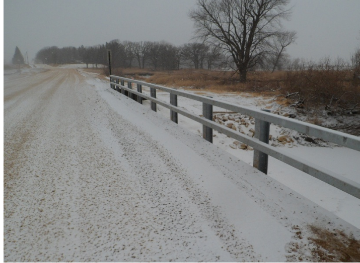
5-2 Blue Earth County Bridge 07593
