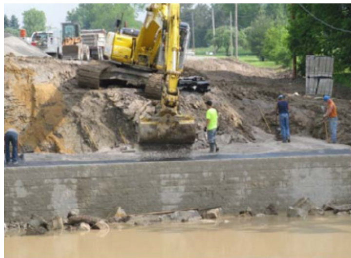
1-1 Example of GRS Abutment (courtesy of FHWA)
