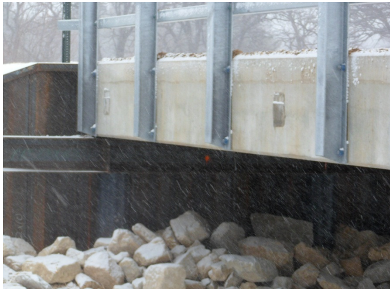
A5-5 Two-Line Railing Attachment on Blue Earth Co. Bridge 07593
