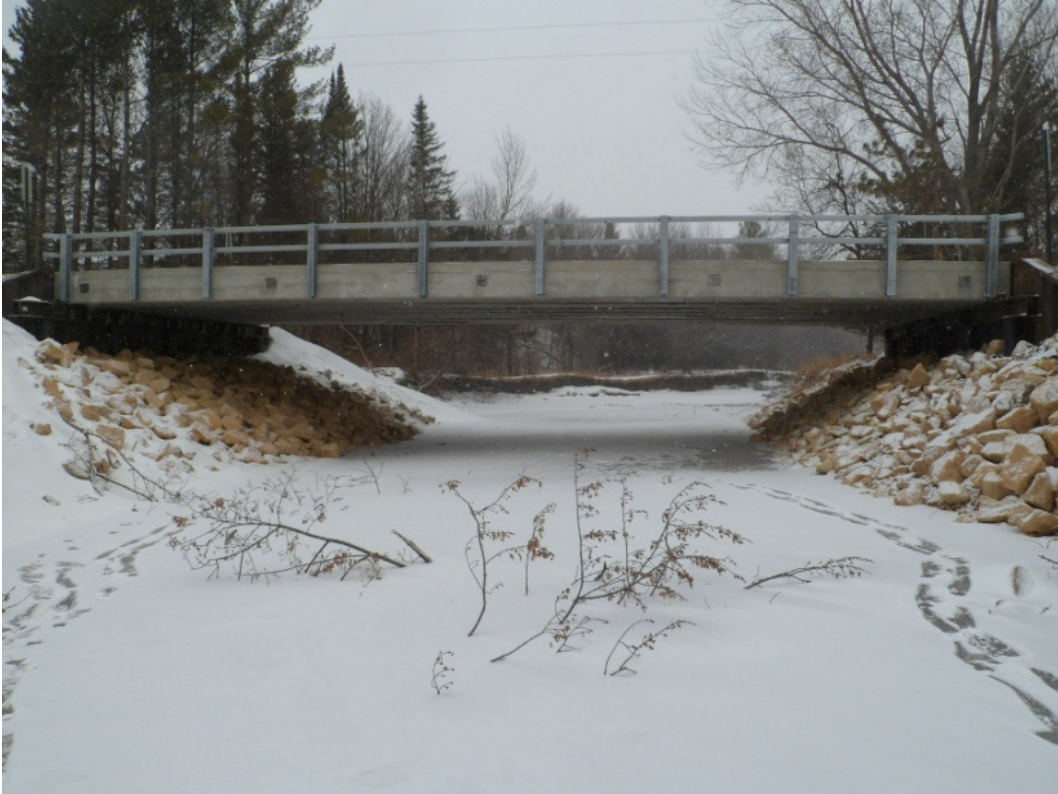
3-1 Blue Earth County Bridge 07547 Precast Box Beams and Sheet Pile Abutments
