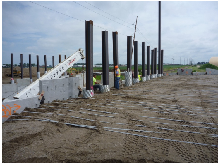
A4-3 MSE Wall Construction for Bridge 74551
