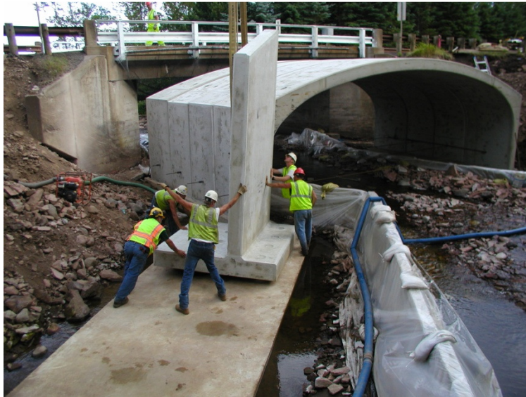
A6-3 MnDOT Bridge 16X03 over Kimball Creek; 32-foot span (courtesy of Cretex Concrete Products)
