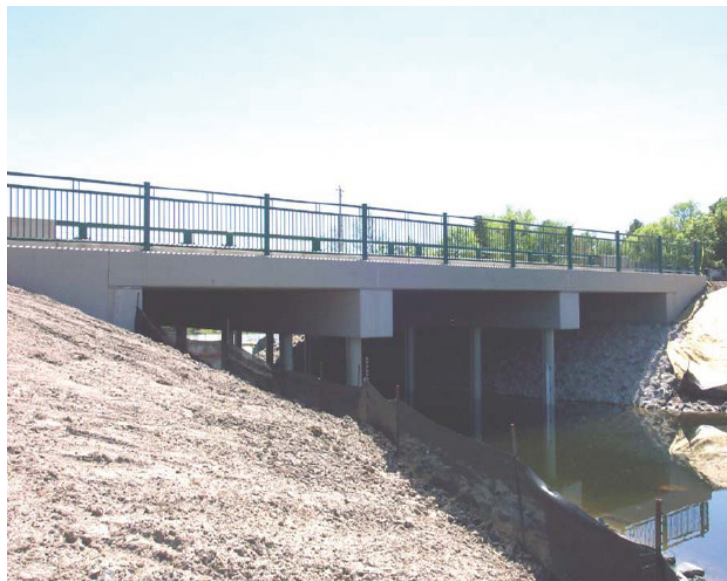
A2-3 MnDOT precast inverted tee Bridge 13004
