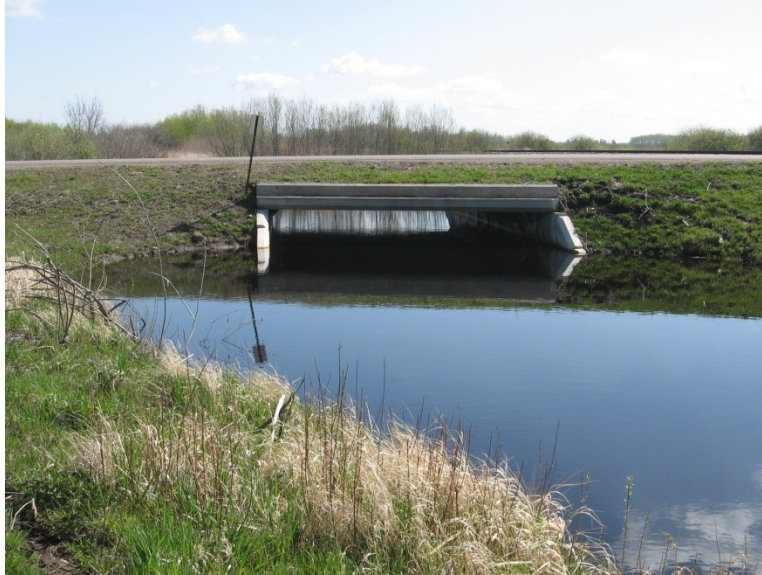
6-1 Aitkin County Bridge 01J31
