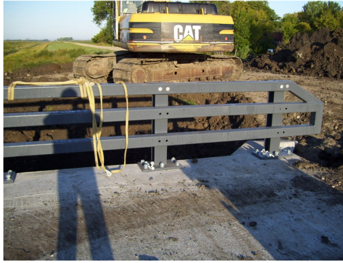
5-1 Polk County Bridge 60559 Metal Railing
