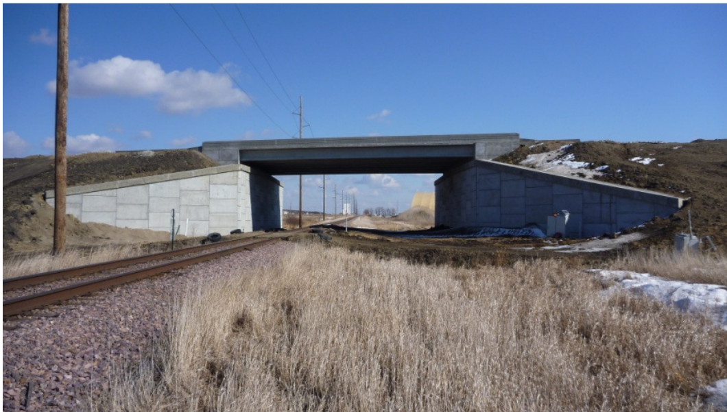
4-1 Steele County Bridge 74551
