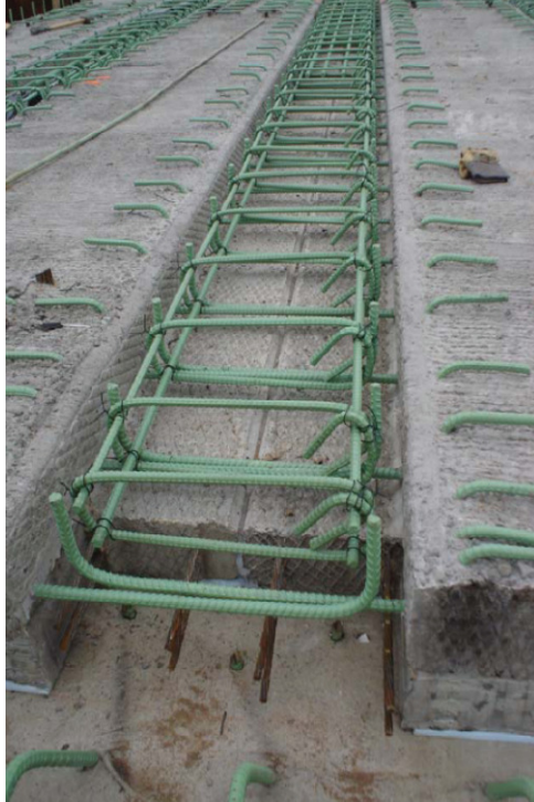
A2-2 Drop-in reinforcing cage between inverted tee sections
