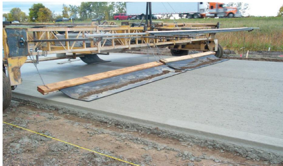
Turf drag is the texture most commonly used by MnDOT for concrete pavement surfaces because it provides good skid resistance while causing less noise than other textures.
