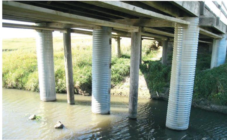
Concrete pile jackets—concrete-filled steel shells installed to strengthen timber piles weakened by minor to moderate deterioration—are one of the rehabilitation procedures detailed in the timber bridge repair manual.
