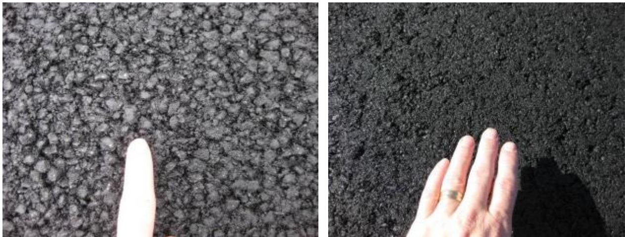
**Figure 3.3 Ultra-Thin Bonded Wearing Coarse [Left], Warm Mix Asphalt [Right]**
