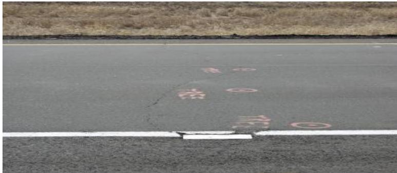
**Figure 2.31 4.75 mm Aggregate Asphalt (Cell 6), August 2009**
