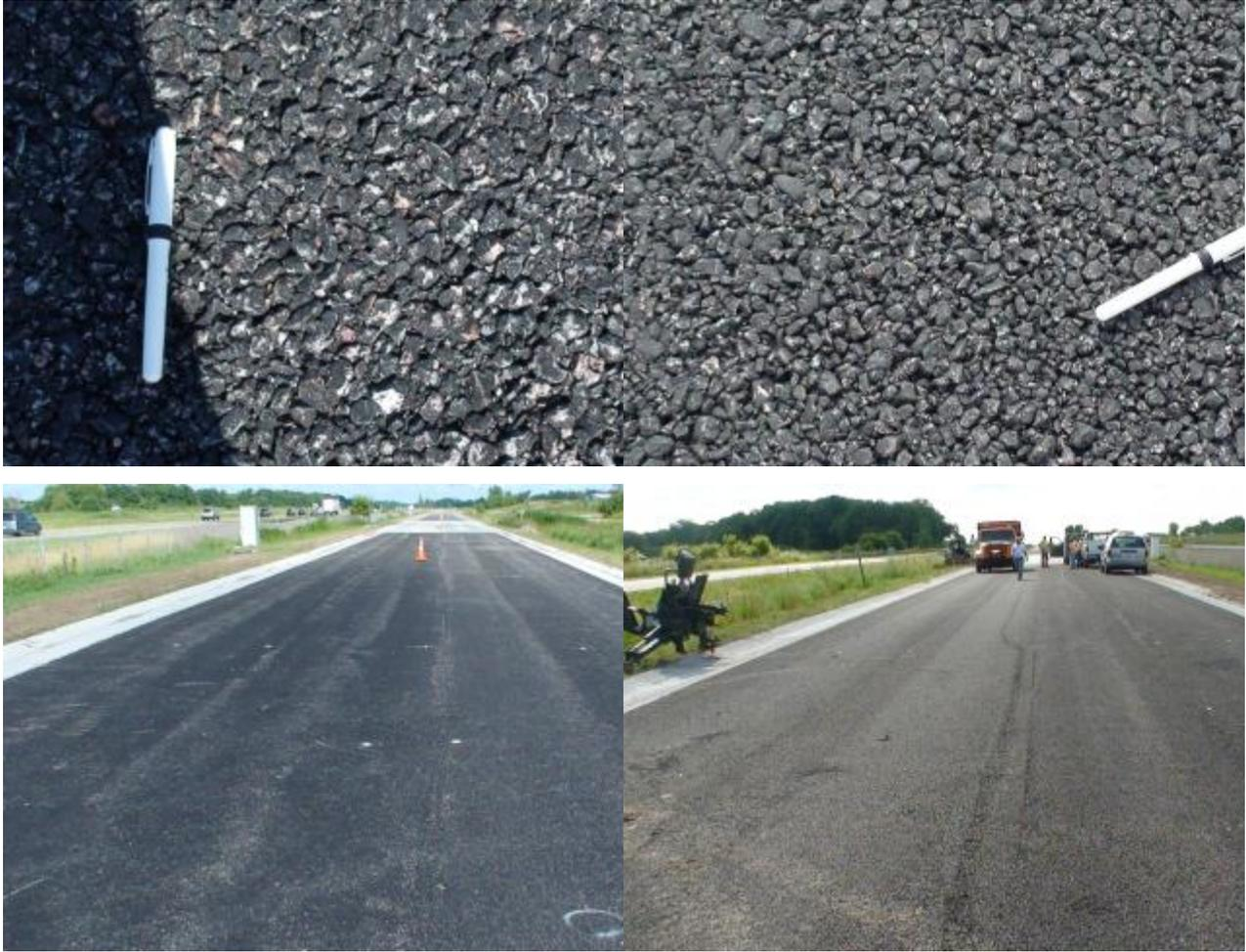
**Figure 2.30 Porous HMA (Cell 86 LEFT, Cell 88 RIGHT), August 2009**
