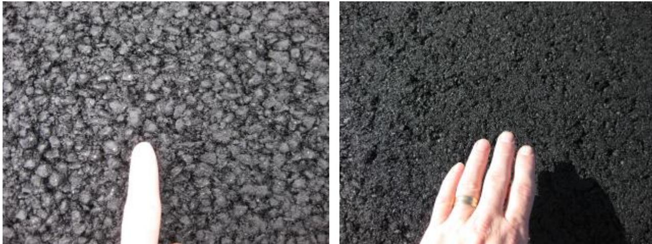
**Figure 2.8: Nova Chip Surface (Left) and Warm Mix Surface (Right)**
