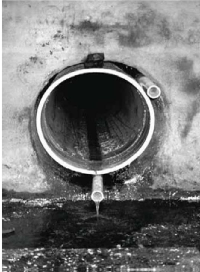
Figure 4.4 PVC Slipliner and Grout Injection Pipes (FHWA, 2010)
