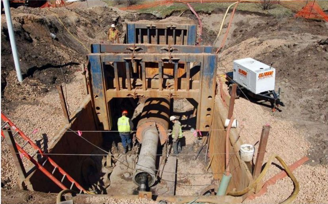
Figure 7.5 Pipe Ramming (CNA Consulting Engineers)
