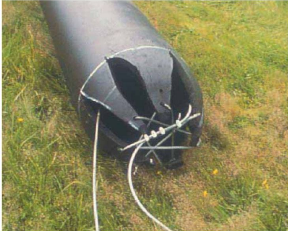
Figure 4.8 Bullet-Shaped Nose on HDPE Slipliner (FHWA, 2010)
