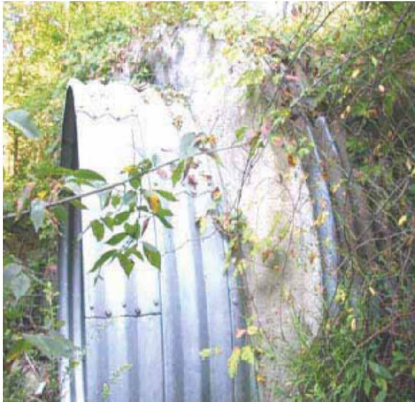
Figure 4.5 CSP Slipliner, Grouted inside CSP Culvert (FHWA, 2010)
