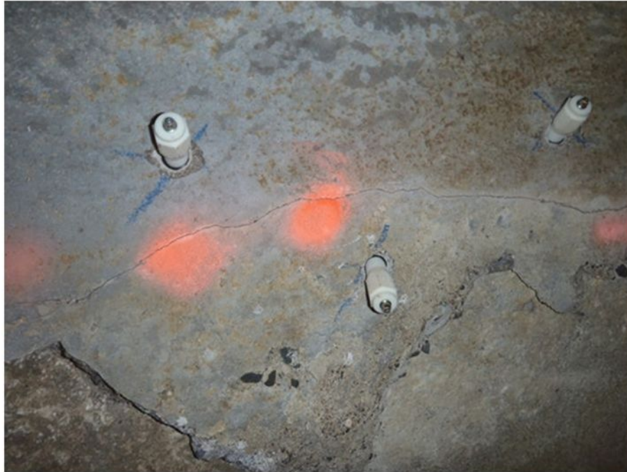
Figure 5.3 Grout Injection Ports on a Concrete Crack (CNA Consulting Engineers)
