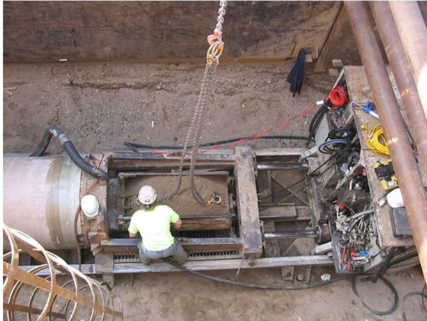
Figure 7.2 Pipe Jacking (CNA Consulting Engineers)
