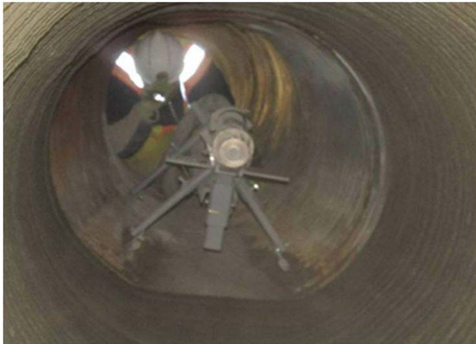
Figure 4.9 Centrifugally Cast Liner Installation (Betcher, 2010)
