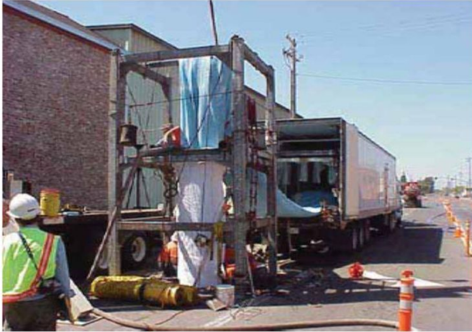
Figure 4.3 Cured-in-Place Pipe Installation by the Inversion Process (FHWA, 2010)
