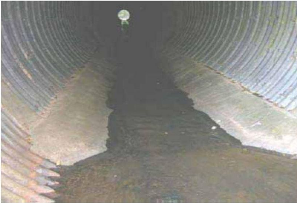
Figure 4.2 Paved Invert in CSP (FHWA, 2010)
