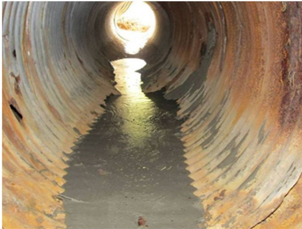
Figure 5.4 Filling Voids below a CSP Culvert (Betcher, 2010)
