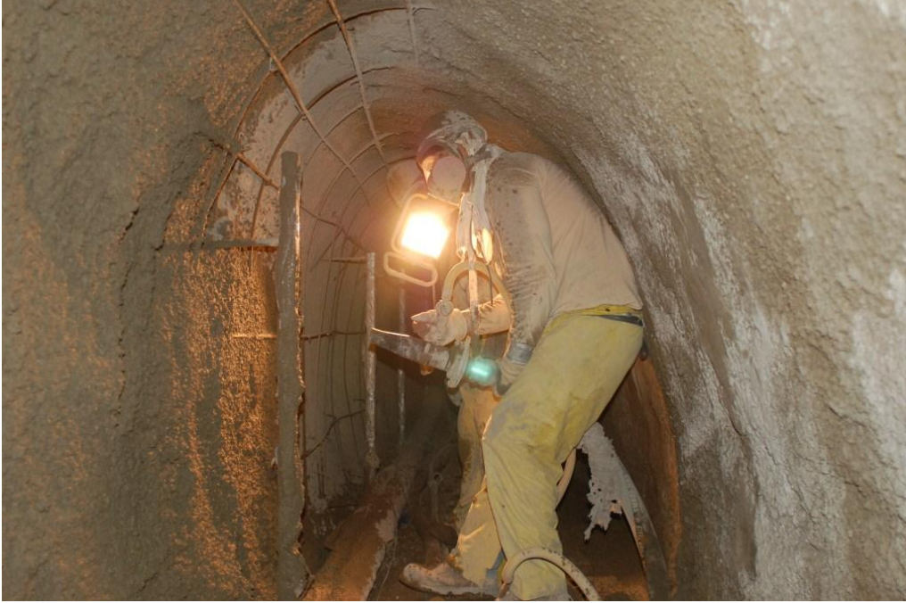
Figure 4.12 Shotcrete Placement over Reinforcing Bars (CNA Consulting Engineers)
