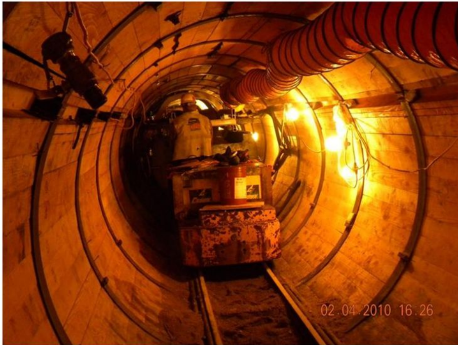
Figure 7.1 Conventional Tunnel, Circular Steel Beams and Wood Lagging (CNA Consulting Engineers)
