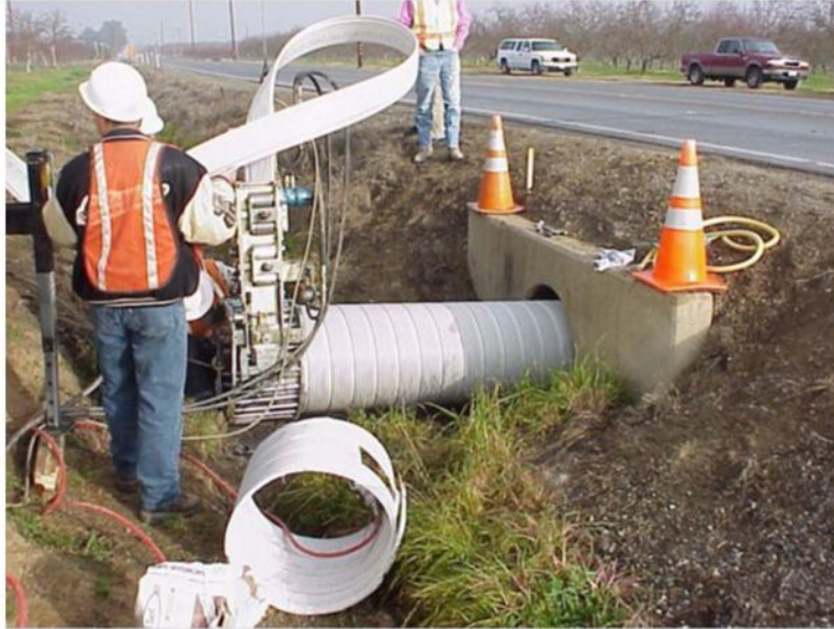
Figure 4.10 Spirally Wound Liner Installation (Caltrans, 2011)
