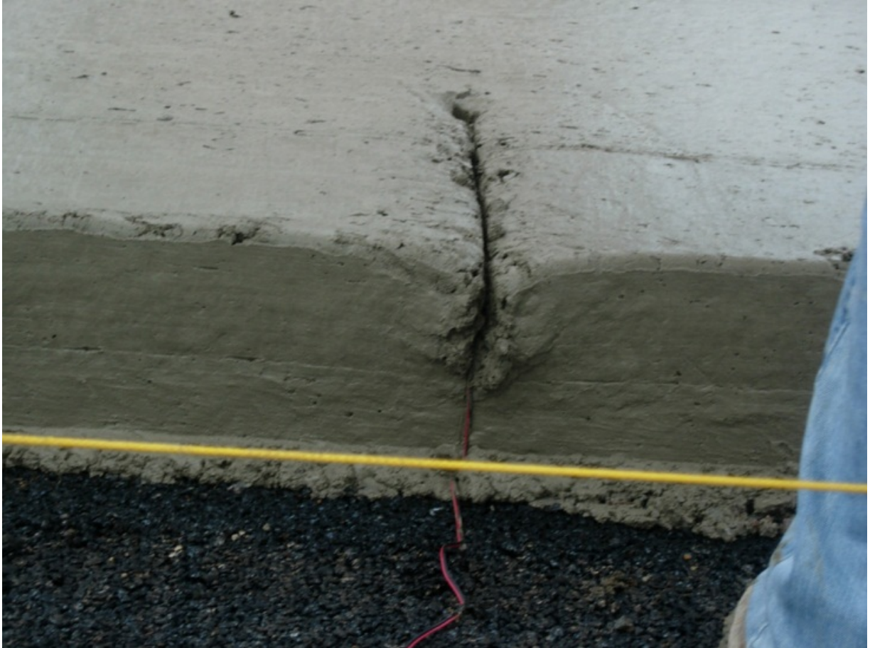
Figure 7: IntelliRock sensor installation.
