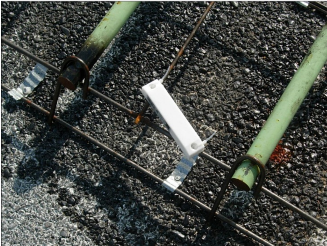
Figure 4: iQtag sensor installation on dowel basket.
