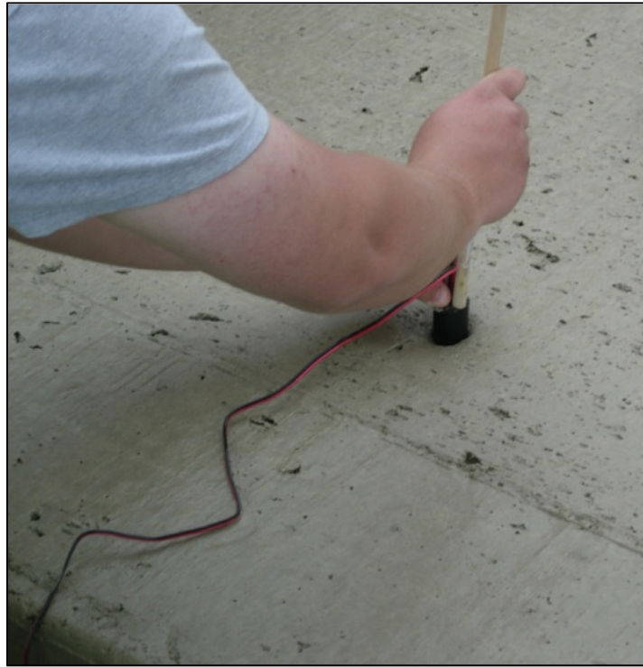
Figure 5: IntelliRock sensor installation.
