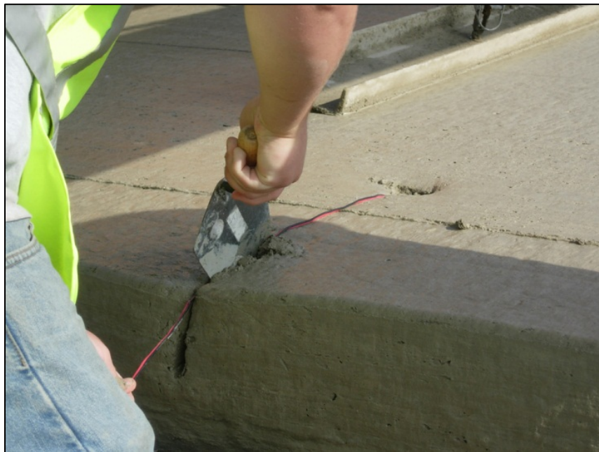
Figure 6: IntelliRock sensor installation.
