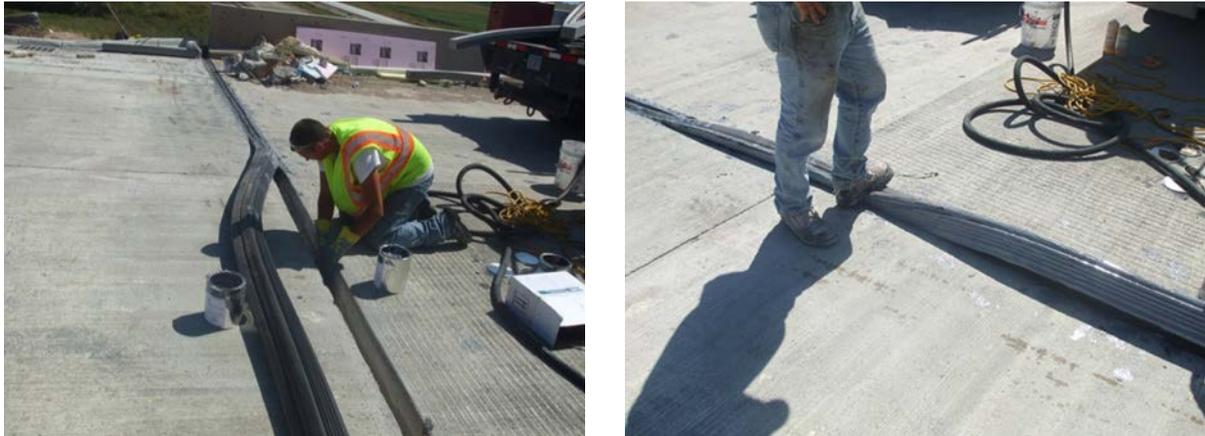
**Figure 28: Installation of D.S. Brown JP series compression seal.**
