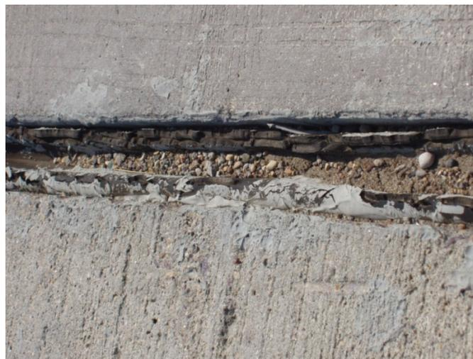
**Figure 27: Failed JP-series compression gland.**
