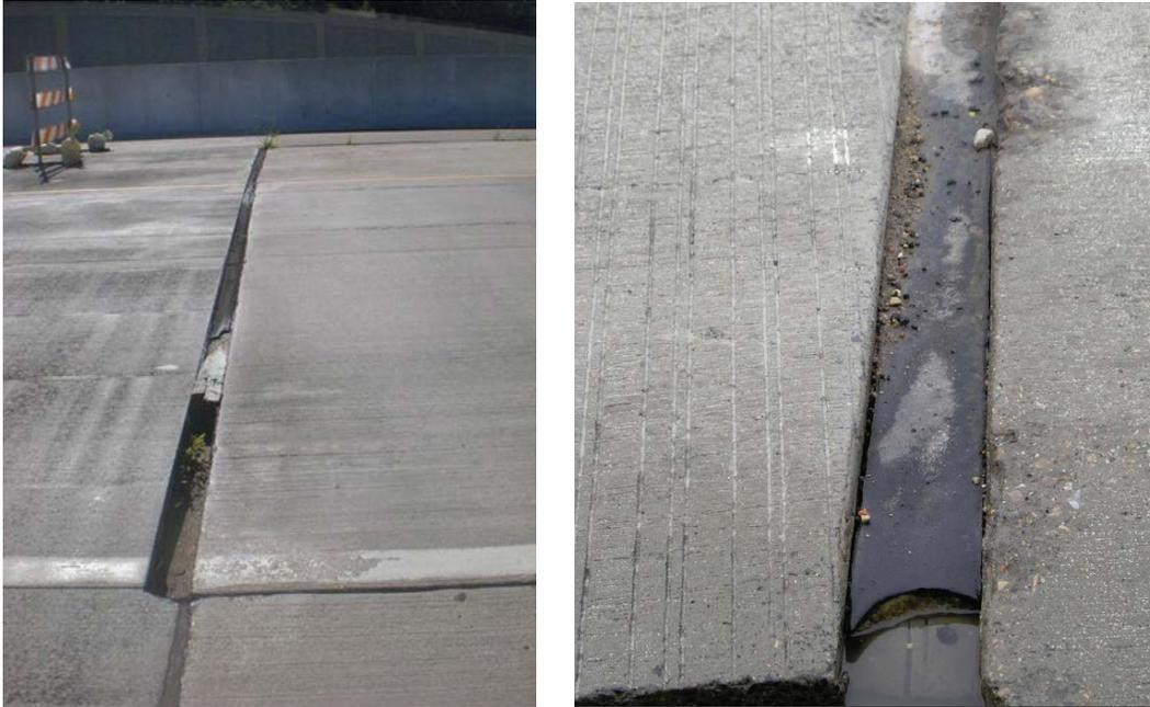
**Figure 6: Failures of E8 expansion joints.**
