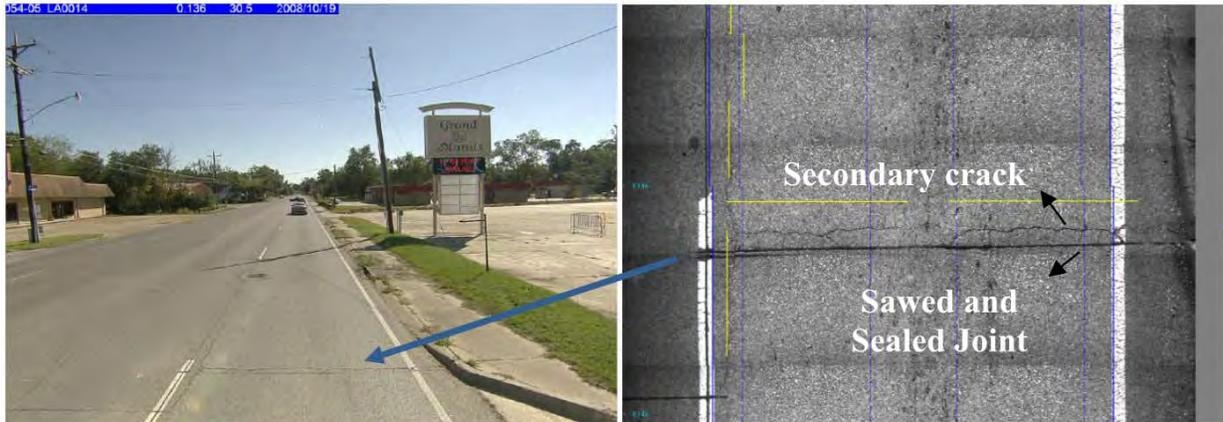
**Figure 5-16: Illinois tollway saw-and-seal (Elsefi 2011).**
