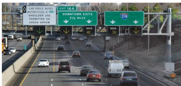
Figure 2: Managed Lane on I-35W
