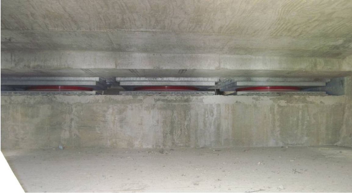
Figure B.12: Northbound Bridge Pier 3 Bearing Pad Assemblies
