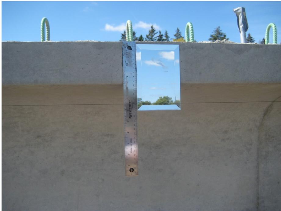
**Figure 4-3. Ruler and mirror located at midspan**
