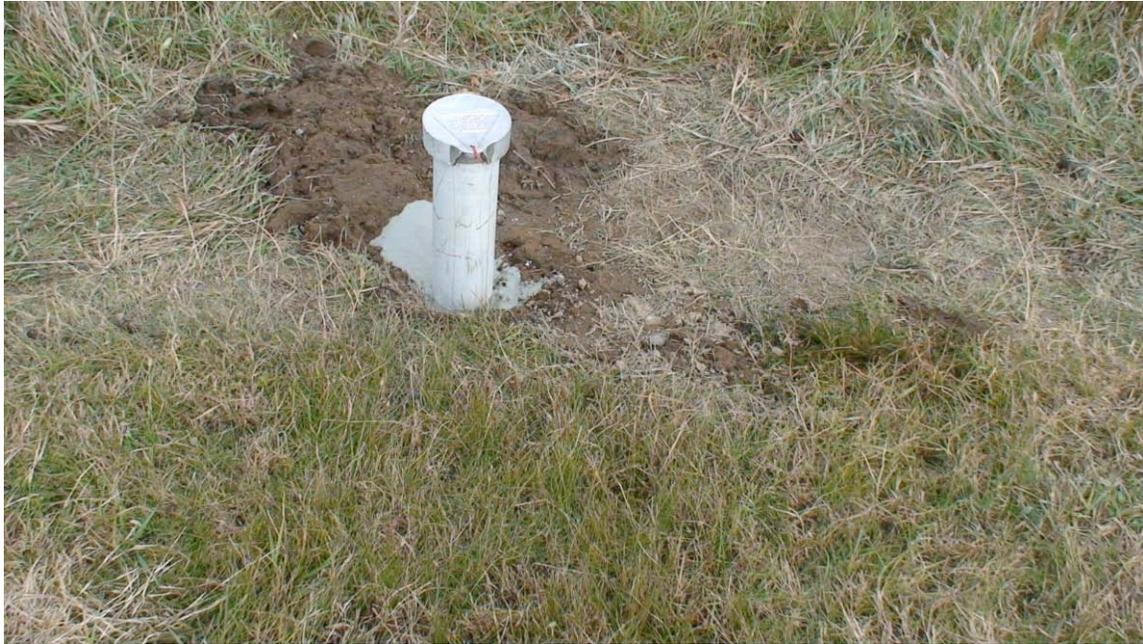
**Figure 2.11: Pervious Well 1 Completed Sand-and-Gravel-Packed, Bentonite-Slurried Cased and Capped**
