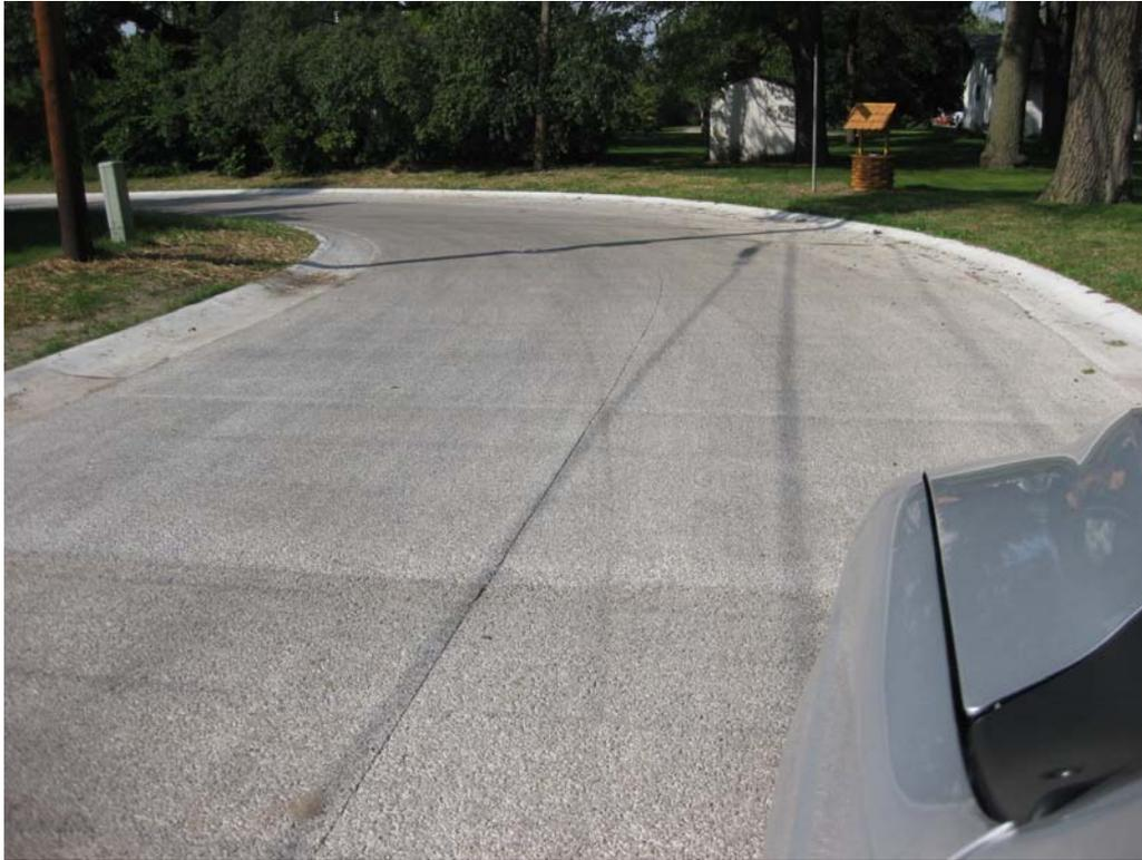
**Figure 7.5: Pervious Concrete in Shoreview**
