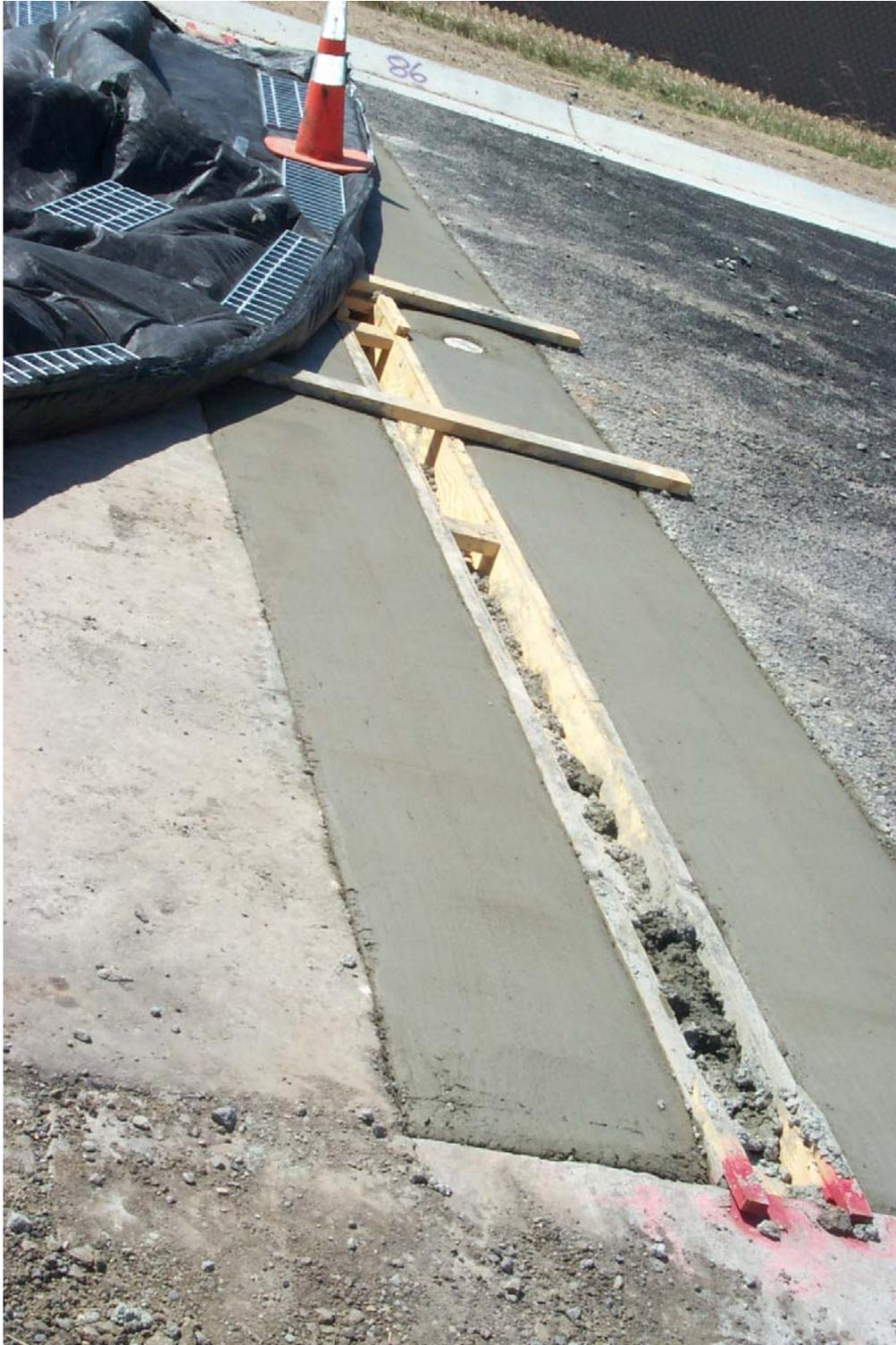
**Figure G6: Cross-Drain Cell 85/Cell 86 Forming and Placement**
