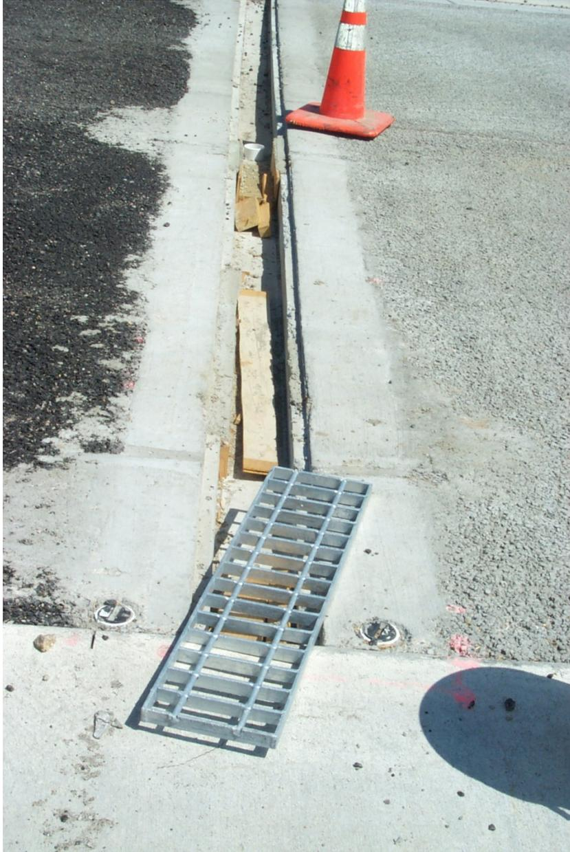
**Figure G3: Cross Drains and Grating**
