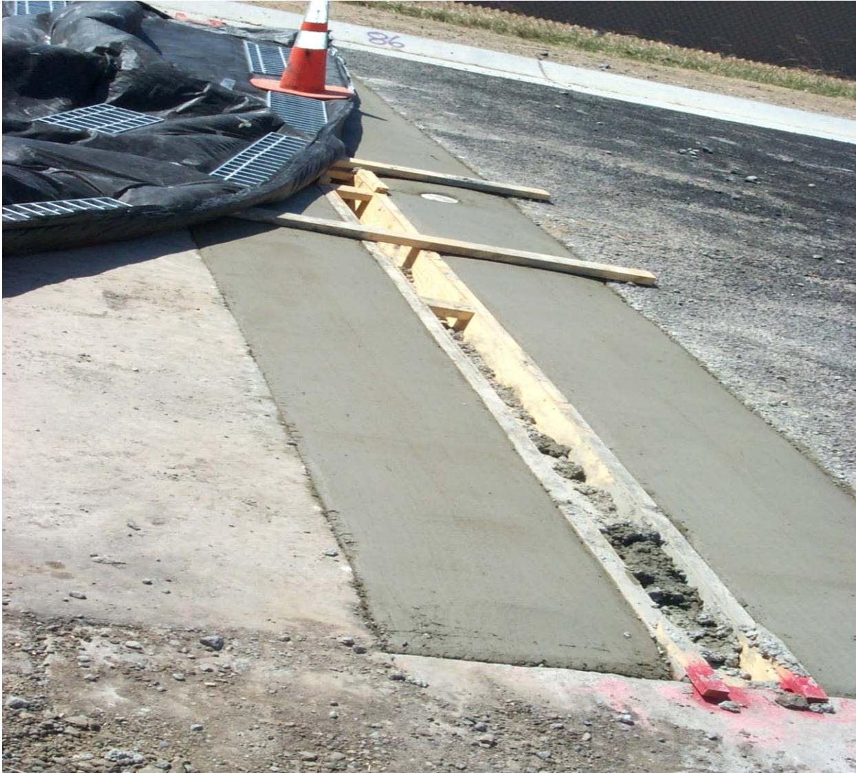
**Figure 3.12: Cross Drain Construction between Porous Cell 86 and Control Cell 87**
