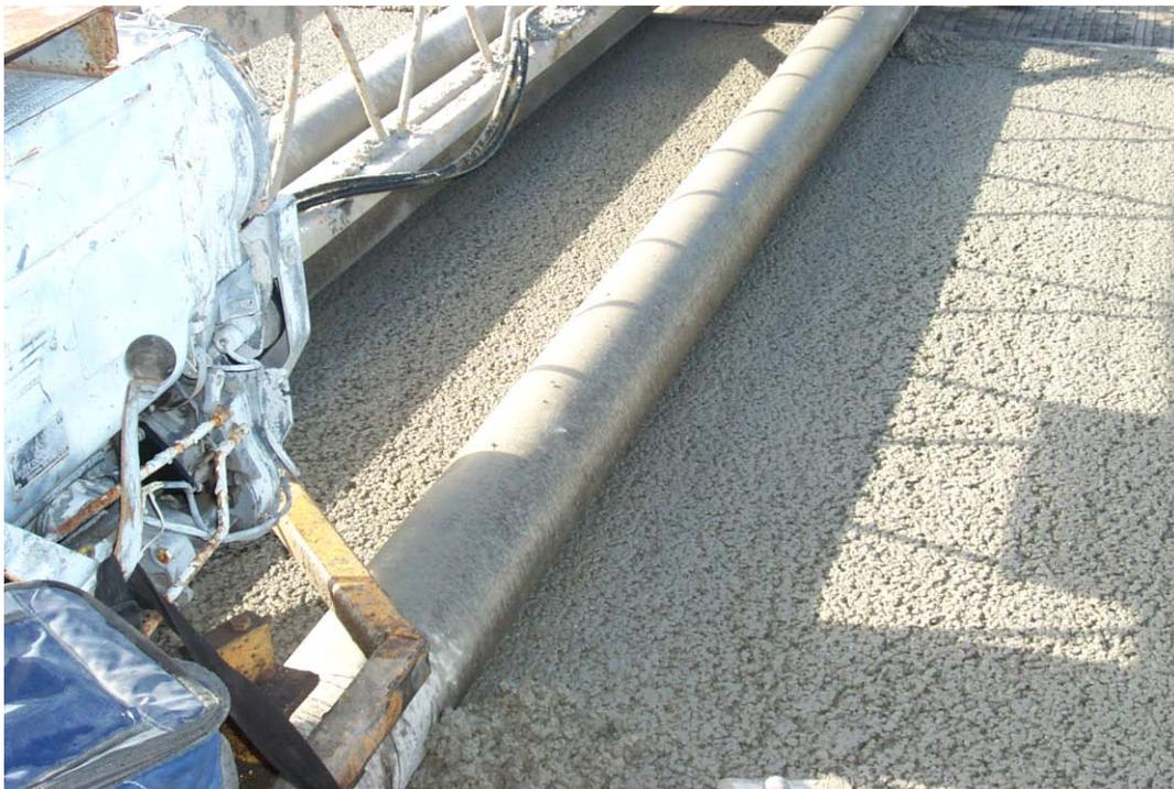
**Figure 3.7: Porous Overlay Multi-Drum Screed Compactor**
