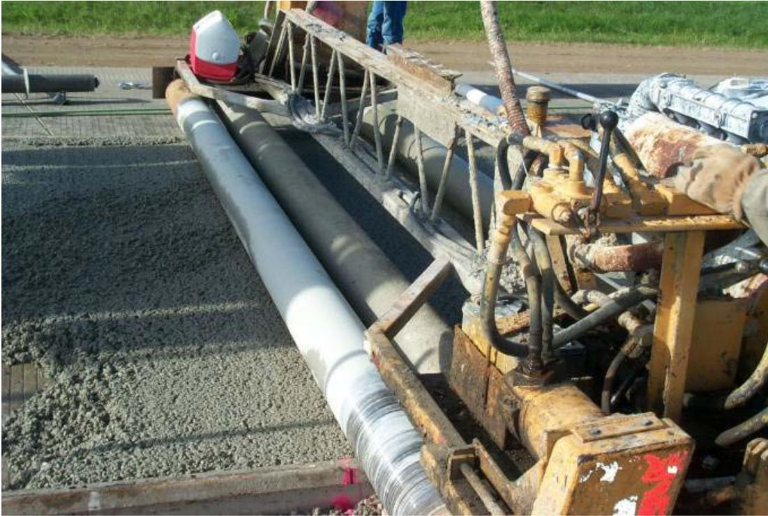
**Figure 3.6: Porous Overlay Compaction**
