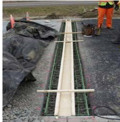
**Figure 5.2: Transverse Drains in Cells 85-89**
