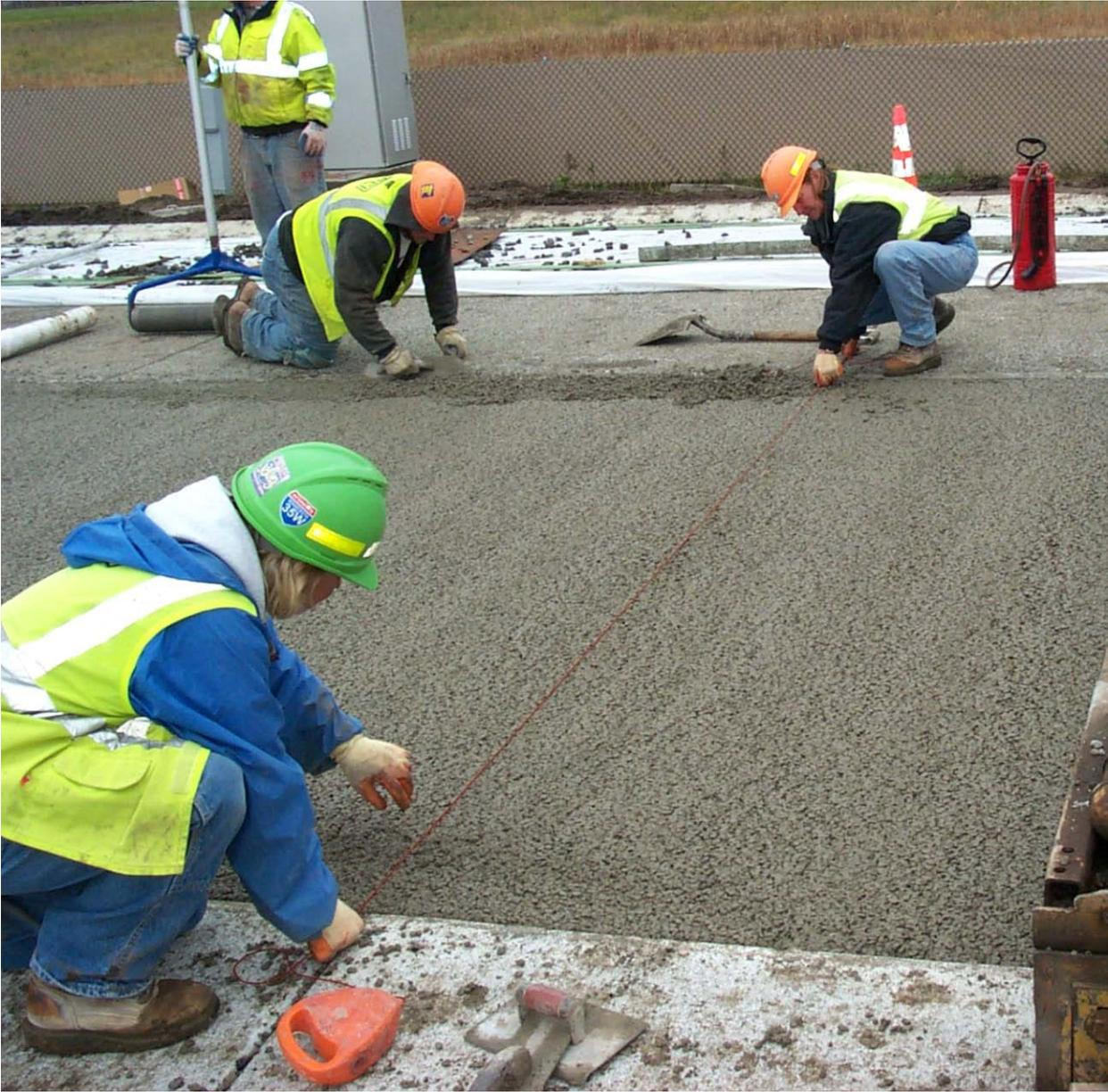
**Figure 3.10: Establishing 10 Ft Joints in Cells 85 and 89**
