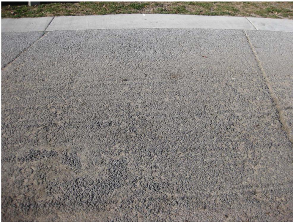
**Figure 7.1: Detroit Lakes Pervious Concrete**
