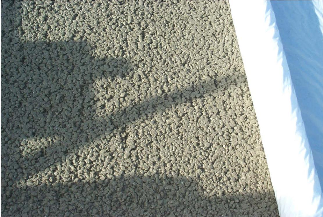
**Figure 3.8: Porous Overlay Surface**
