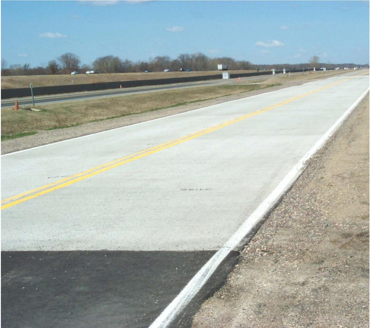
**Figure 3.11: Cell 39 Looking NW Showing Porous Concrete Overlay, Bituminous Transition and French Drain Shouldering Aggregate**
