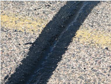
Researchers recommend avoiding sealant overbanding on the sides of cracks.
