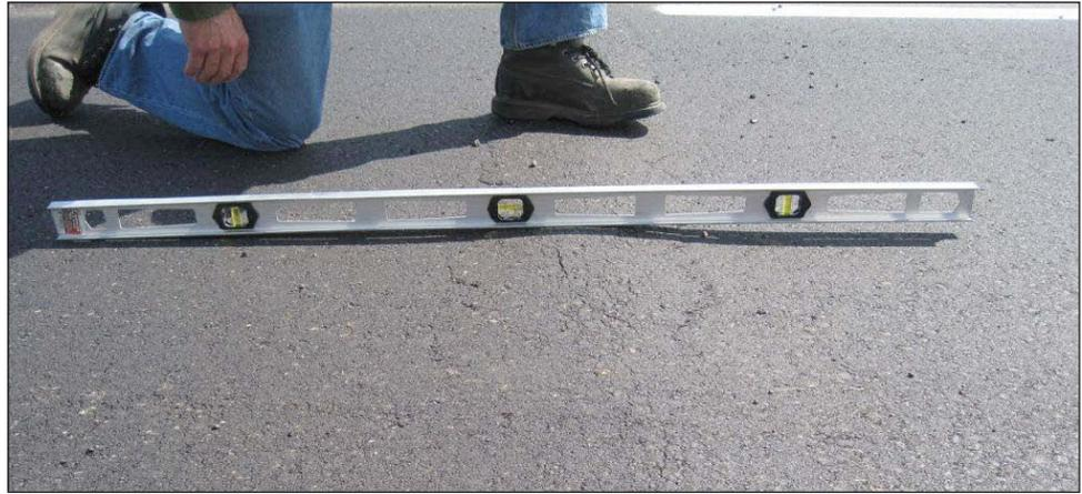
Researchers often found bumps during the first field visit, including this 1/2-inch tall bump with hairline cracking, indicating that compaction equipment had been operated when the HMA temperature was not optimum.
