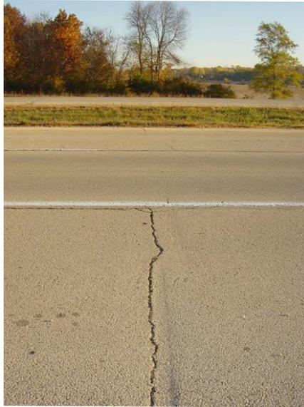
Low-temperatures cause asphalt pavements to contract, which may lead to cracking. Asphalt mixtures and binders that are not as rigid in cold temperatures are better able to relax stresses, making pavements less brittle and prone to fracture.
