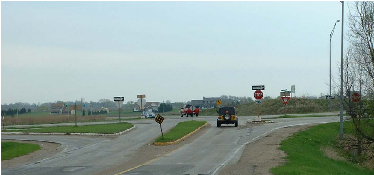
FIGURE 4-13 Southbound Approach of NE 70 th Street. (Note the median on NE 70 th Street and general sign clutter.)
