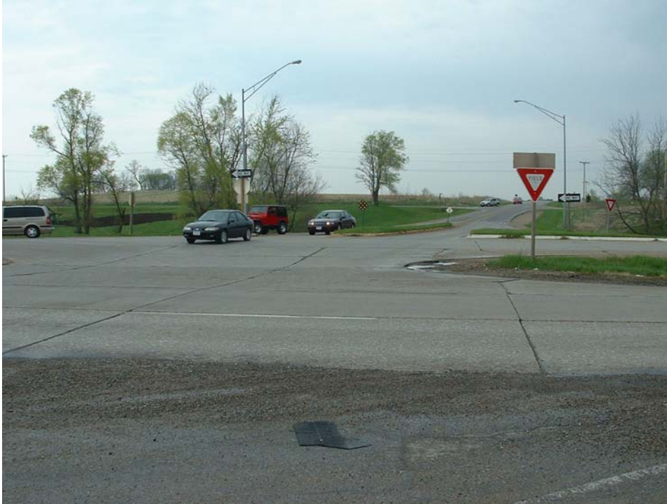
FIGURE 4-12 Looking North at Vehicles Crossing IA 163.
