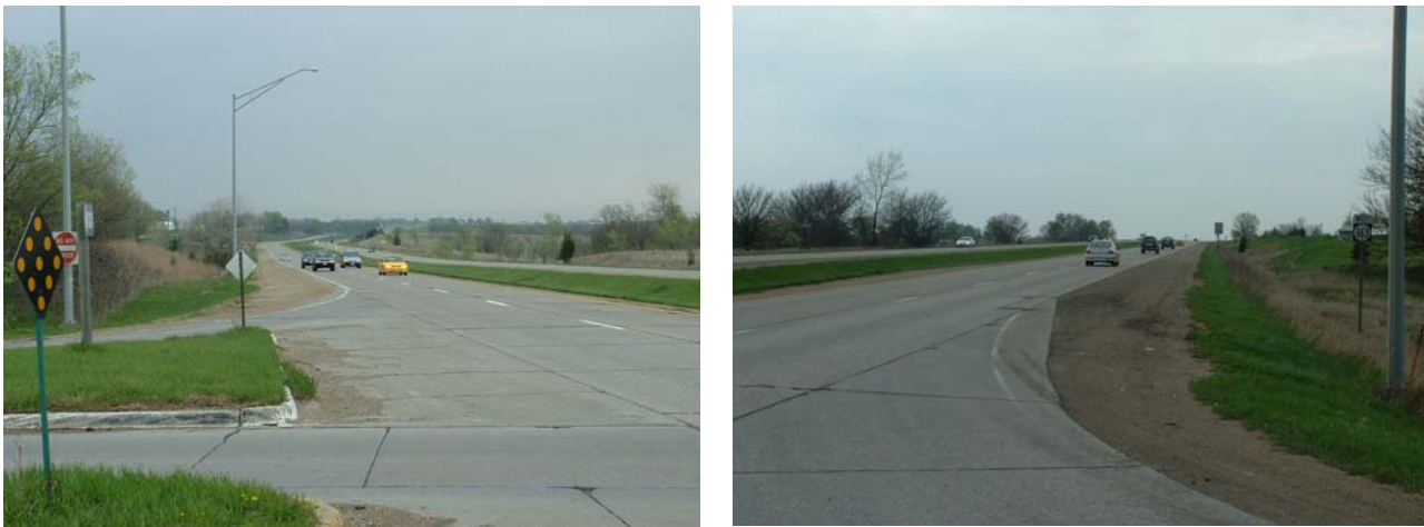
FIGURE 4-11 Looking East (left) and West (right) from North Approach of NE 70 th Street.
