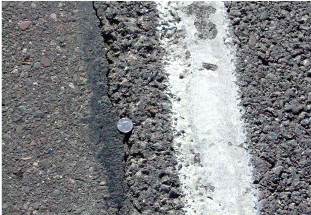
Figure 7: Longitudinal Edge Crack - after 7 years. Photo Taken at RP 184 NB on February 14 th , 2007.
