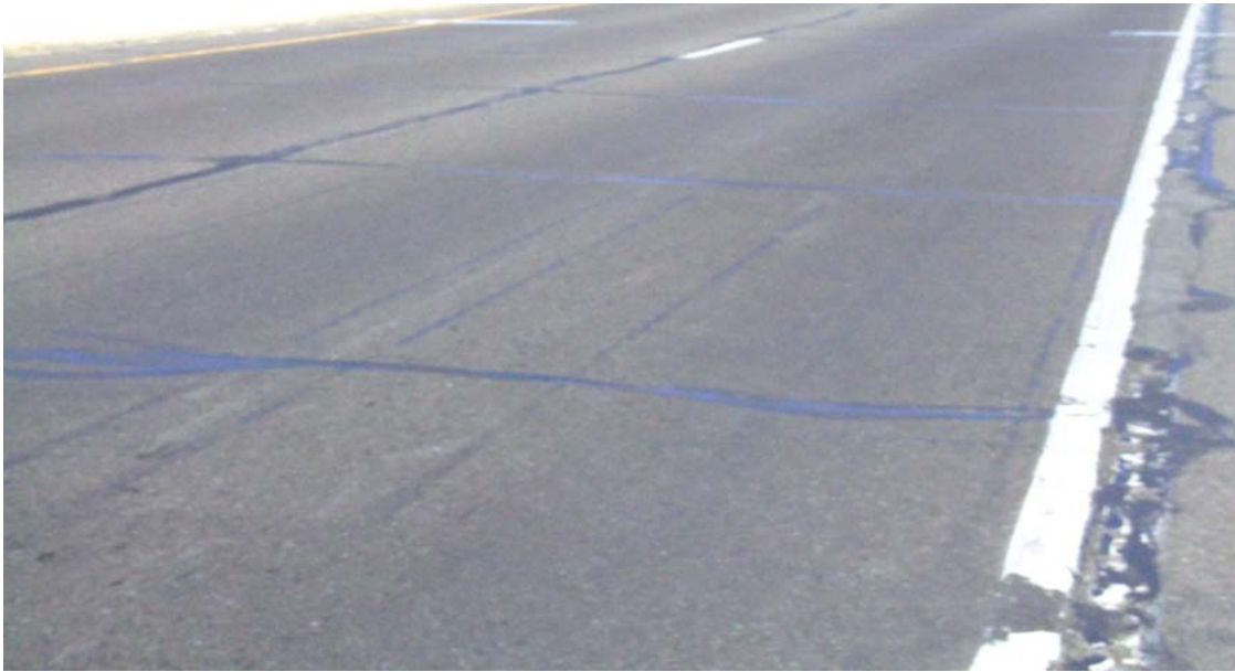
Figure 6: Cracks Sealed Section. Photo taken at RP 185.4 NB on February 14 th , 2007.
