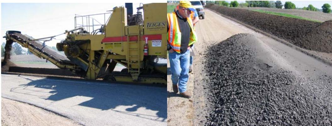
Figure 1.1: Full Depth Reclamation and Recycled Asphalt Pavement (RAP).
