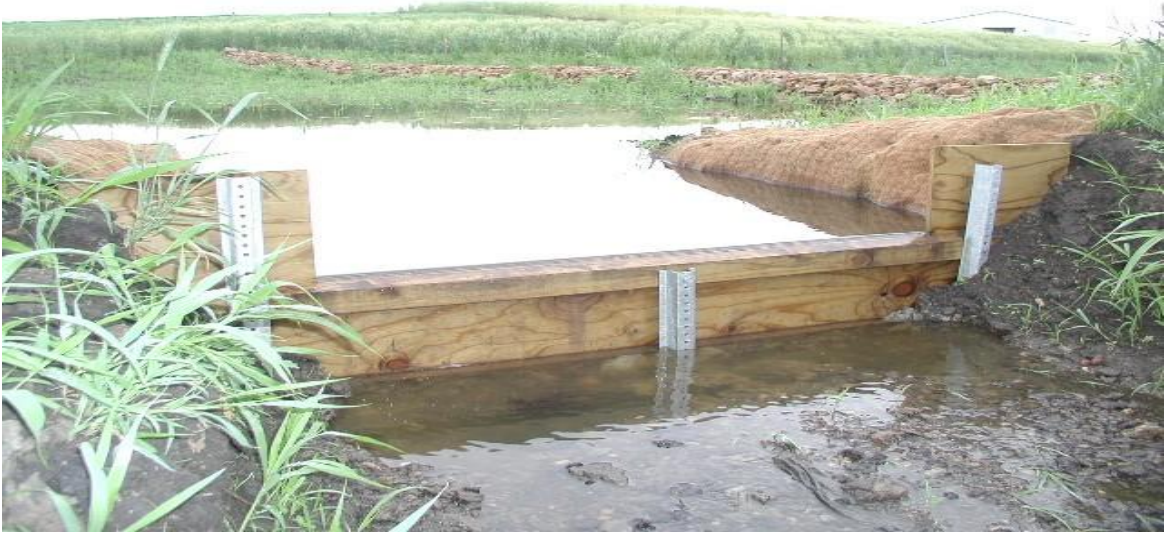
Figure 3.15: Rectangular weir at the inlet of Carver County dry detention pond
