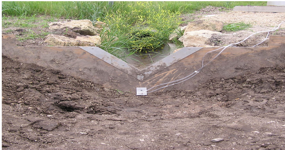
Figure 3.11: Compound weir, bubble line and suction line at the inlet of the Mn/DOT dry detention pond 4012-04
