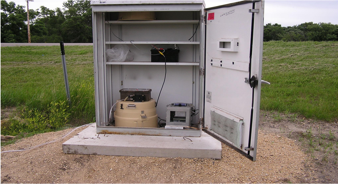
Figure 3.10: Storm water monitoring equipment at the inlet of the Mn/DOT dry detention pond 4012-04
