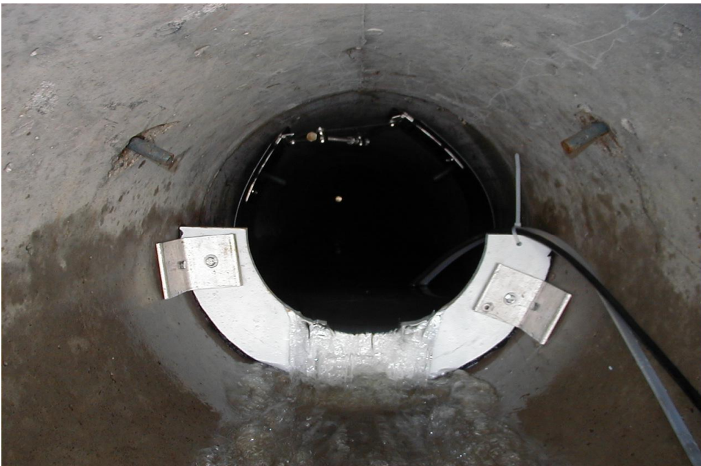
Figure 3.18: 3.5 inch high plastic circular weir at the outlet (culvert) of the Carver County dry detention pond
