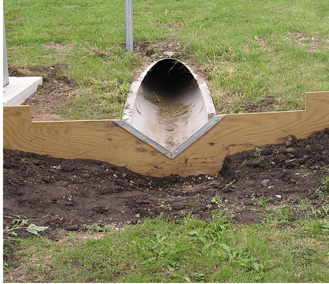
Figure 3.14: Compound weir at the outlet of the Mn/DOT dry detention pond 4012-03
