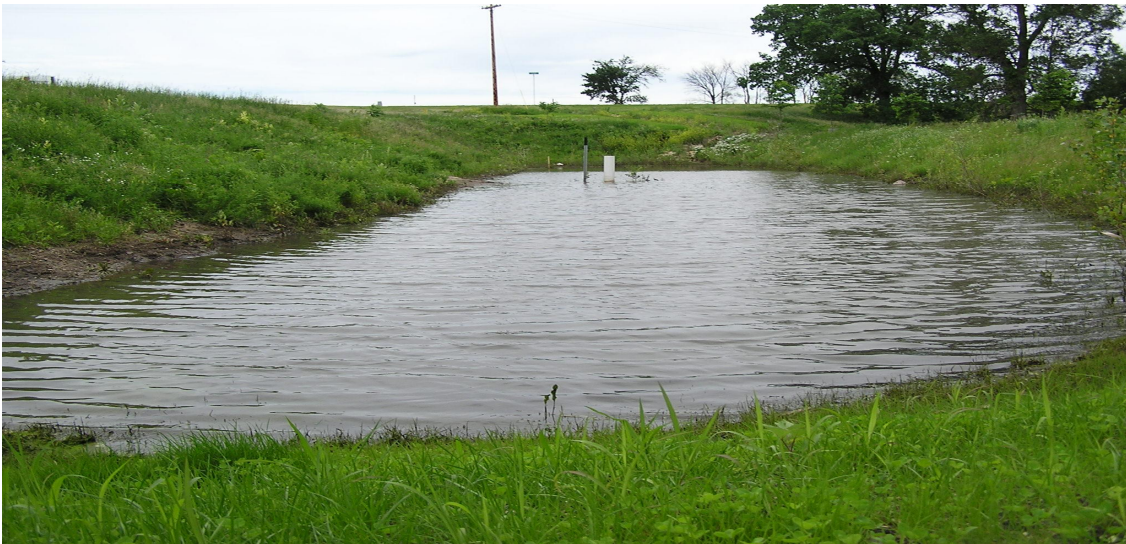
Figure 4.1: Mn/DOT dry detention pond 4012-03 after a few storms in August 2004.
