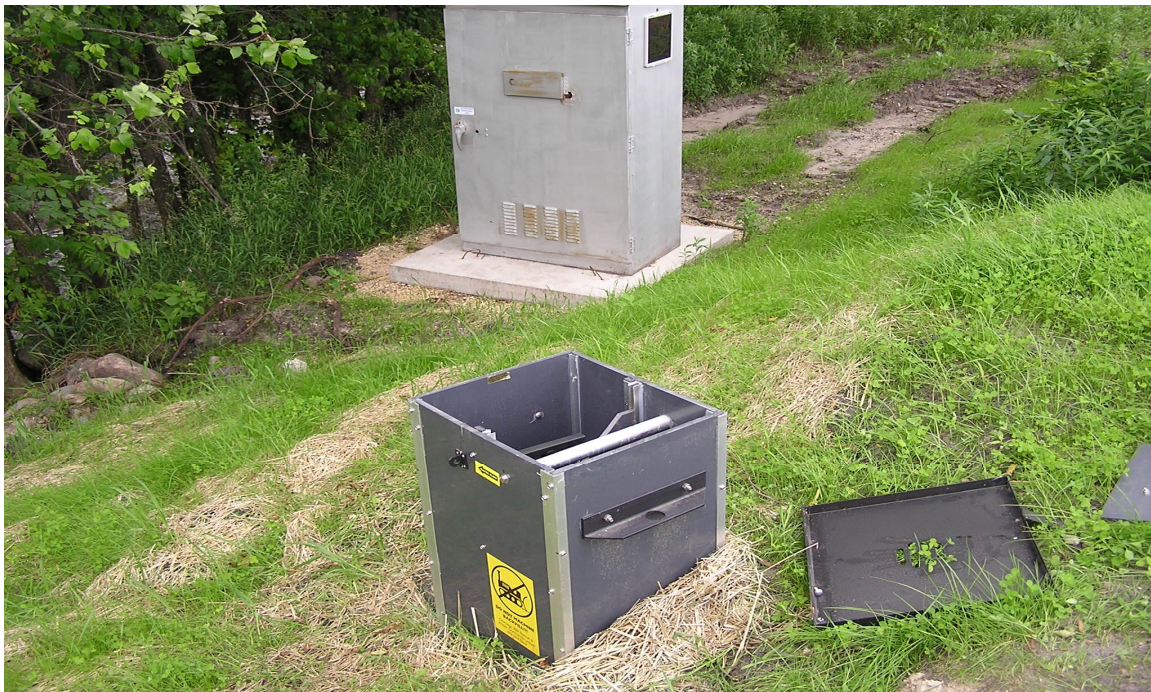
Figure 3.13: AgriDrain® Outlet structure and environmental cabinet at the outlet of the Mn/DOT dry detention pond 4012-03
