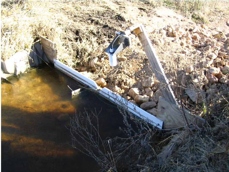
Figure 3.16: Rectangular weir with v-notch insert at the inlet of Carver County dry detention pond
