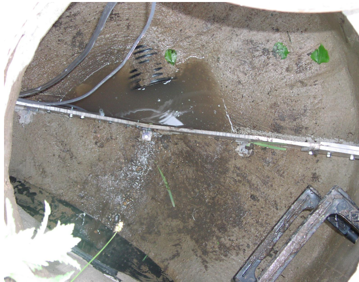
Figure 3.12: Top view of the compound weir, bubble line and suction line at the outlet of the Mn/DOT dry detention pond 4012-04
