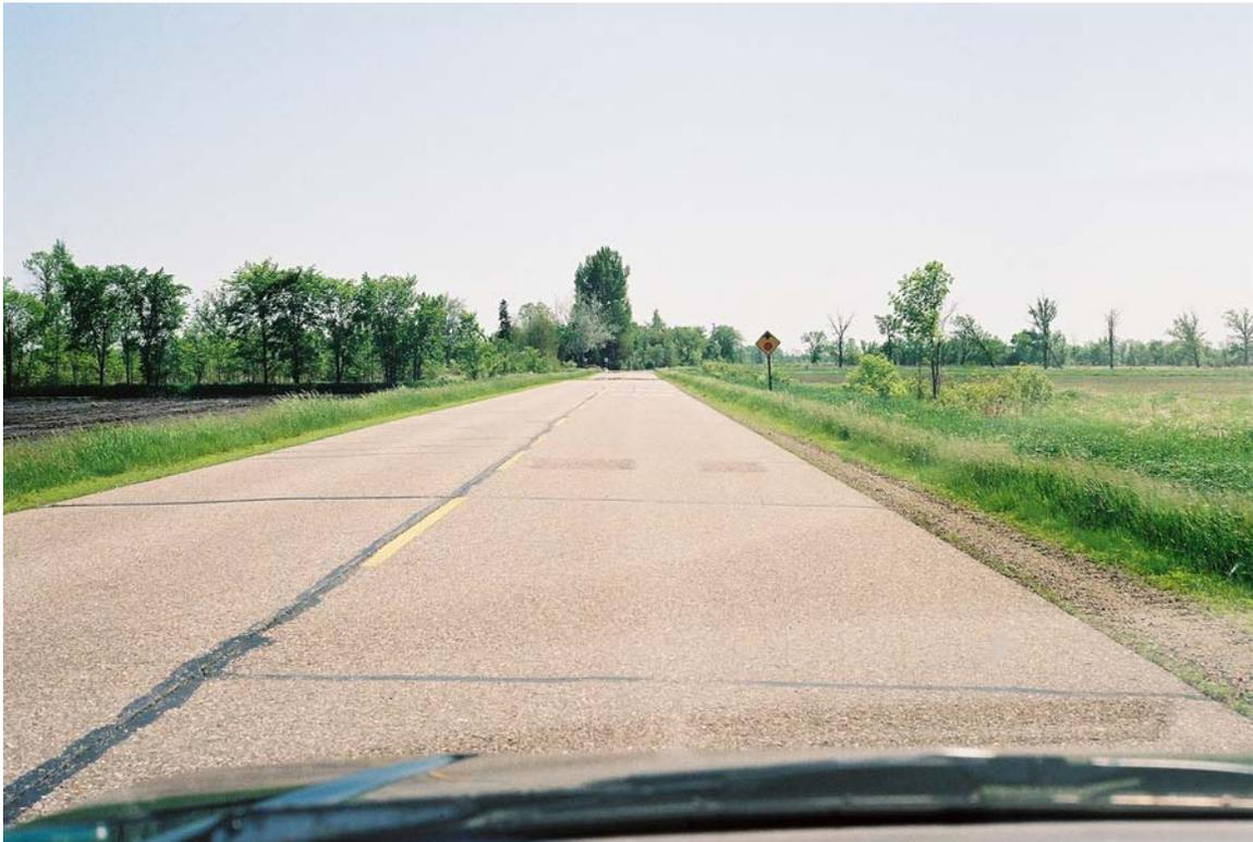
Photograph #251 (Reel #12, 13A) (from North, looking South): first rumble strip and warning sign in view; also, STOP AHEAD on road.
