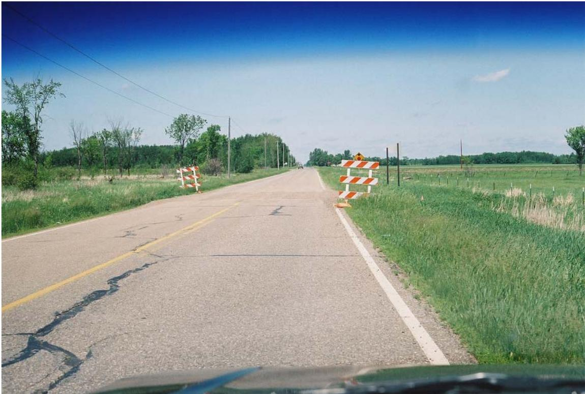
Photograph #224 (Reel #11, 10A) (from South, looking North): first rumble strip difficult to see—it is just before new construction; warning sign in view; STOP AHEAD on road also difficult to see.
