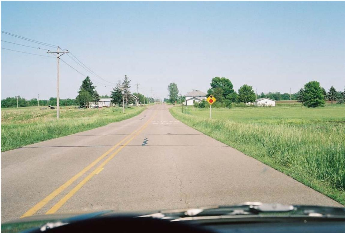
Photograph #272 (Reel #13, 10) (from West, looking East): first rumble strips *missing*; warning sign in view; also, STOPAHEAD on road.
