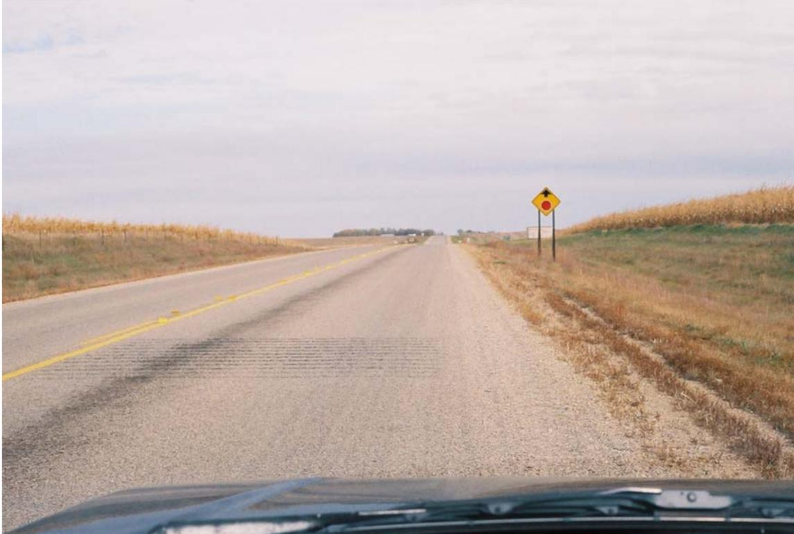
Photograph #97 (Reel #5, 16A) (from South, looking North): first rumble strip and warning sign (with red center unlike warning signs on other three approaches to the four-way stop) in view.
