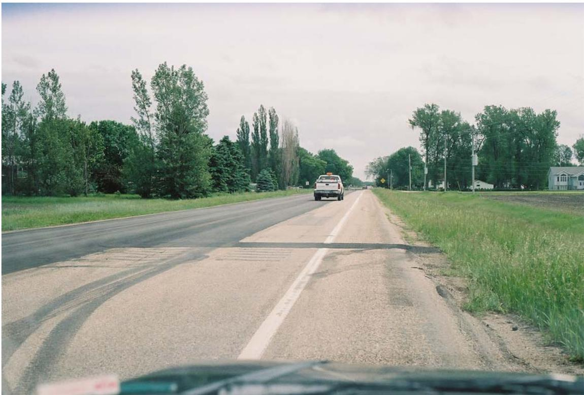
Photograph #371 (Reel #17, 17) (from West looking East): rumble strips on old road surface are filled in, then to the right there is an operational *half rumble* strip on old road surface (new surface does *not* have other half rumble strip to left); warning sign in view [note distance between warning sign and rumble strip greater than usual].
