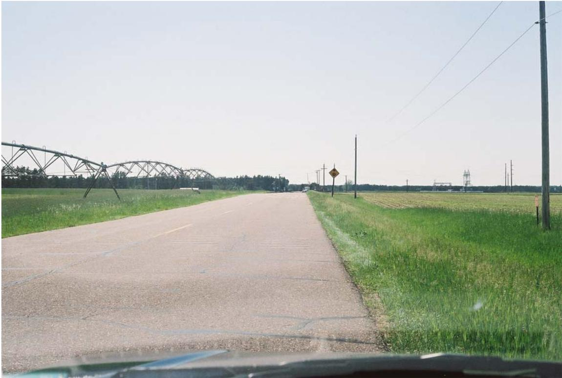
Photograph #261 (Reel #12, 23A) (from East, looking West): first rumble strips *filled in* (note second set—a double set—is in place closer to intersection); warning sign in view; also, STOP AHEAD on road.
