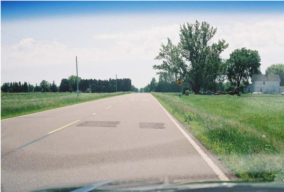
Photograph #228 (Reel #11, 14A) (from North, looking South): first rumble strip and warning sign in view, also STOP AHEAD on road.
