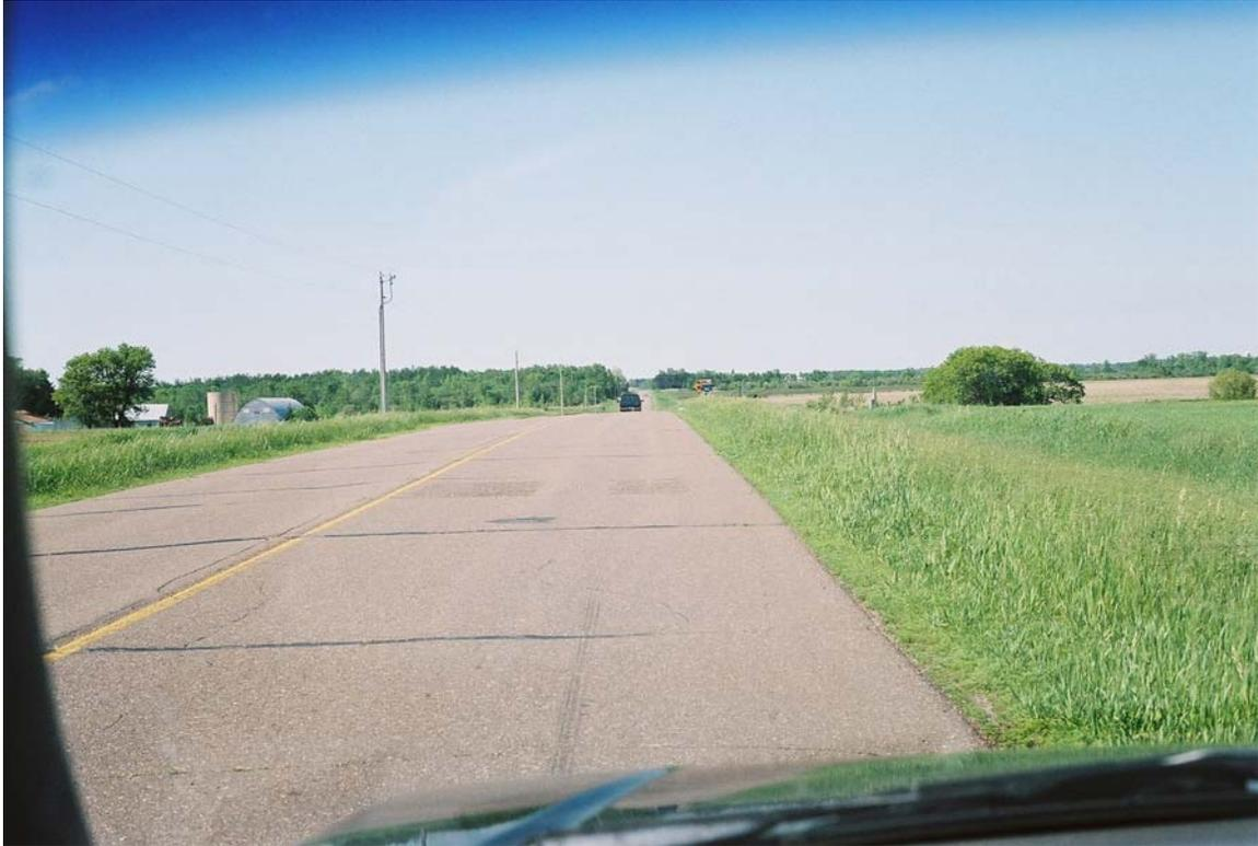
Photograph #268 (Reel #13, 6) (from South, looking North): first rumble strips but *No* warning sign.
