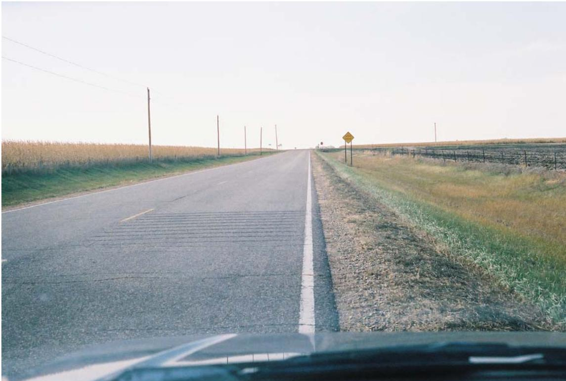
Photograph #145 (Reel #7, 16A) (from East, looking West): first rumble strip and warning sign in view.
