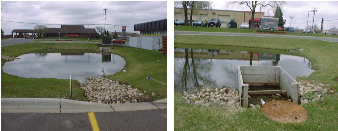
Figure 2. Photograph of Constructed infiltration Basins at the Inter-bank, Roseville
