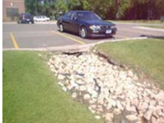
Figure 2: Erosion at USBank. Taken 6/22/05 (Pre-10-day precip. >2")
