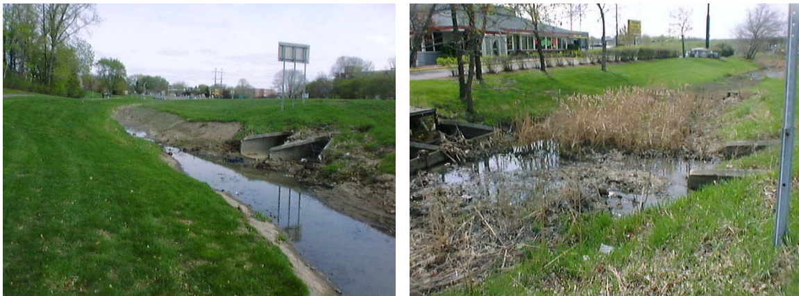
Figure 5. Photograph of Wet Swales on the west and east sides, respectively, of Century Avenue, Maplewood
