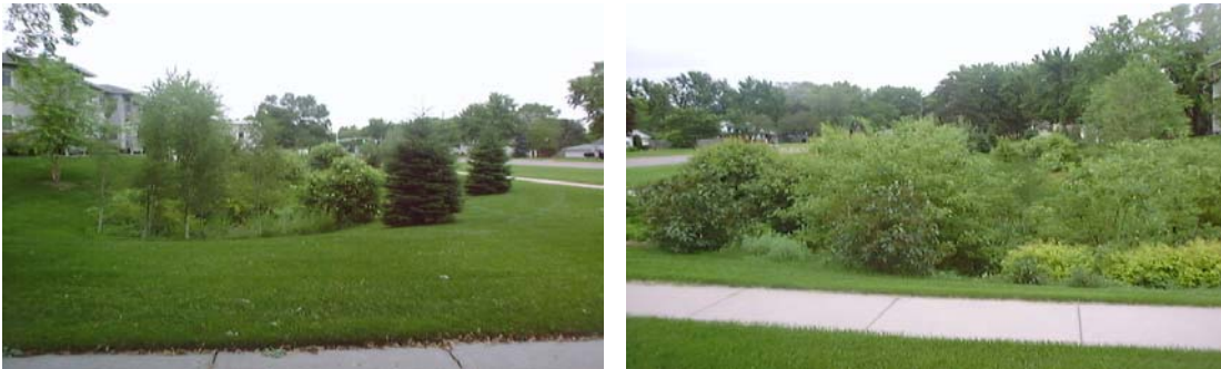
Figure 7. Photograph of Constructed Infiltration Basin at Realife Coop apartment complex in Bloomington
