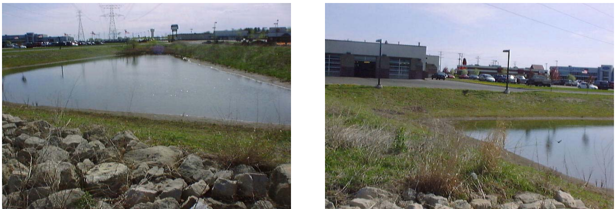
Figure 6. Photograph of Constructed Infiltration Basin at the Pony Express Car Wash in Oak Park Heights
