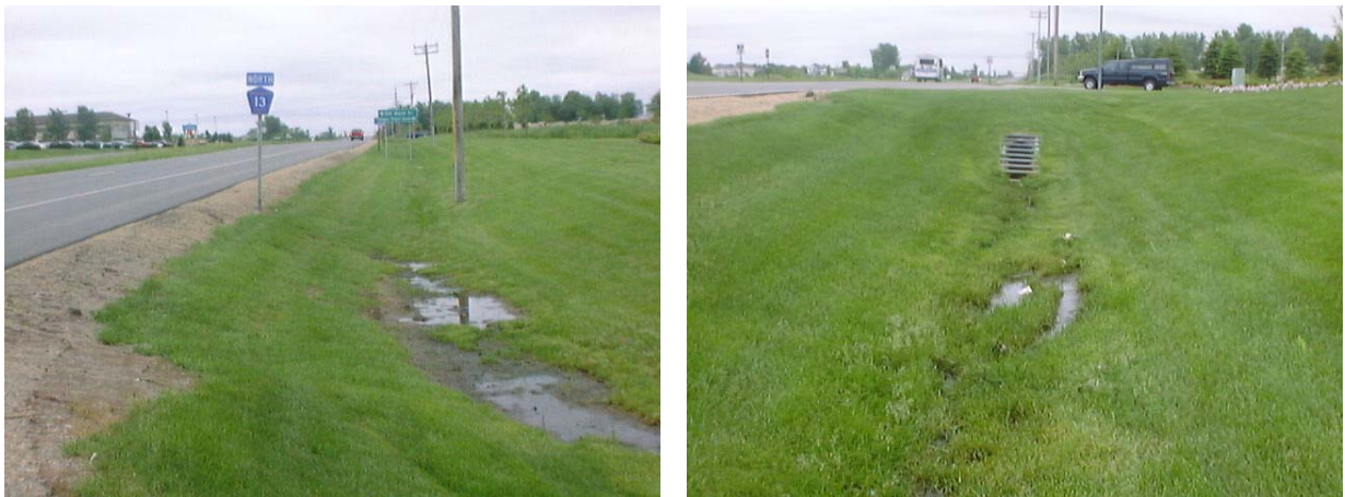
Figure 9. Photograph of Grassed Swale with check dams at Bremer Bank, CR 13
