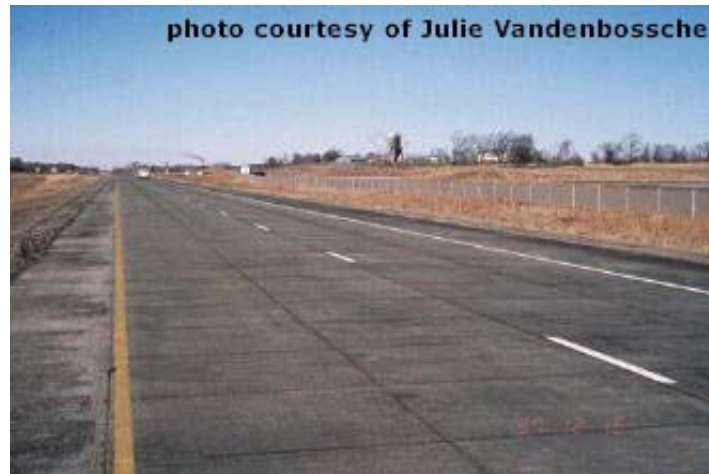
Figure 5.3 Newly Constructed Sections on I-94
