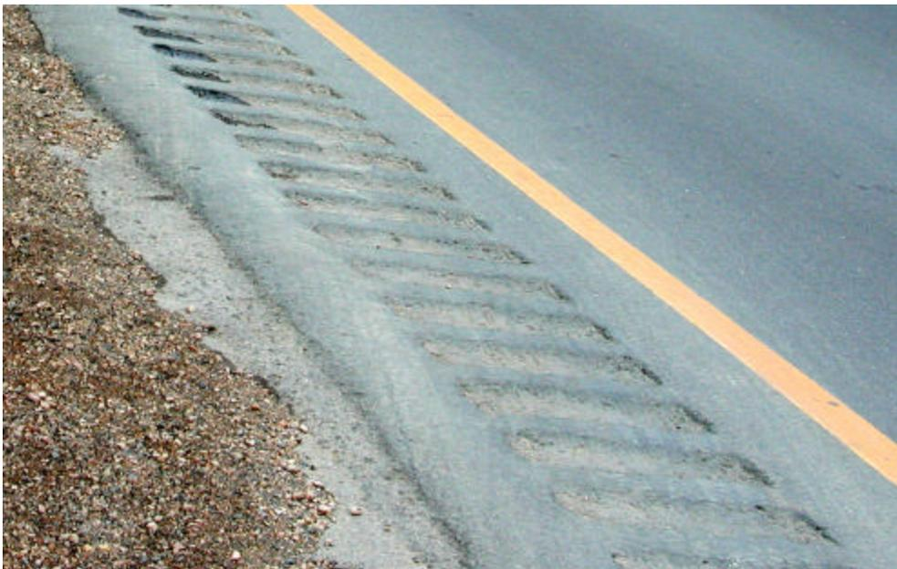
Figure 1-4: Longitudinal rumble strips, clustered
