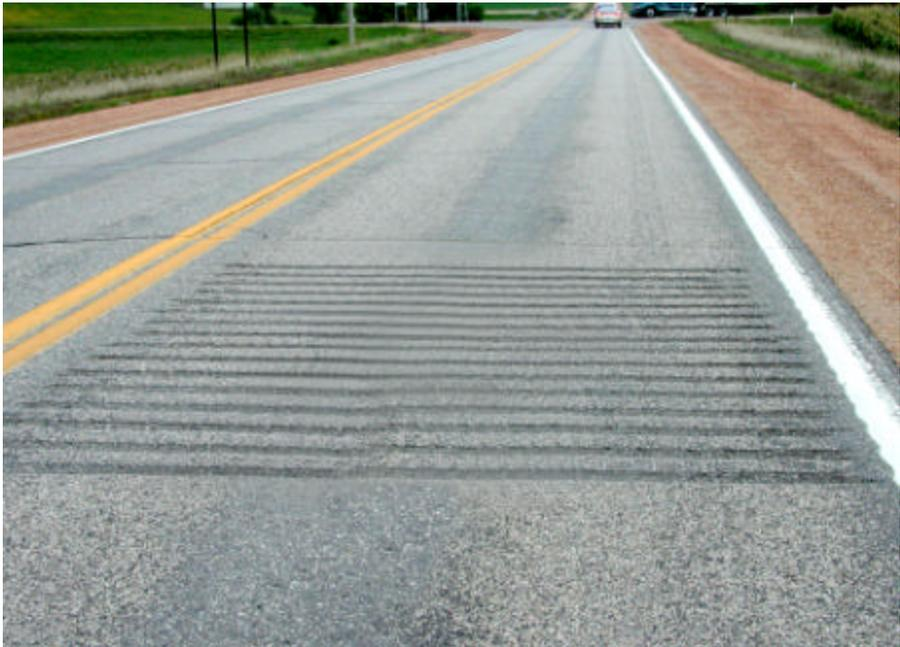
Figure 1-2: In-lane rumble strips, wheelpath
