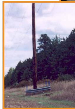
Examples of Guardrail Creating a Greater Hazard than the Object
