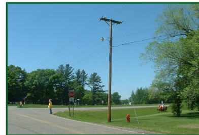
Example of Using Luminaire Mast Arm on Existing Utility Pole Source: MnDOT Traffic Engineering Manual.
