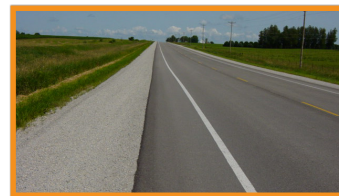
Example of Re-graded Roadside and the Use of Grates on Culverts
