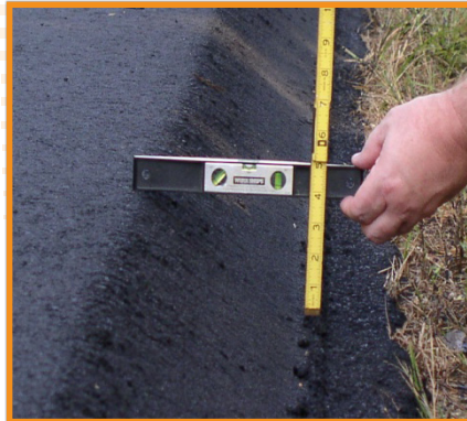
With Safety Edge
