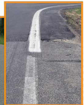
Example of Embedded Wet Reflective Marking
